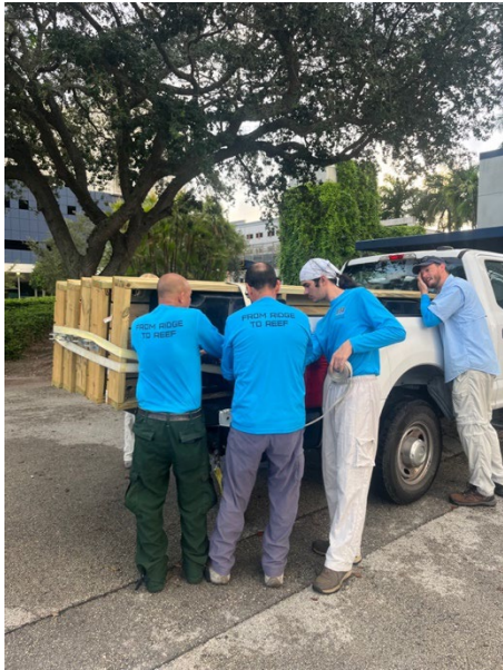
Figure 4: Floating docks and steel pilings being loaded into transport trucks at Florida International University for delivery to Big Cypress National Preserve (BICY) as part of flume construction efforts.
