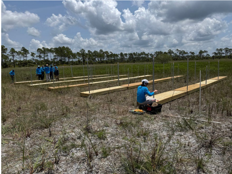
Fig. 6: Floating docks positioned within steel pilings at the flume installation site C. These docks will form the channel walls of the experimental flumes and are secured in place to withstand hydrologic conditions within the marsh.
