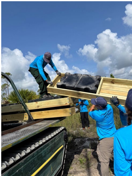
Fig. 5: Loading floating docks from transport trucks into a Marsh Master for delivery to flume construction sites within the marsh. Each dock weighs approximately 230 pounds, requiring coordinated effort during transfer and deployment.
