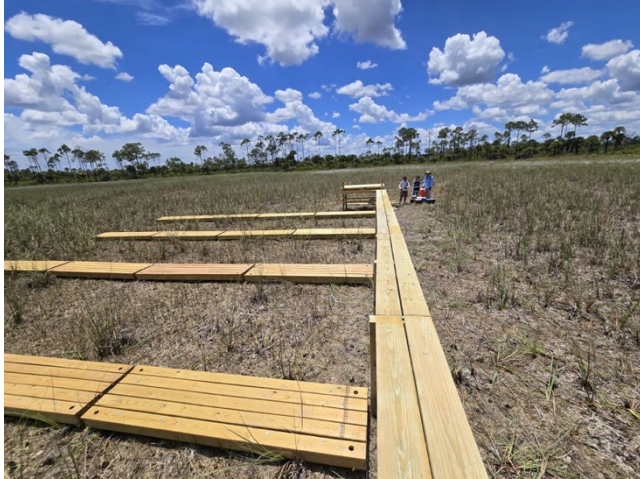
Fig. 7: Front wooden boardwalk and command center alongside installed floating docks at Site B. The boardwalk provides access to the flumes, while the command center will house electronics and phosphorus dosing equipment.
