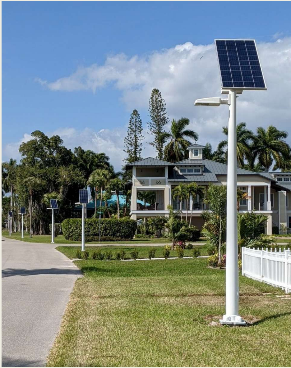
New LED Solar Lamp posts replaced the historic lamp fixtures
