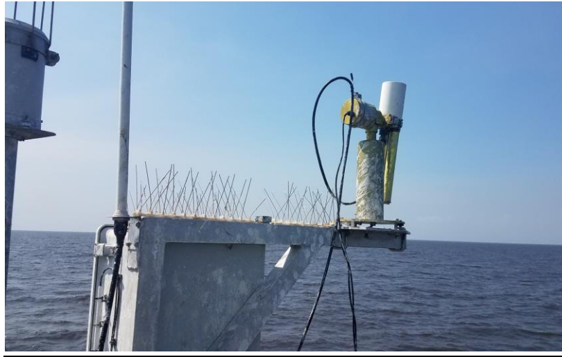
Figure 5A-2: SeaPRISM maintenance site visit on 3/18/21. Bird spikes and cables visible, along with guano covering the vertical piece of the robotic mount.
