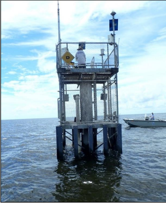
Figure 6-1: Pre-installation view (north side) of instrument tower L001.
