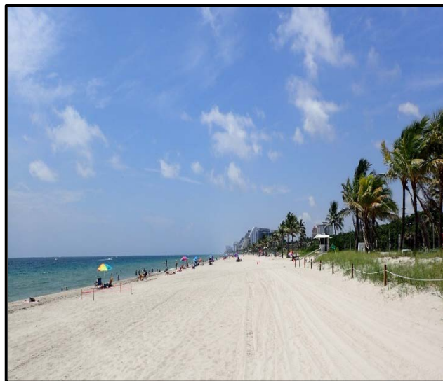
Broward County Shore Protection Project – Segment II, August 2018
