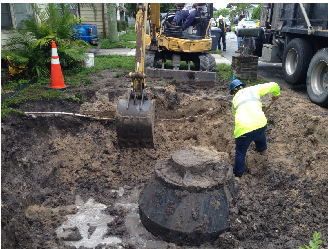
Figure 4: Installation of Gravity Sewer in Lakeland
