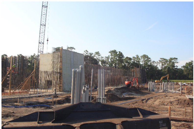
New St. Johns County Wastewater Treatment Plant
