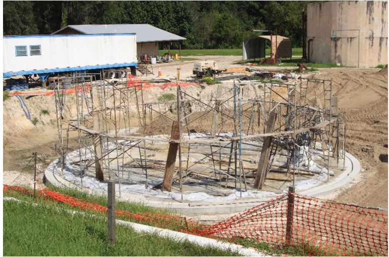
Construction starting on Perry's new clarifier
