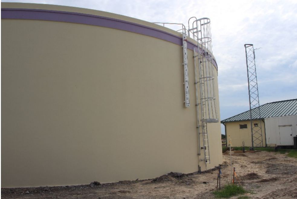
New Reclaimed Water Tank for Deltona
