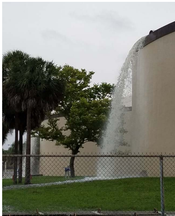
FIGURE 3-1 NWWRF HOLDING TANK OVERFLOWING TO GRADE
