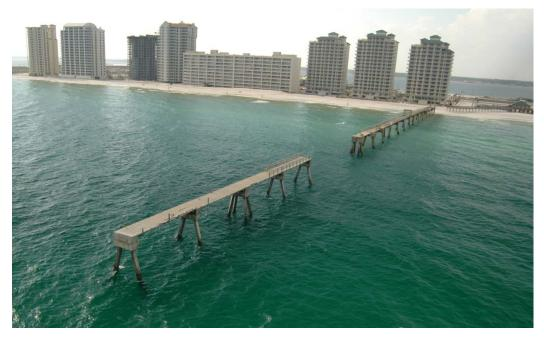
**Photo 31.** Hurricane Dennis destroyed three sections of the solid concrete Navarre Beach Fishing Pier at the seaward end, a mid-section, and at the shoreline [BBCS Files]
