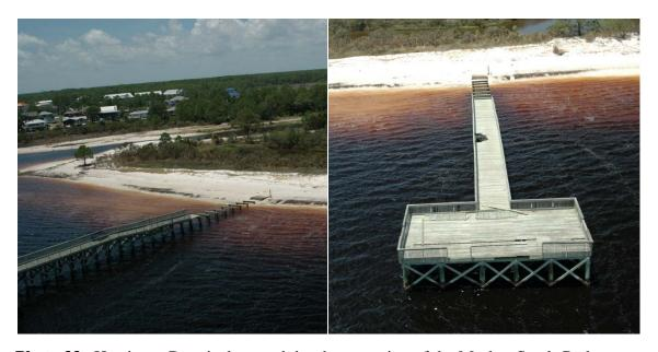
**Photo 33.** Hurricane Dennis damaged the shore-section of the Mashes Sands Park Fishing Pier [BBCS Photo Files]
