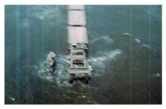
**Photo 6.** Okaloosa Island Pier's terminal end destroyed by Hurricane Frederic (1979)
