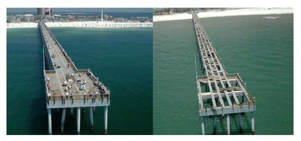
**Photo 30.** Before and after aerial views of the Pensacola Beach Fishing Pier showing that Hurricane Dennis' wave uplift forces removed deck panels without major structural damage [BBCS Photo Files]
