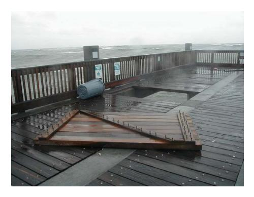
**Photo 21.** Tropical Storm Isidore's wave uplift forces dislodged deck panels on Pensacola Beach Pier (2002)
