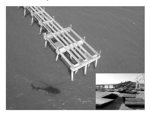
**Photo 28.** Wave uplift forces from Hurricane Ivan dislodged deck panels from the Pensacola Beach Fishing Pier [Photo courtesy of Olsen Associates, Inc.]
