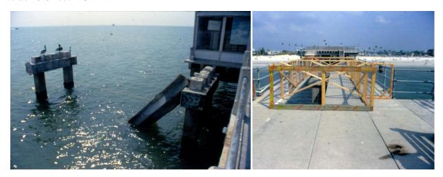
Photo 10. Elena caused isolated major wave damage to Big Pier 60, Clearwater Beach
