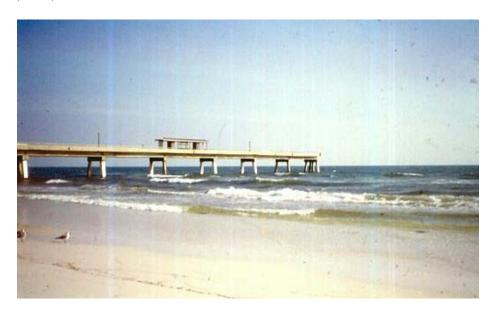
Photo 15. Seaward end of the Okaloosa County Pier destroyed by Opal (1995)
