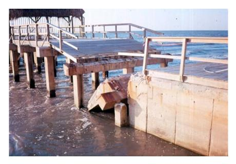
**Photo 18.** Northern Sand Key pier damaged by Tropical Storm Josephine (1996)
