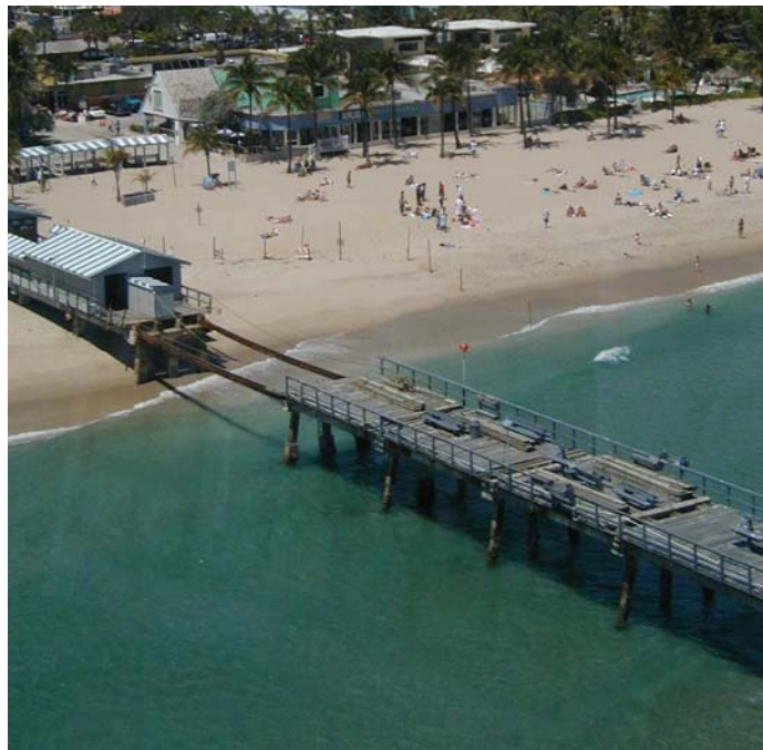
Photo 27. Hurricane Frances destroyed the shore section of the Anglin's Pier, Lauderdale-by-the-Sea [BBCS Photo Files]
