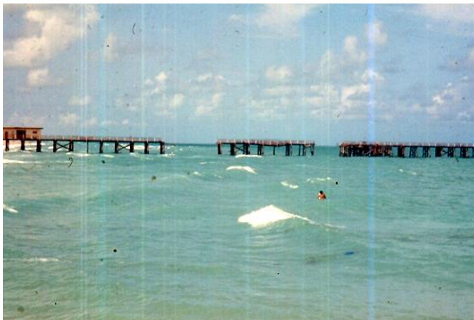
Photo 13. Haulover Beach Pier damaged by Hurricane Andrew (1992)
