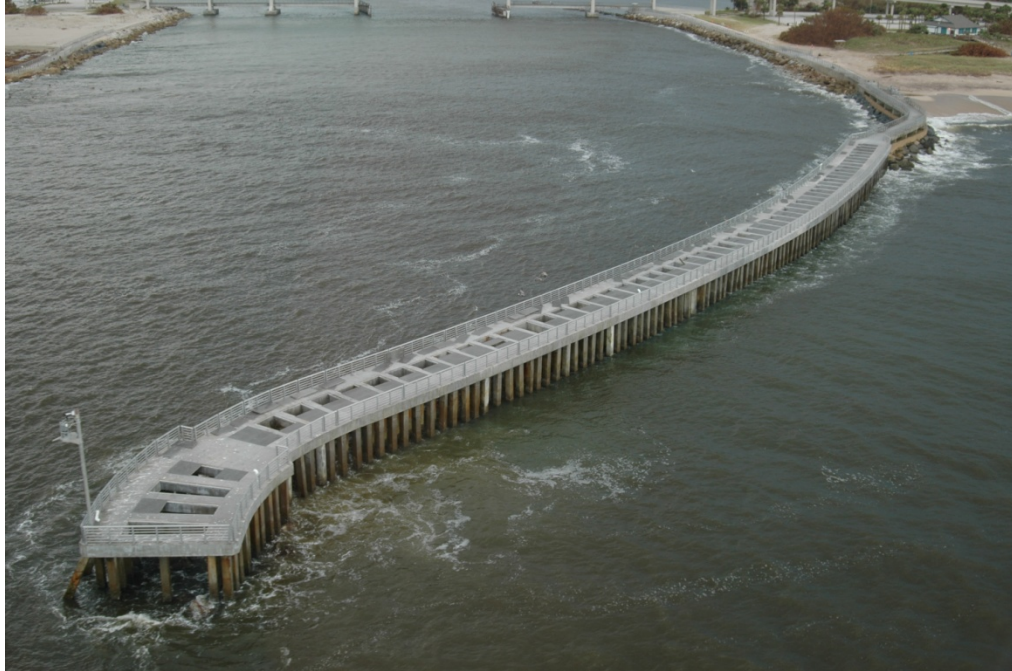
Photo 24. Sebastian Inlet State Park Fishing Pier lost 40-50 breakaway deck grates to Hurricane Frances [BBCS Photo Files]
