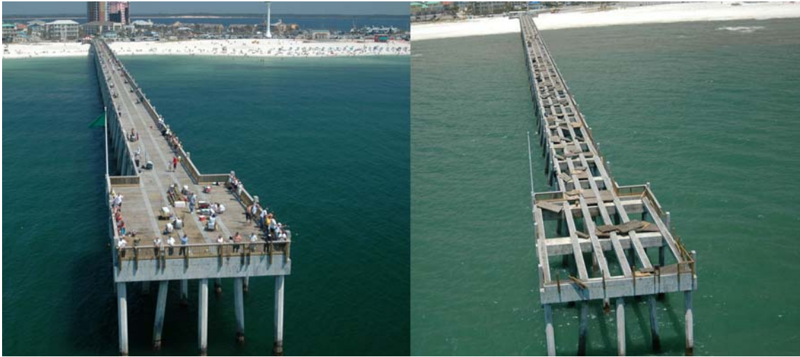
Photo 30. Before and after aerial views of the Pensacola Beach Fishing Pier showing that Hurricane Dennis' wave uplift forces removed deck panels without major structural damage [BBCS Photo Files]
