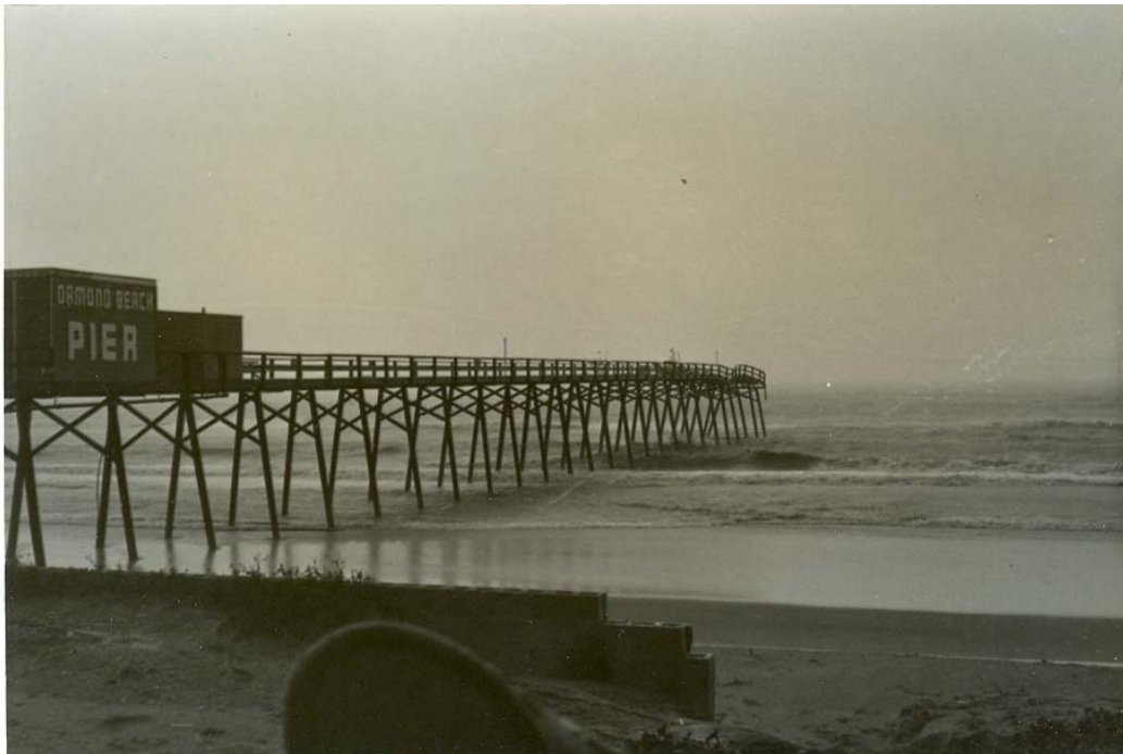
Photo 4. Hurricane Dora destroyed the end of the Ormond Beach Pier (1964) [Photo by W.T. Carlton]
