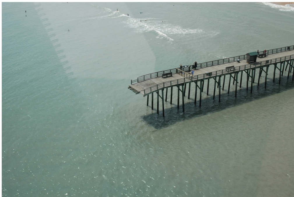
Photo 23. Hurricane Frances destroyed end of Flagler Beach Fishing Pier [BBCS Photo Files]
