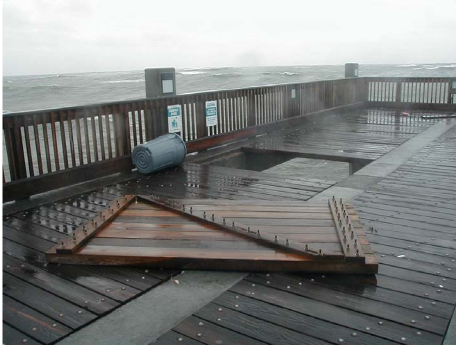
Photo 21. Tropical Storm Isidore's wave uplift forces dislodged deck panels on Pensacola Beach Pier (2002)
