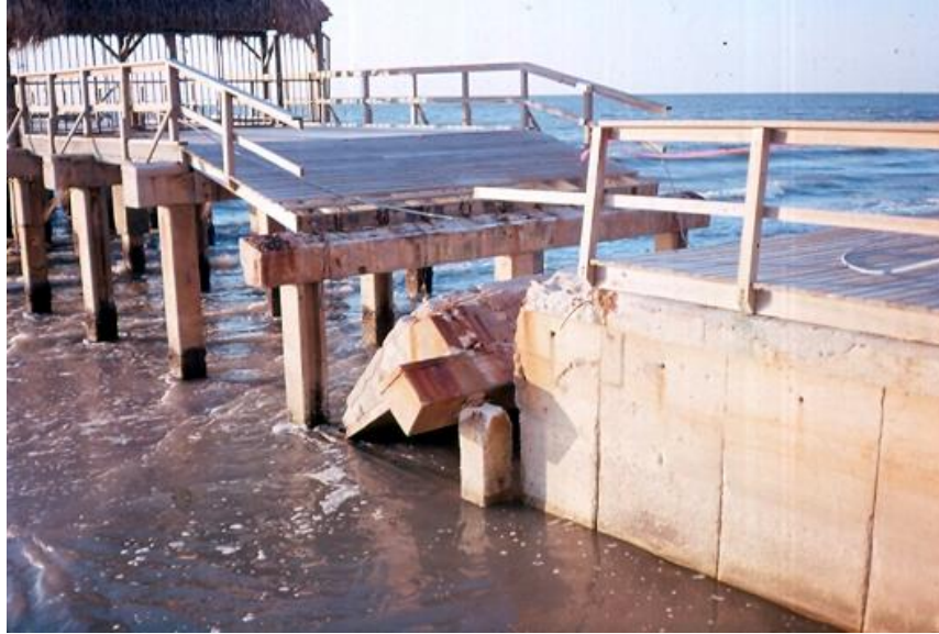
Photo 18. Northern Sand Key pier damaged by Tropical Storm Josephine (1996)
