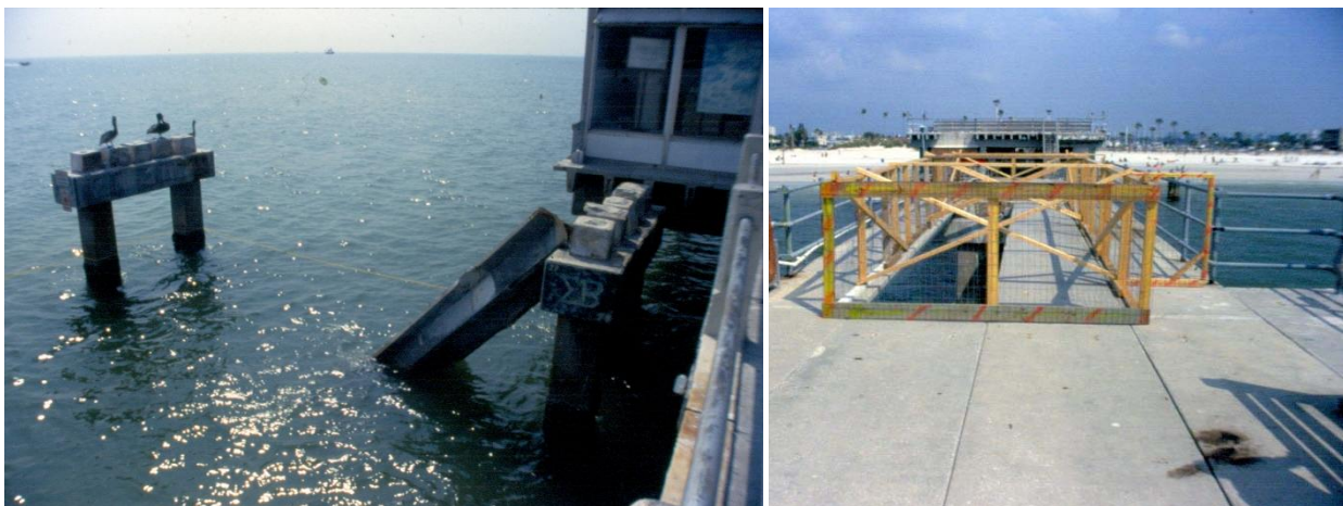
Photo 10. Elena caused isolated major wave damage to Big Pier 60, Clearwater Beach
