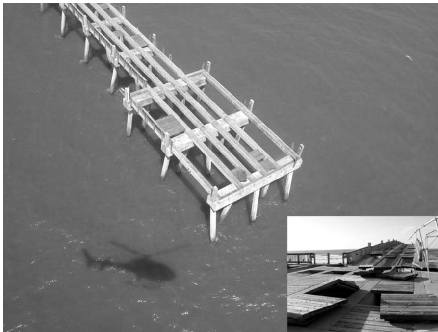
Photo 28. Wave uplift forces from Hurricane Ivan dislodged deck panels from the Pensacola Beach Fishing Pier [Photo courtesy of Olsen Associates, Inc.]
