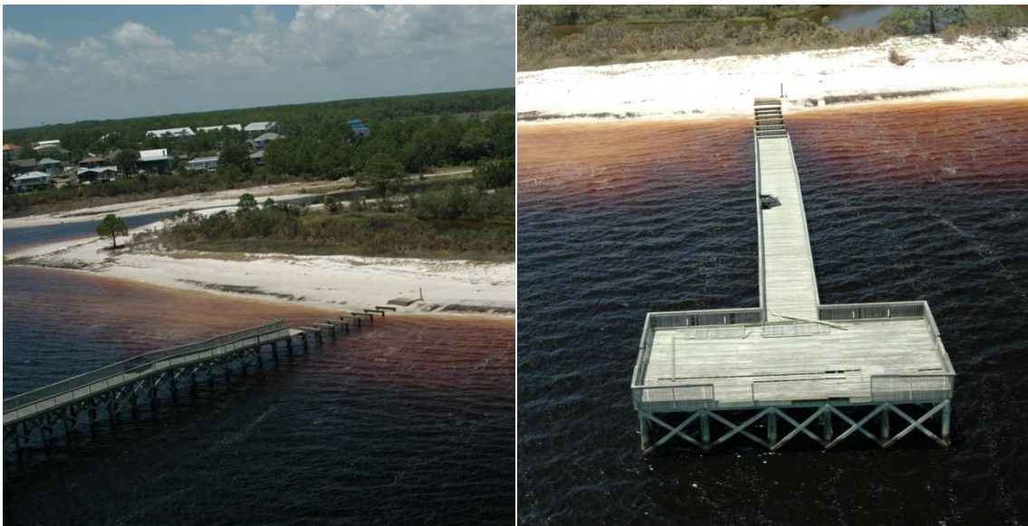
Photo 33. Hurricane Dennis damaged the shore-section of the Mashes Sands Park Fishing Pier [BBCS Photo Files]
