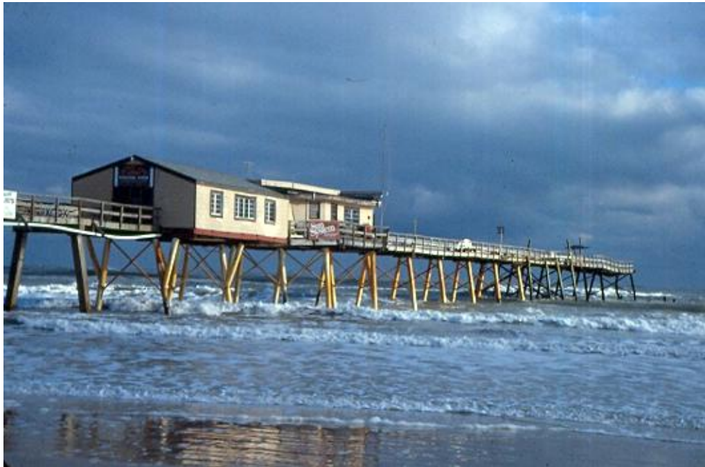
Photo 8. Sunglow Fishing Pier lost its seaward end during Thanksgiving Storm, 1984
