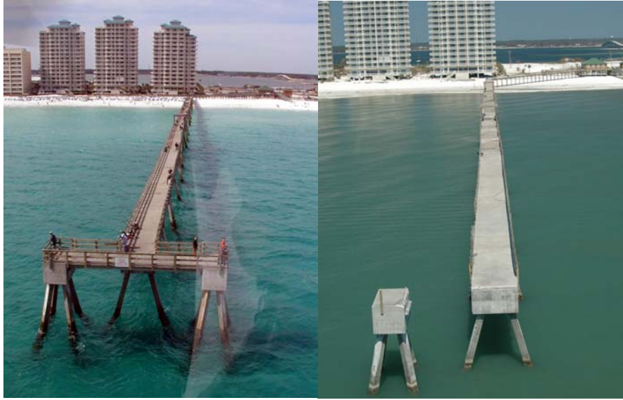
Photo 29. Before and after (April and September 2004) aerial views of the solid concrete Navarre Beach Fishing Pier showing damage from Hurricane Ivan [BBCS Photo Files]
