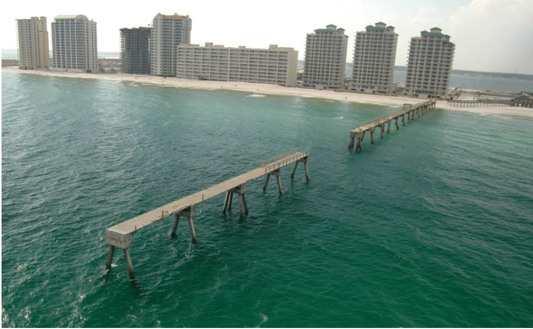
Photo 31. Hurricane Dennis destroyed three sections of the solid concrete Navarre Beach Fishing Pier at the seaward end, a mid-section, and at the shoreline [BBCS Files]
