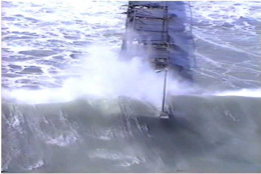
Photo 11. Wave impact loads on the Lake Worth Pier during the Halloween Northeaster (1991) [BBCS Photo Files]
