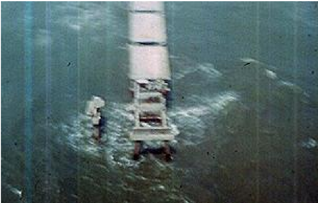
Photo 6. Okaloosa Island Pier's terminal end destroyed by Hurricane Frederic (1979)
