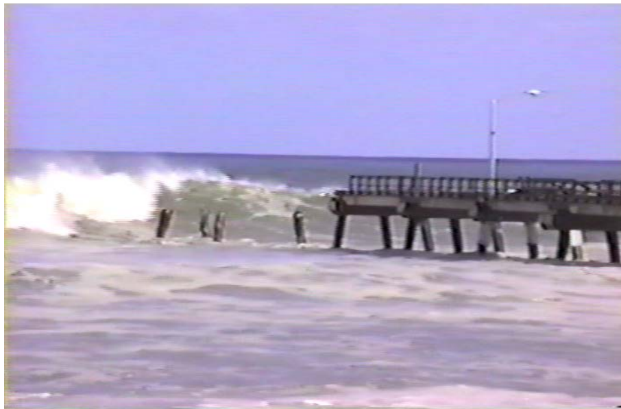
Photo 12. Lake Worth Pier damage from the Halloween Northeaster (1991) [BBCS Photo Files]
