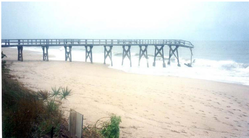
Photo 20. Hurricane Floyd destroyed 400 feet of the Sea Quay Pier, Vero Beach
