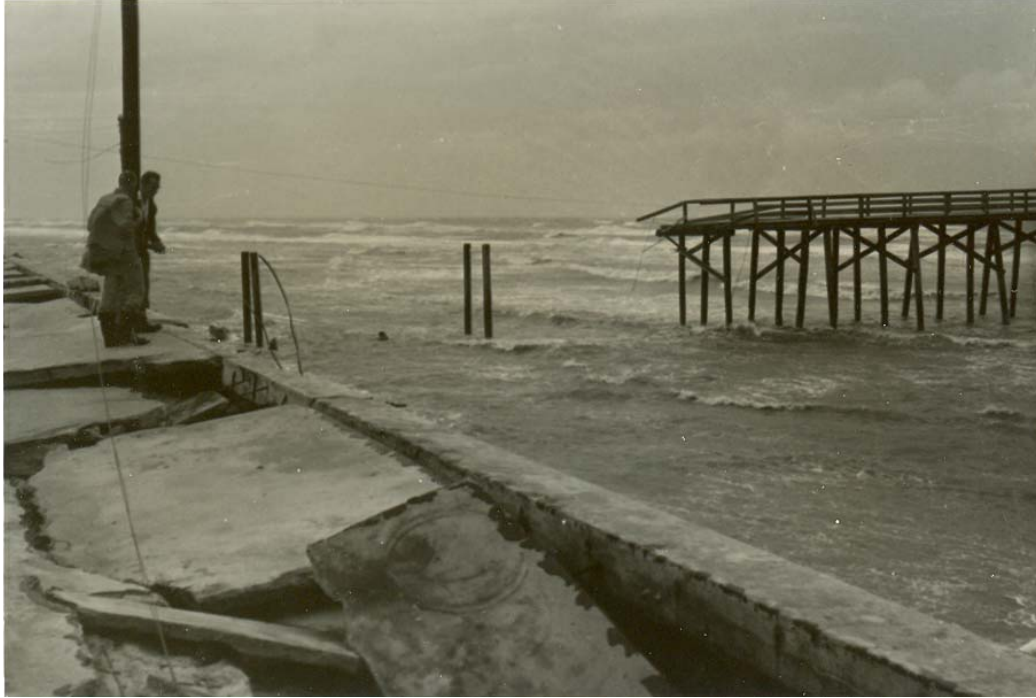
Photo 3. Damage to Jacksonville Beach Pier from Hurricane Dora (1964) [Photo by W.T. Carlton]
