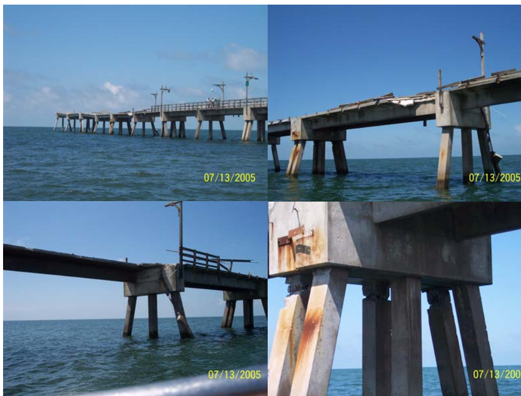
Photo 32. Hurricane Dennis removed an additional 50 feet off the end of the Dan Russell Pier at Panama City Beach and inflicted major damage to another 250 feet [Photos provided by Al Shortt, P.E., City Engineer, Panama City Beach]
