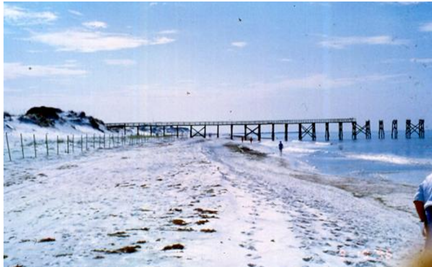
Photo 17. Opal (1995) destroyed 135 feet of St. Andrews State Park Pier
