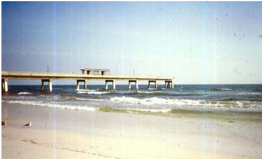
Photo 15. Seaward end of the Okaloosa County Pier destroyed by Opal (1995)
