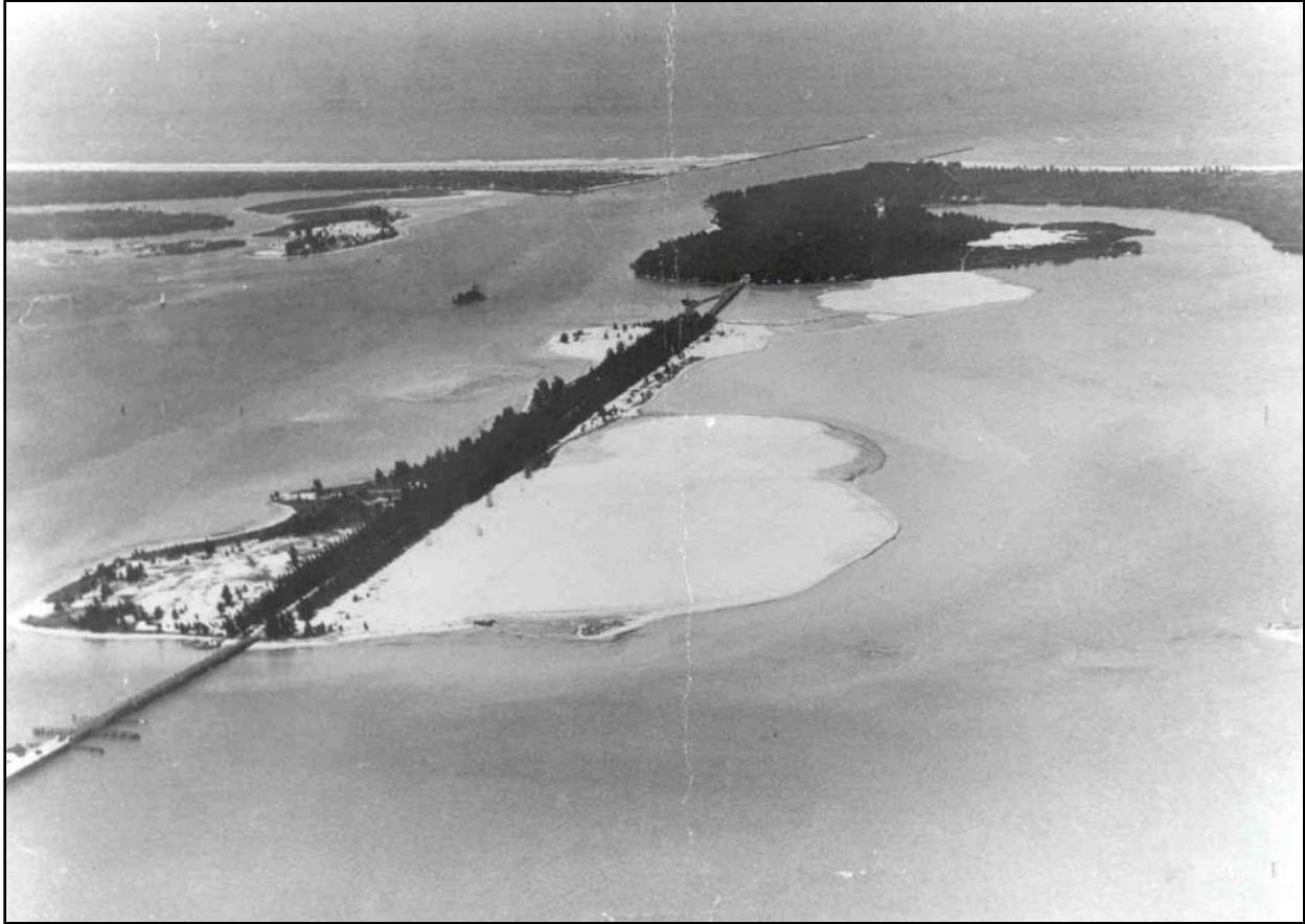
Figure 2. 1926 aerial photograph of the Ft. Pierce causeway, channel and inlet with newly constructed jetties (courtesy of Ft. Pierce Inlet District, St. Lucie County).
