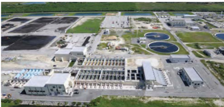
The Clean Water State Revolving Fund provided loans for the Miami-Dade South District Wastewater Treatment Plant.
