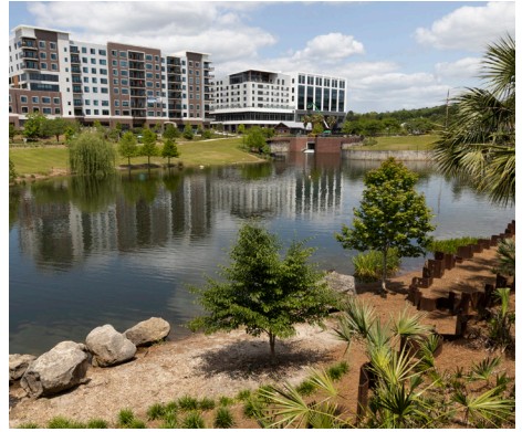
Stormwater pond at Capital Cascades Park.
