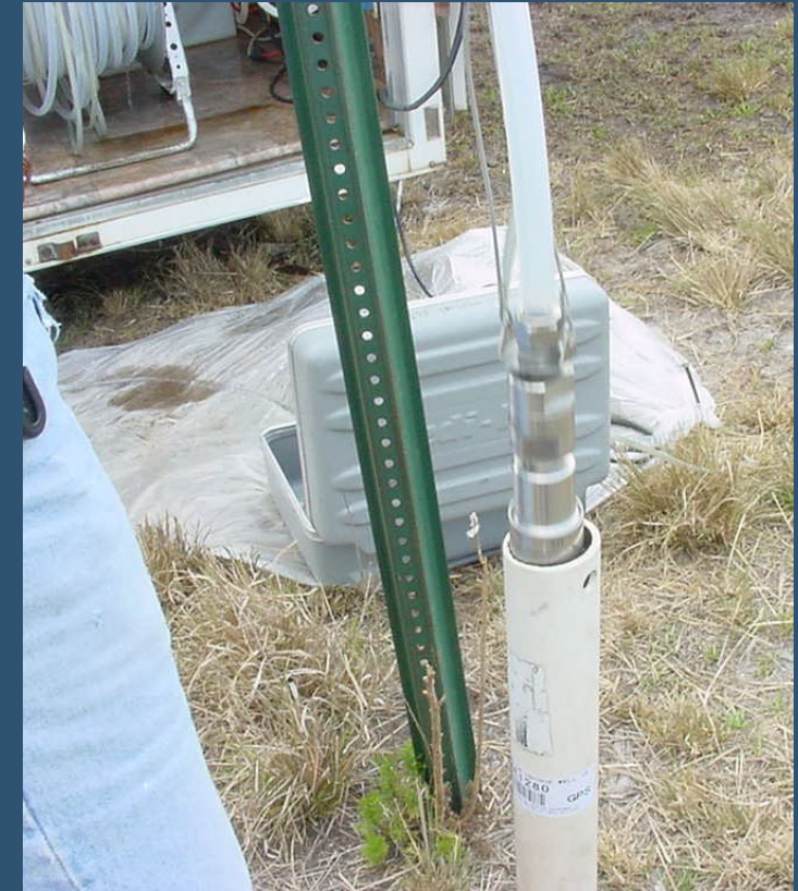
Submersible pump lowering into well.
