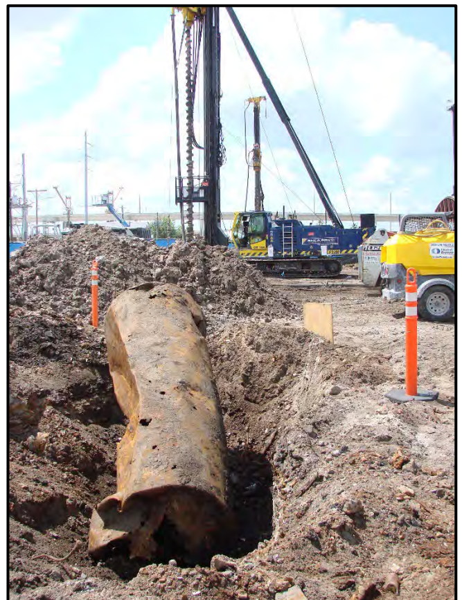
Foundation drilling and soil fill placement. Abandoned tank to be investigated.
