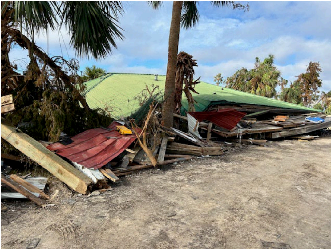
Figure 23. Cedar Island dwelling destroyed.
