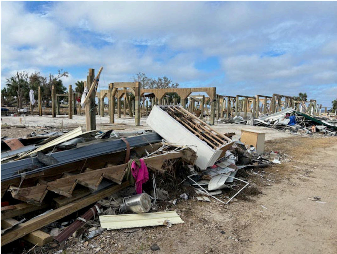
Figure 21. Catastrophic damage on Cedar Island.
