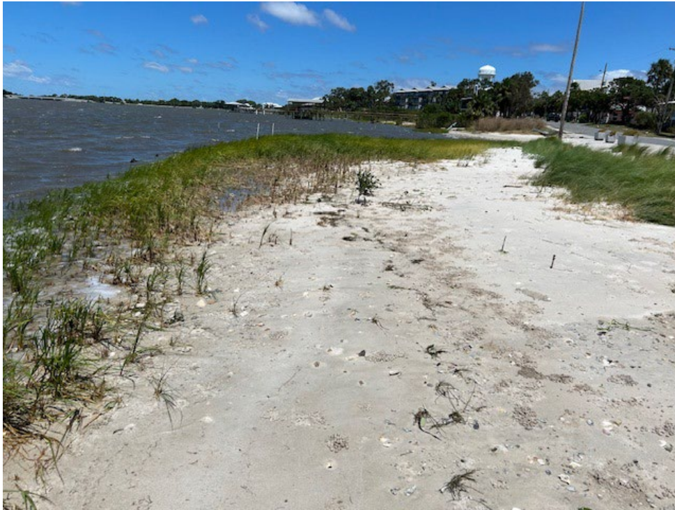
Figure 55. Living shoreline project at G Street after Debby.
