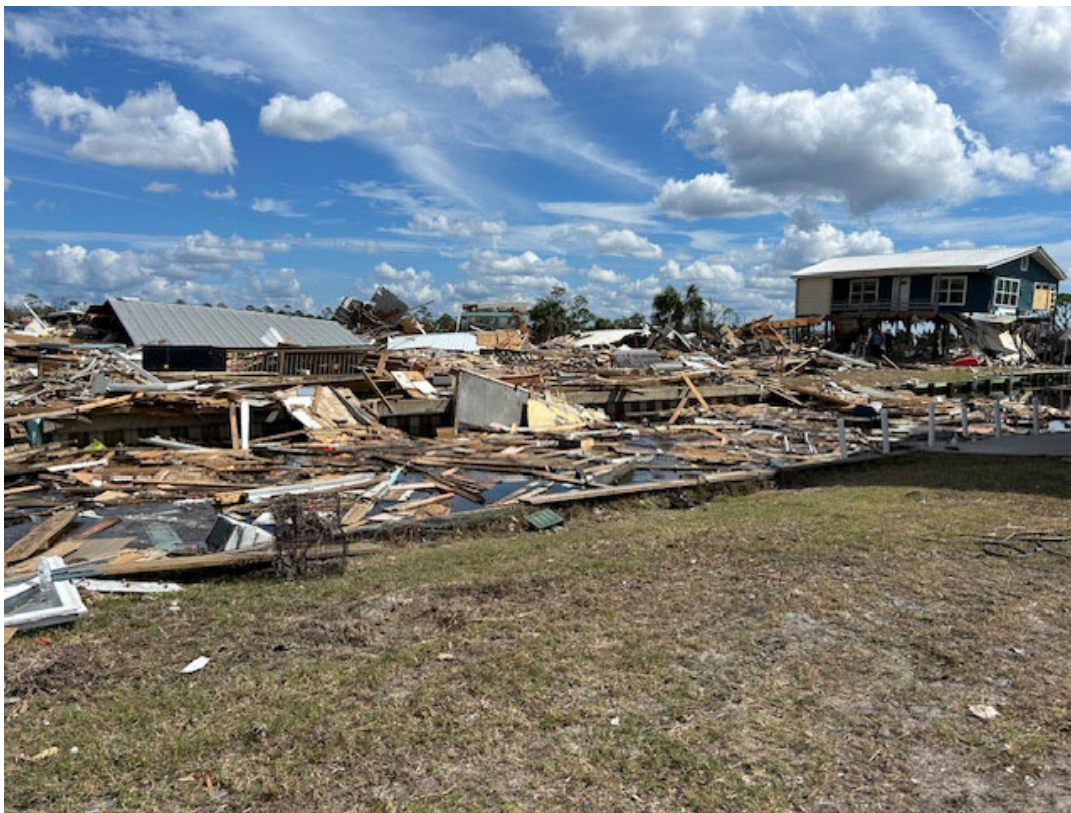
Figure 14. Catastrophic damage in Dekle Beach.
