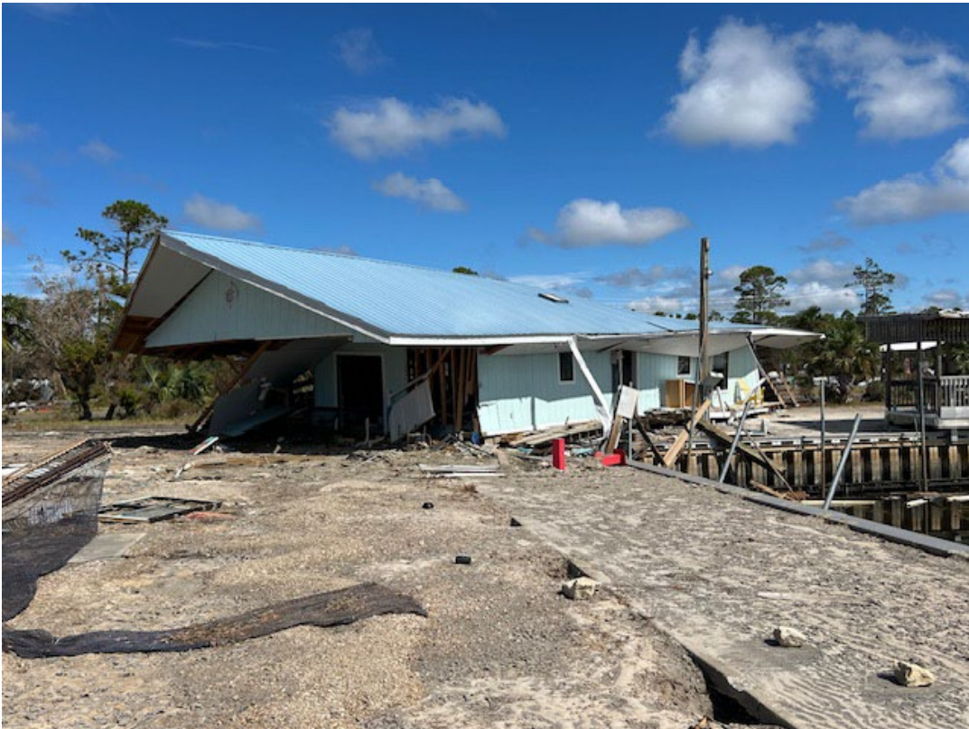
Figure 19. Keaton Beach dwelling on a road blocking access.
