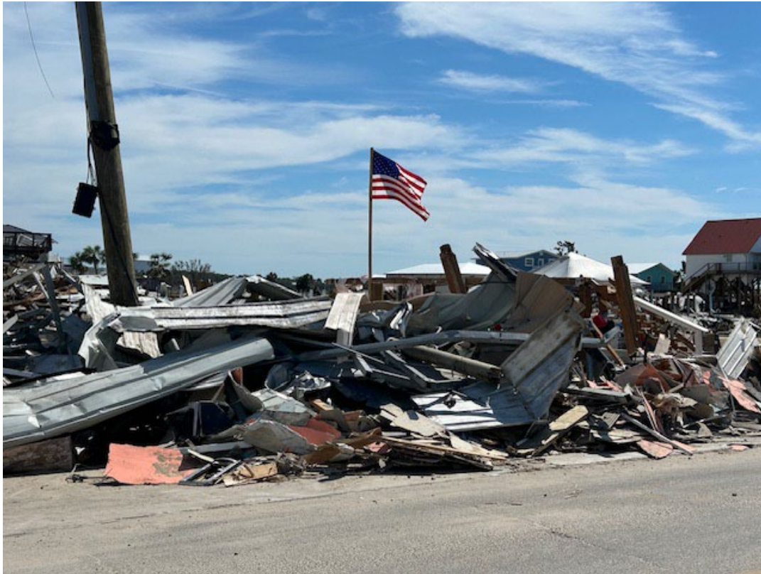
Figure 16. Catastrophic damage in Keaton Beach.
