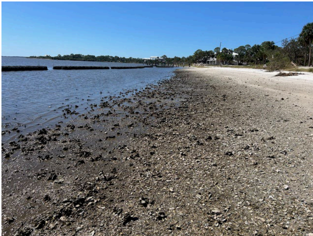
Figure 58. Airport Road eroded beach after Helene.
