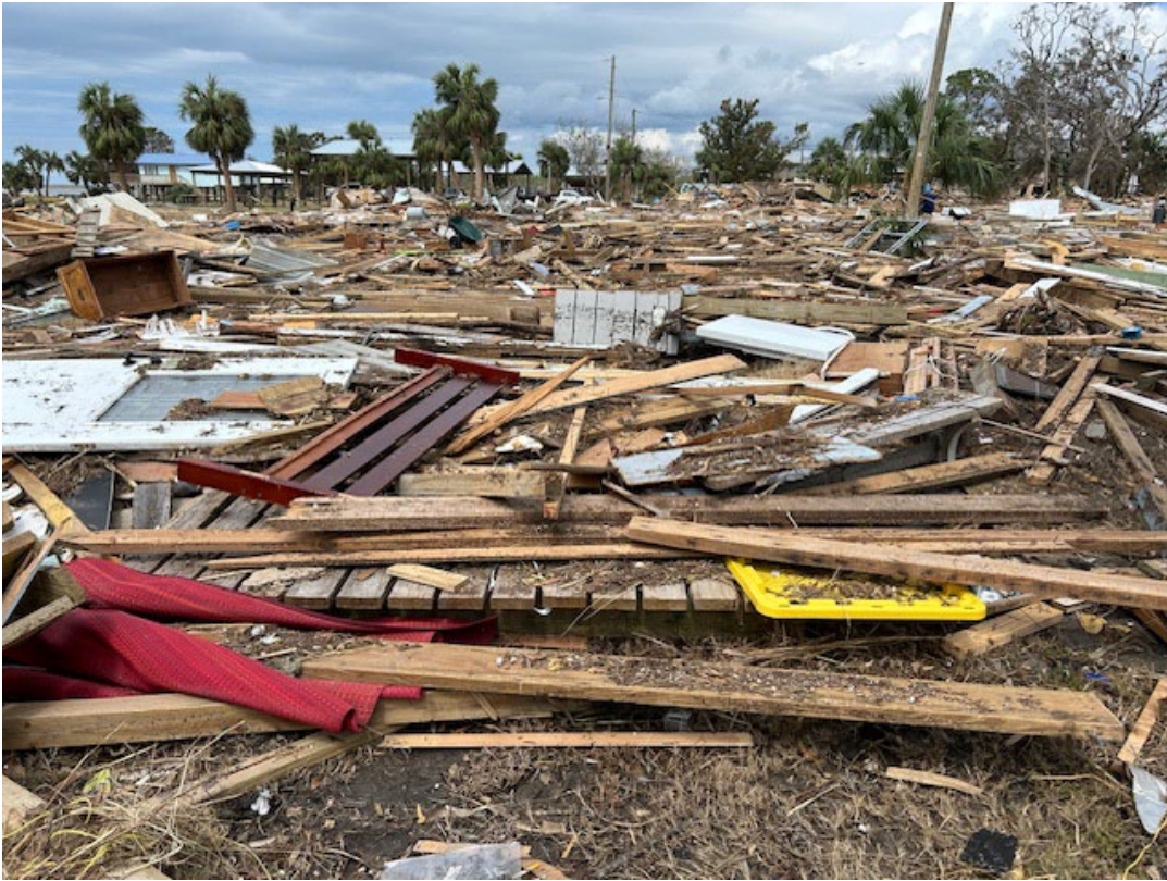
Figure 38. Catastrophic damage in Horseshoe Beach from Helene.
