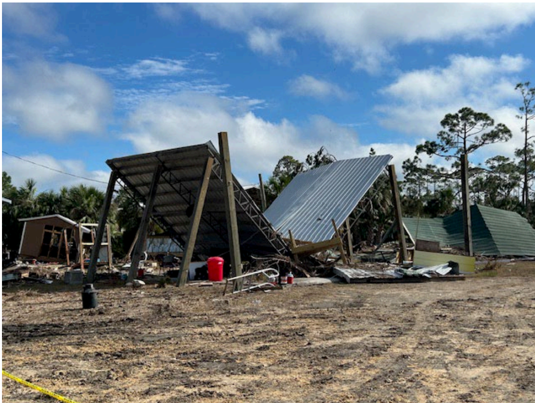
Figure 24. Recreation vehicle shelter destroyed on Cedar Island.
