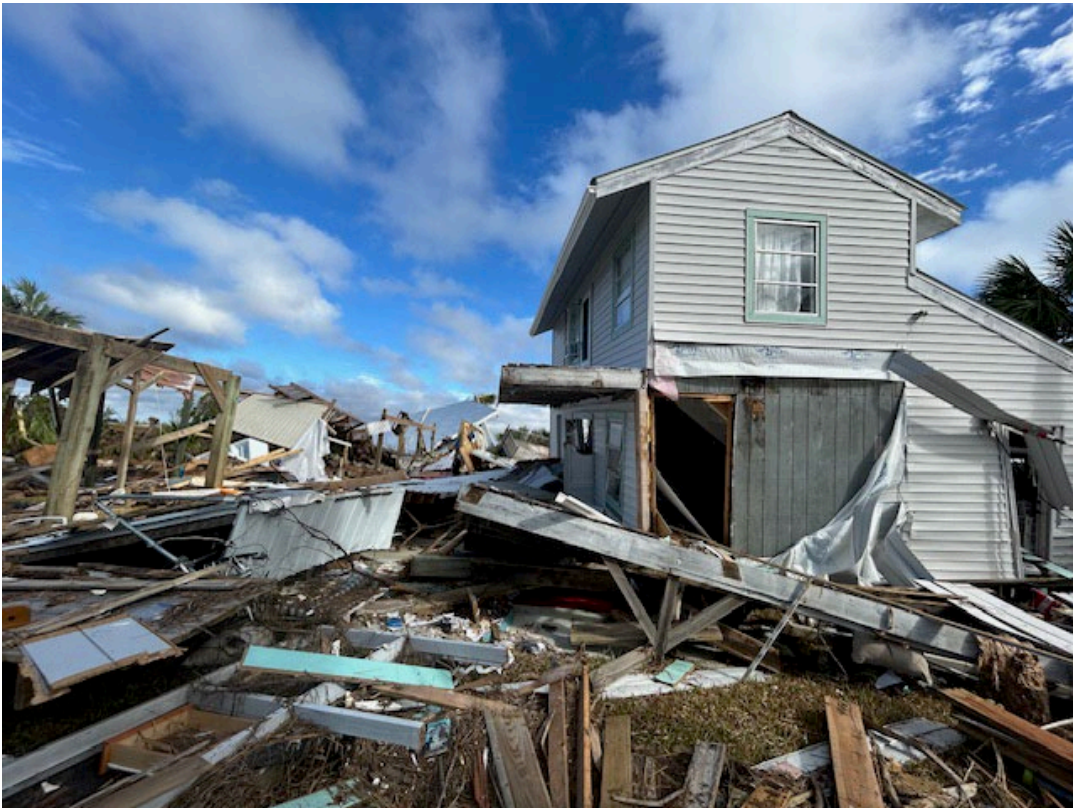
Figure 22. Catastrophic damage on Cedar Island.
