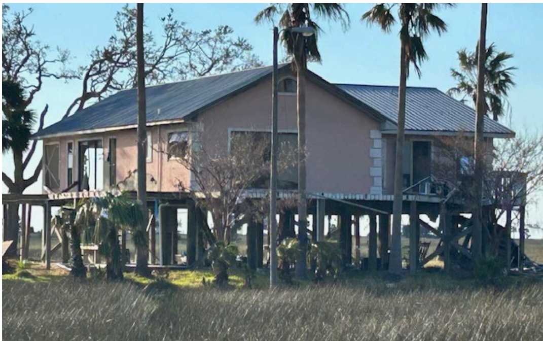
Figure 28. Damaged house on Bird Island.
