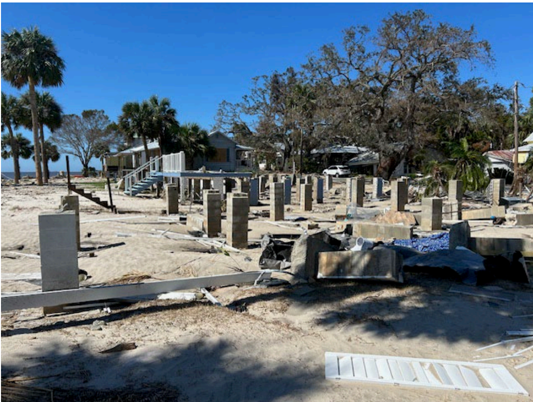
Figure 62. Three single-family dwellings destroyed on 1st Street, Cedar Key.
