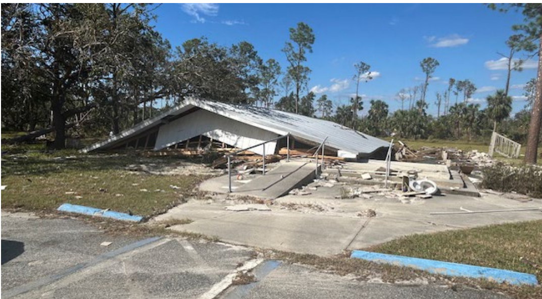
Figure 42. Grade level church building destroyed in Horseshoe Beach.
