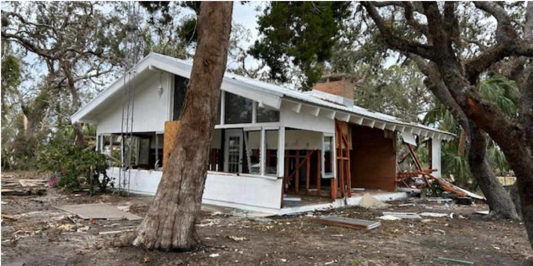
Figure 40. Grade level dwelling destroyed in Horseshoe Beach.
