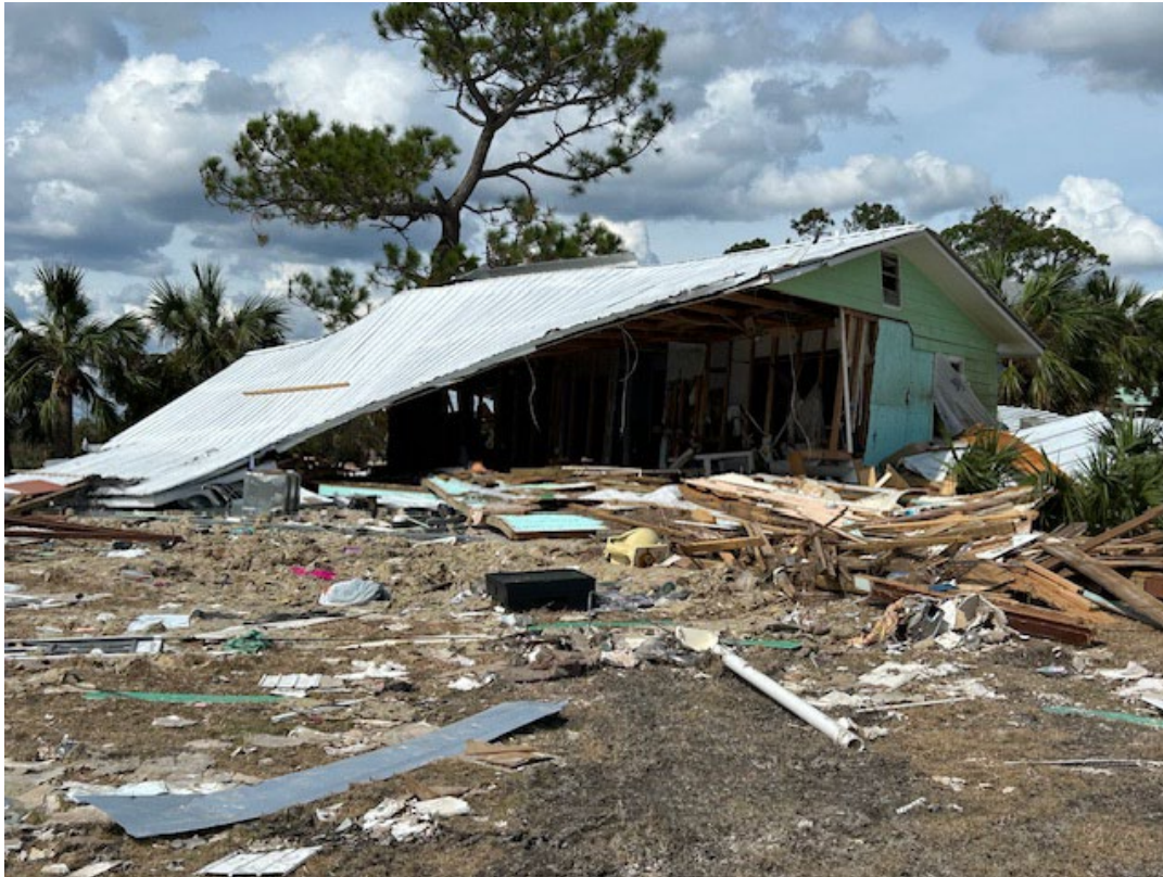
Figure 15. Dekle Beach dwelling destroyed.
