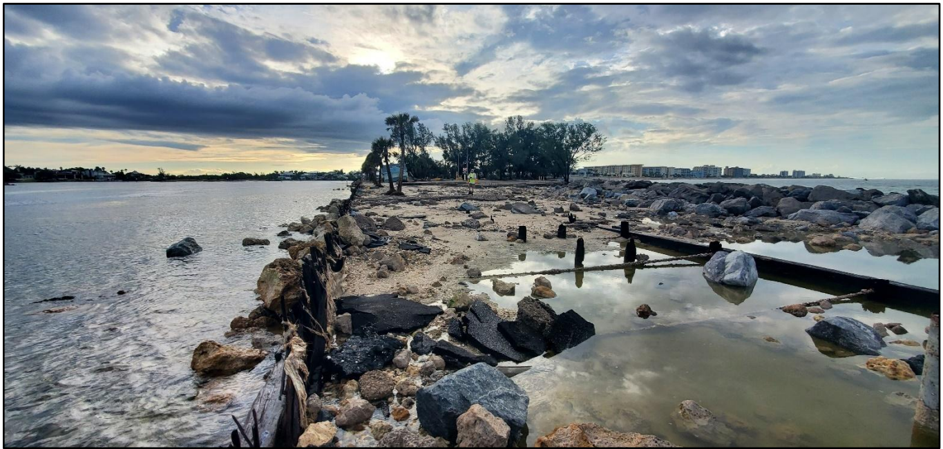
Figure 98. Major damage to Humphris Park and Venice Inlet south jetty and bulkhead by Helene, R-115.
