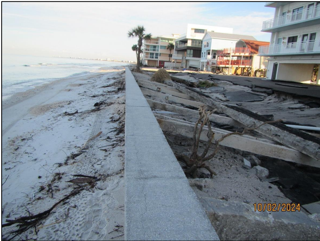
Figure 23. Seawall damage in Treasure Island/ Sunset Beach due to Hurricane Helene near R-139.
