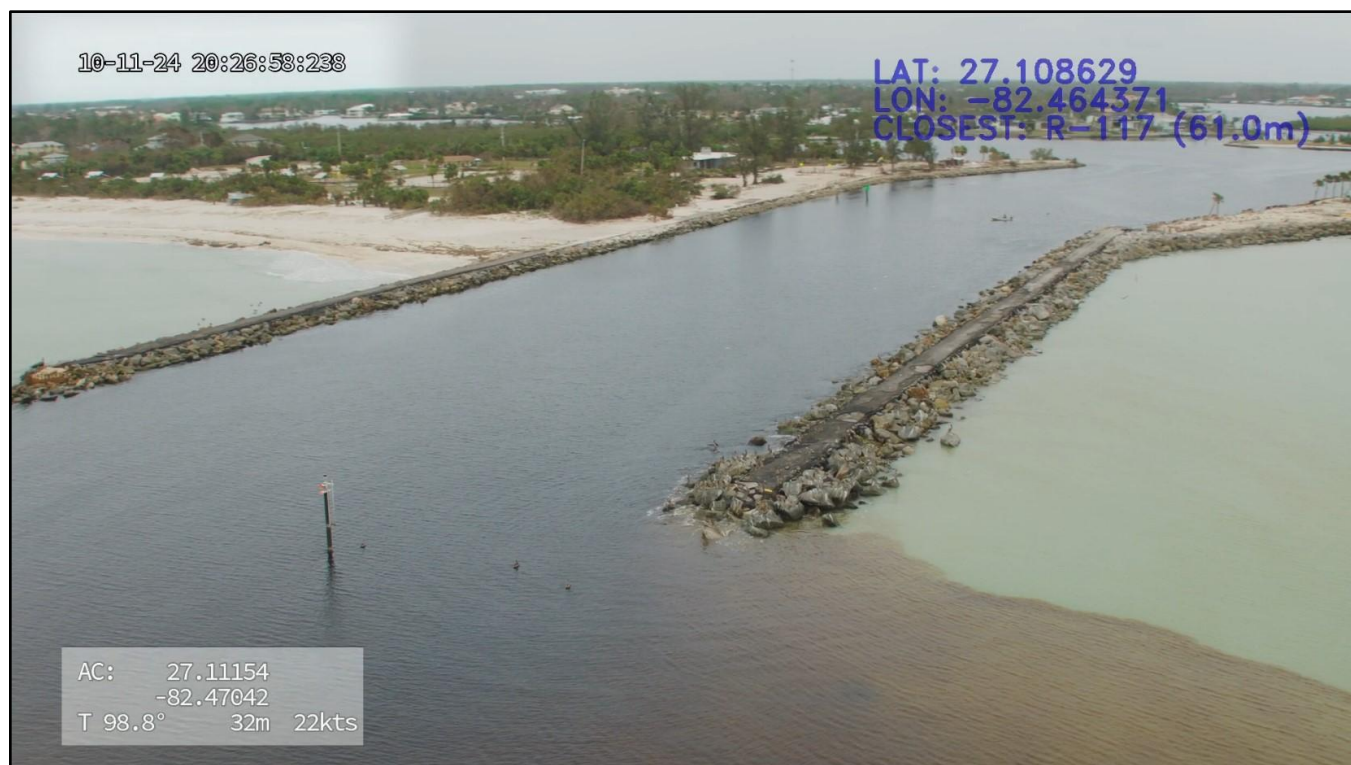
Figure 96. Major damage to the jetties of Venice Inlet by Helene and Milton.
