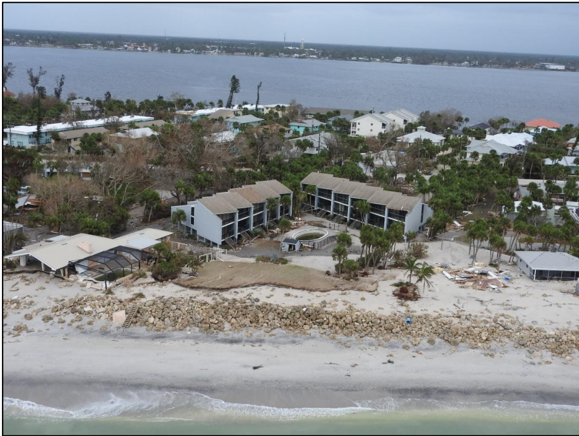
Figure 107. Major beach erosion and rock revetment damage following Milton at Englewood Beach near R-2.
