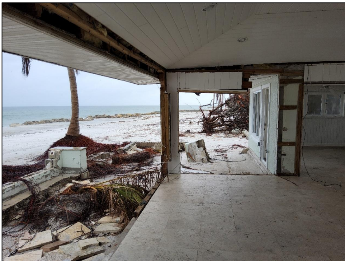
Figure 51. A single-family dwelling destroyed by Helene and major erosion (condition IV) on northern Longboat Key, near R-50.
