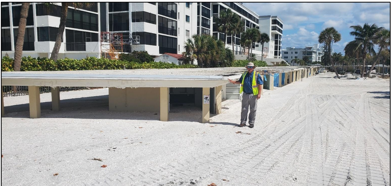
Figure 5710. Major damage to a Lido Key hotel from Helene's storm surge and overwash deposit of approximately three to four feet of beach sand near R-40.
