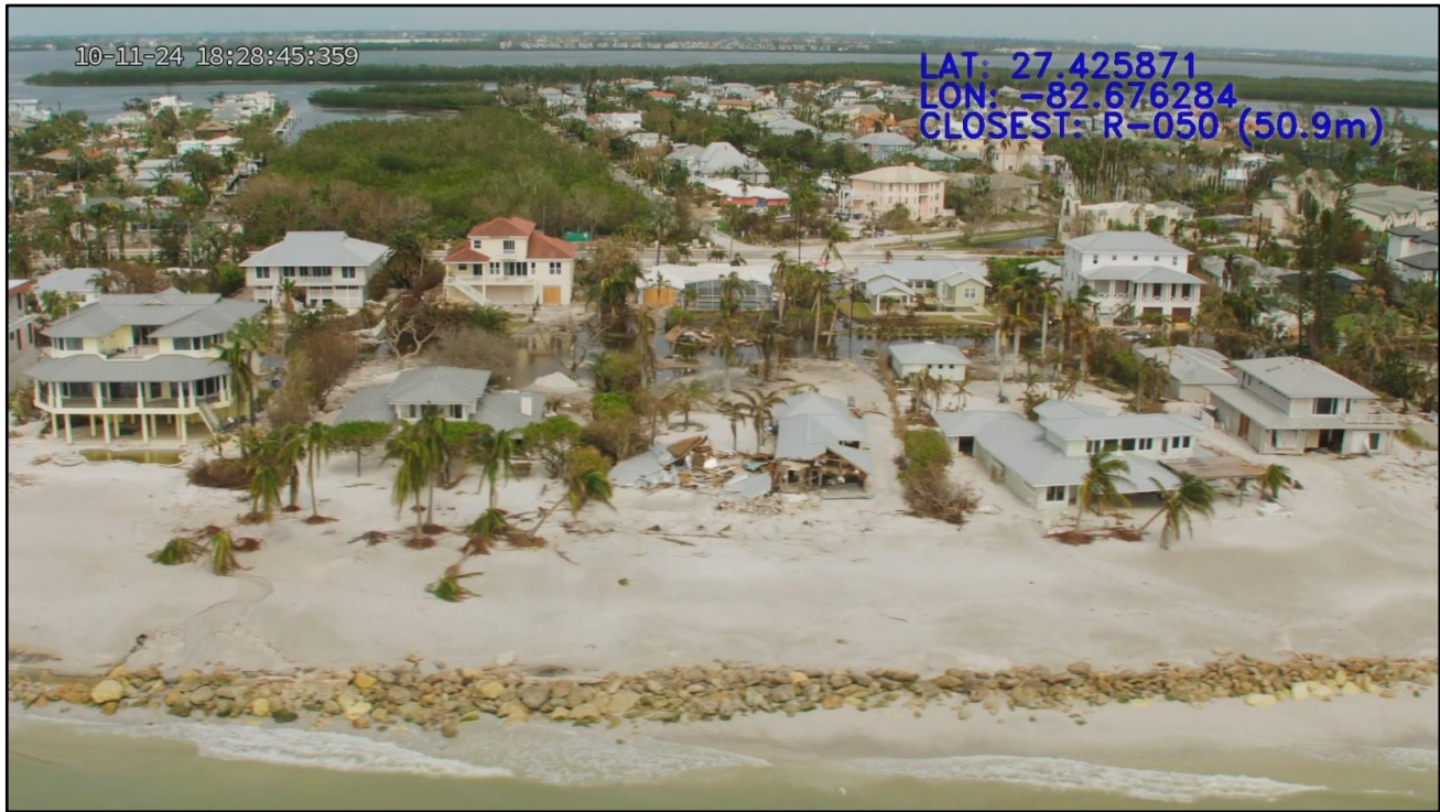
Figure 497. A single-family dwelling destroyed, armoring damage and major beach and dune erosion (condition IV) following Helene and Milton on Longboat Key near R-50.
