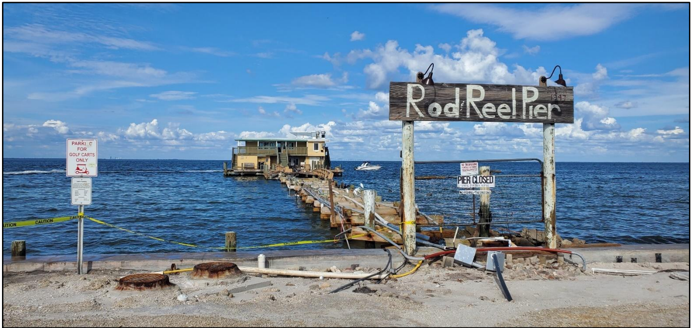
Figure 35. Major deck damage to the Rod and Reel Pier by Hurricane Helene at the northeast end of Anna Maria Island near R-1.
