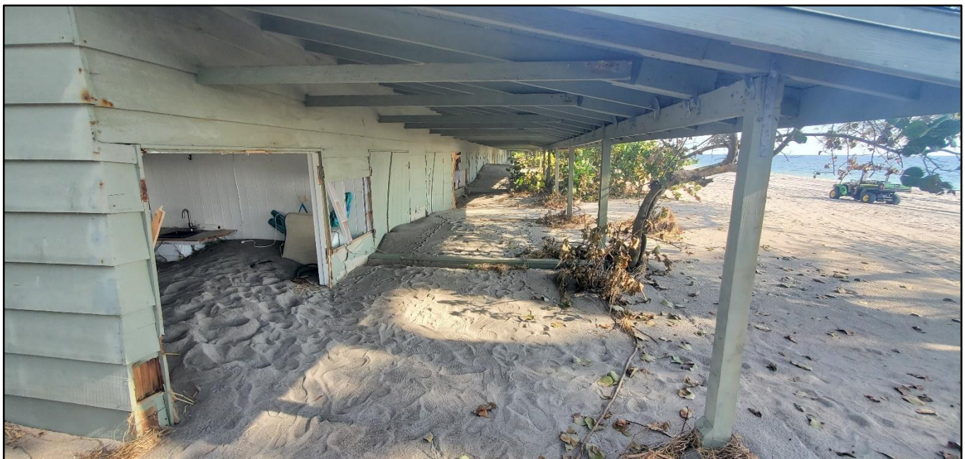
Figure 86. Damaged and sanded beach cabanas impacted by Helene's storm surge at Turtle Beach on Siesta Key near R-71.
