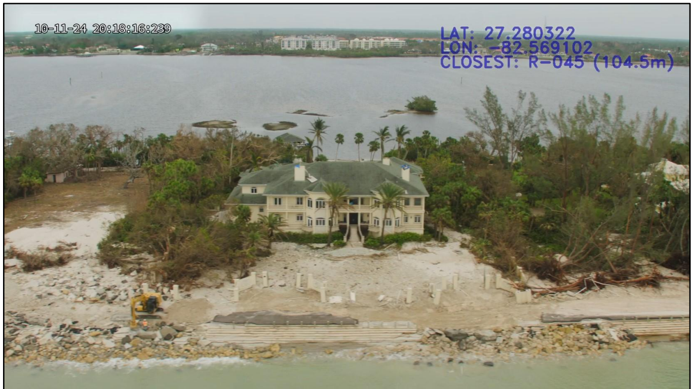
Figure 89. Major road and revetment damages from Helene's storm surge on Casey Key near R-85.
