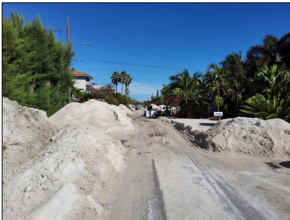
Figure 29. Beach sand piled up on either side of the roadway following road scraping of Helene's overwash deposit at Avenue E, Anna Maria Island near R-24.
