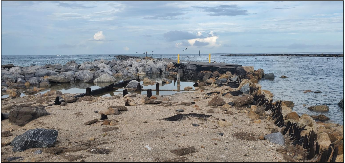
Figure 99. Major damage to Venice Inlet south jetty and bulkhead by Helene, R-115.
