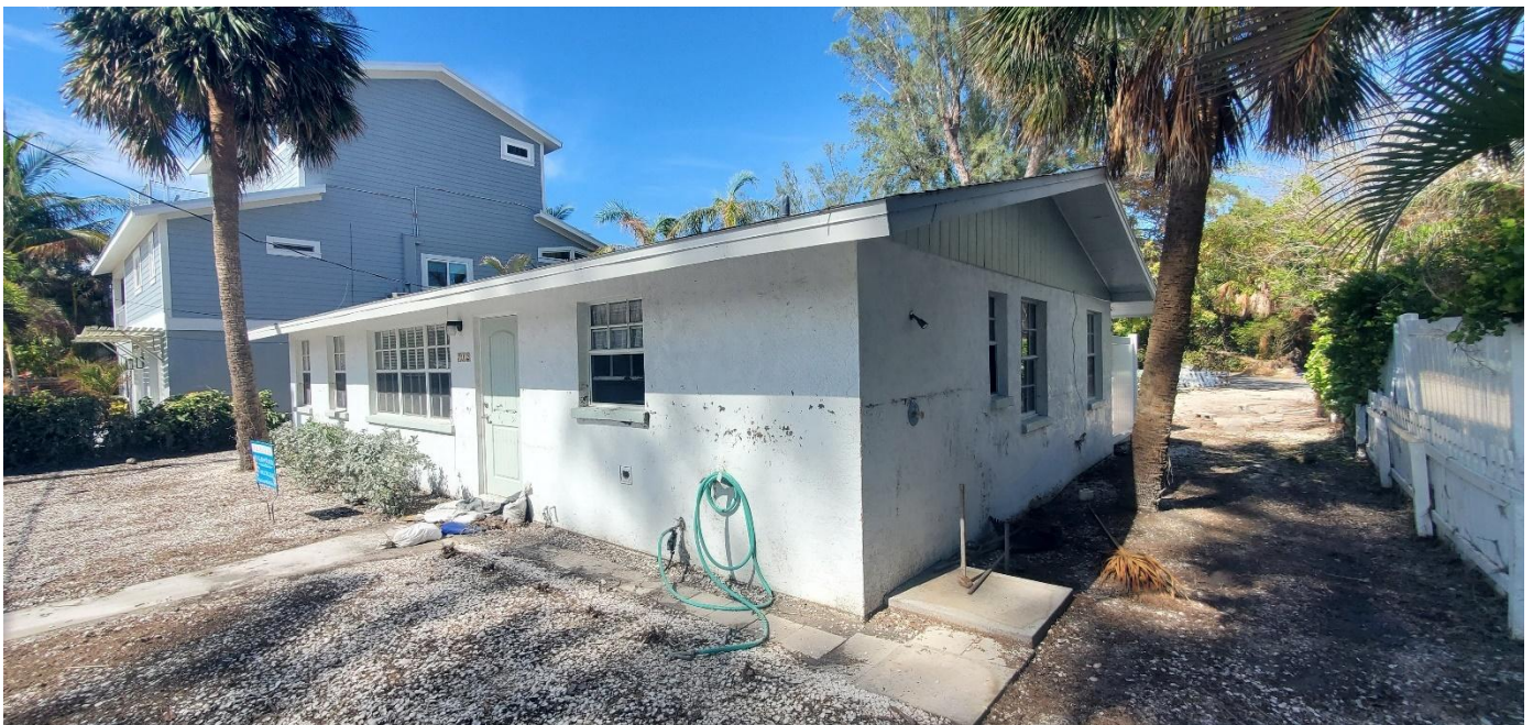
Figure 46. A single-family dwelling flooded by Helene’s storm surge on Anna Maria Island. Note the high water mark above the outdoor shower handle and the front window base.
