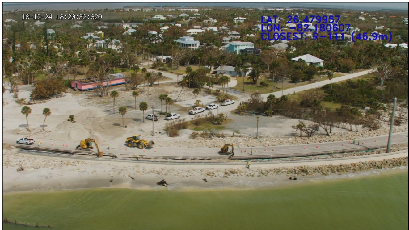
Figure 144. 120 feet of road damage on northern Sanibel Island near R-110.
