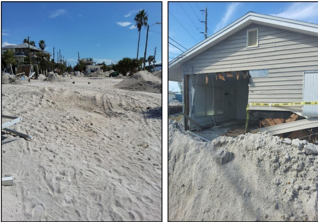
Figure 18. Overwash due to Helene's storm surge on Treasure Island near R-137 (left) and R-139 (right).
