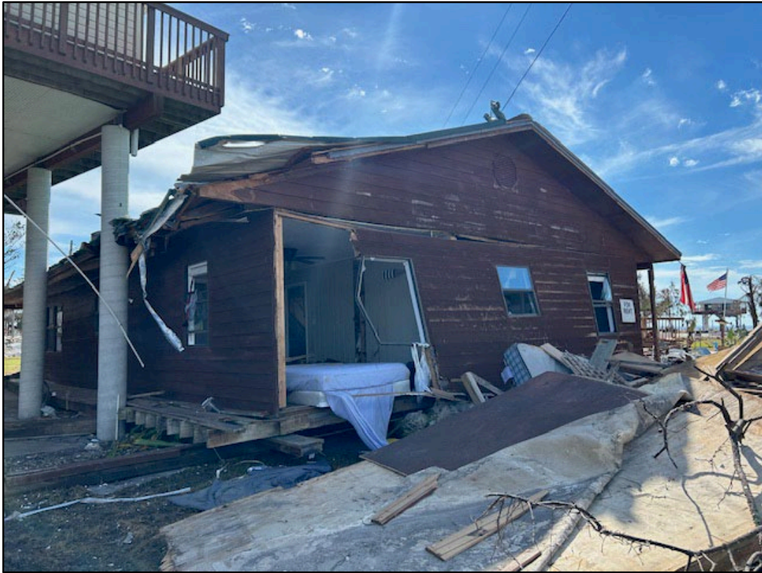
Figure 19. Keaton Beach dwelling carried across a canal and deposited on a neighbor’s driveway.
