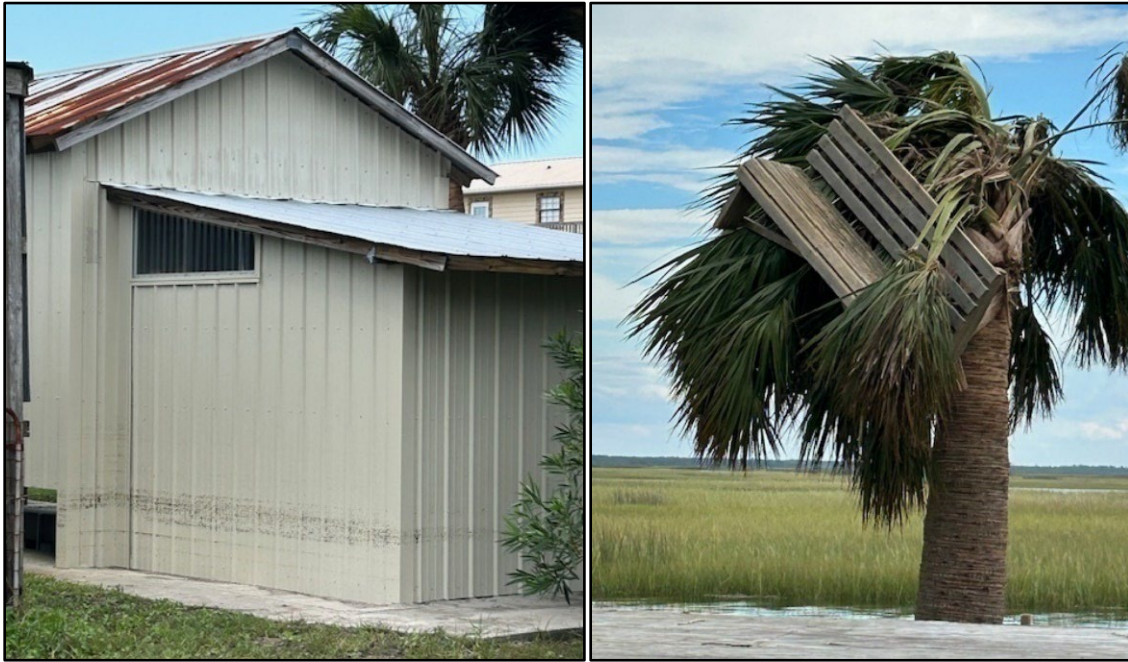
Figure 30. High water indicators for Debby on the left and Helene to the right.
