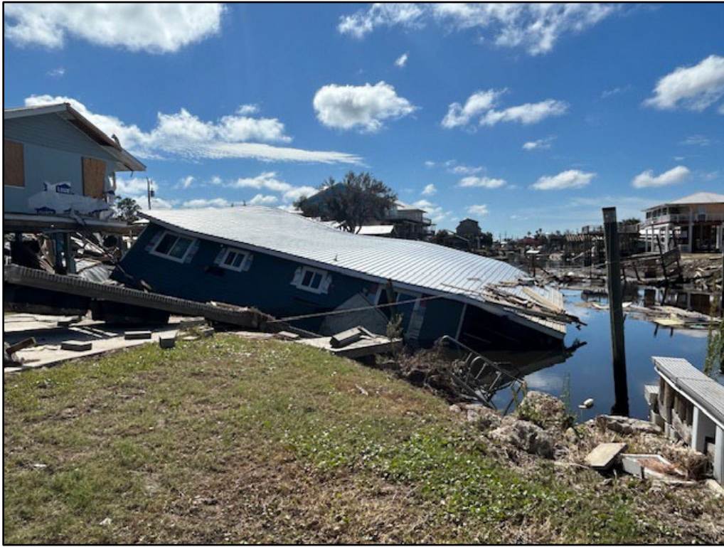
Figure 17. Keaton Beach dwelling in a canal.
