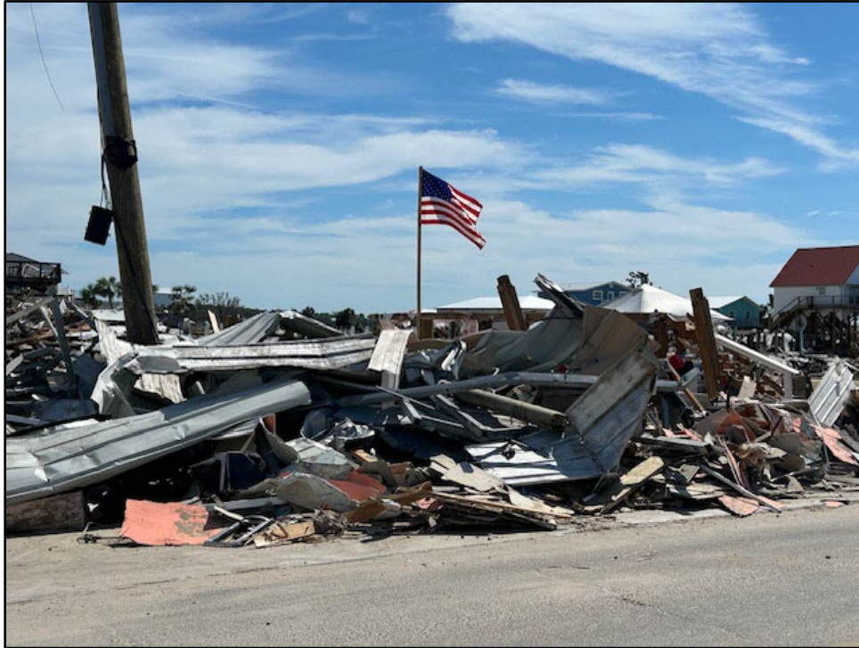
Figure 15. Catastrophic damage in Keaton Beach.
