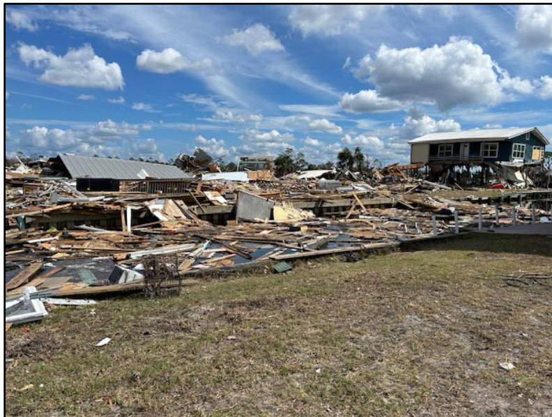
Figure 13. Catastrophic damage in Dekle Beach.
