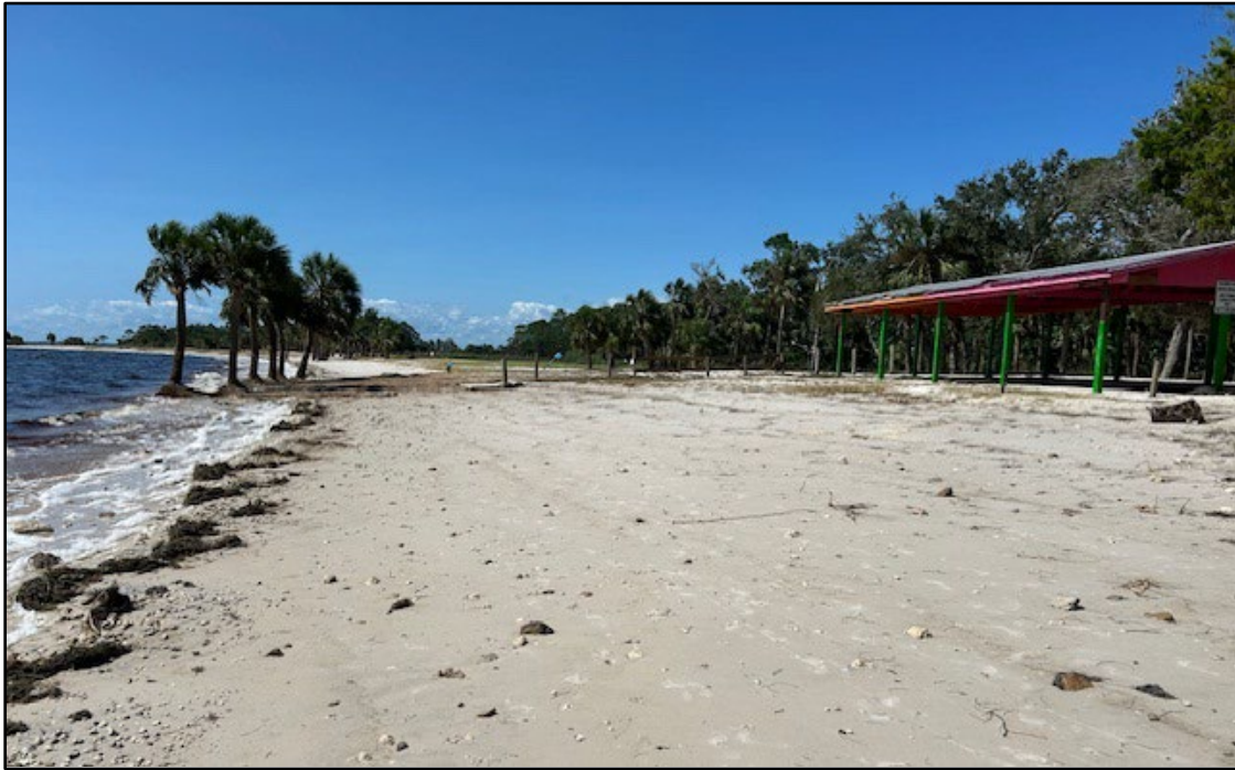
Figure 31. Shired Island beach erosion after Hurricane Debby.
