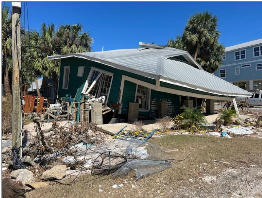
Figure 59. Single-family dwelling destroyed on 1 st Street, Cedar Key.
