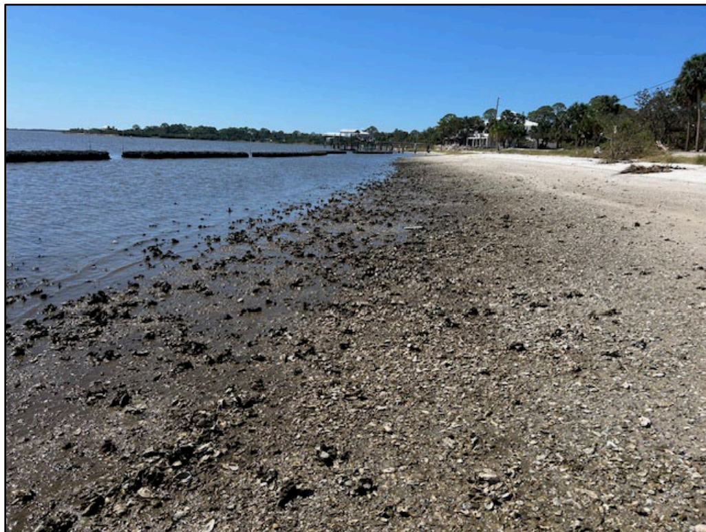
Figure 57. Airport Road eroded beach after Helene.
