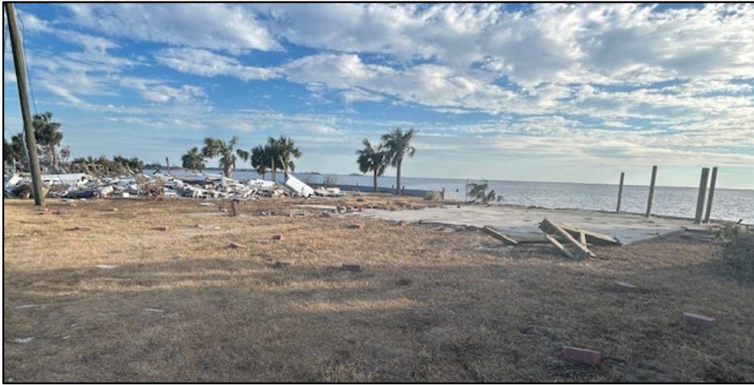
Figure 25. Six single-family dwellings in a row destroyed on Dark Island.
