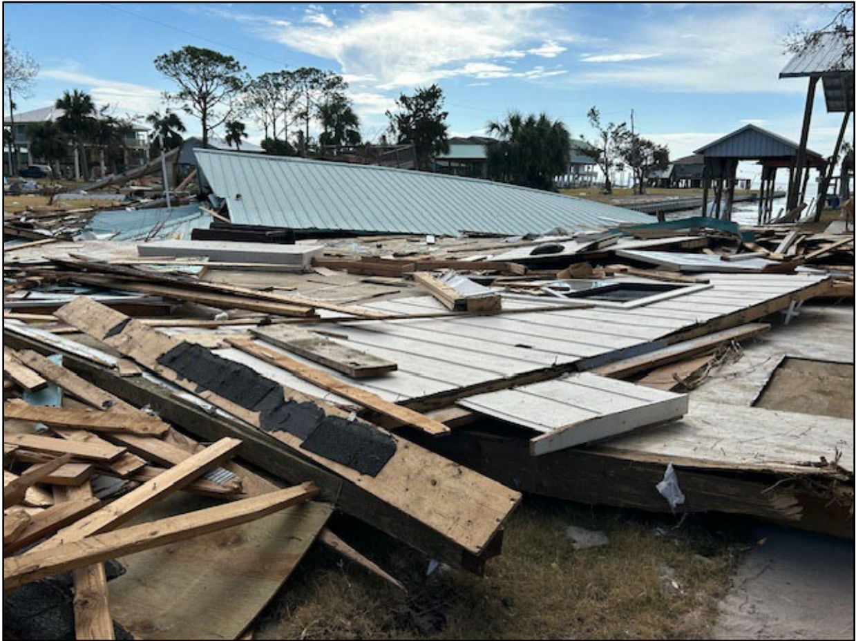
Figure 38. Catastrophic damage in Horseshoe Beach.
