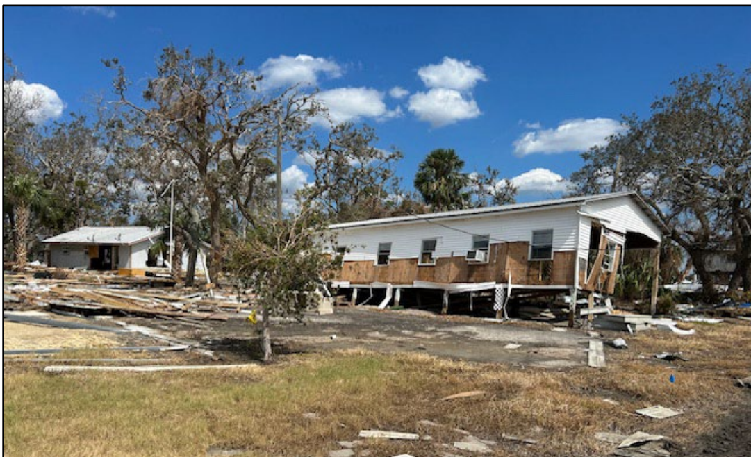
Figure 46. Buildings destroyed with insufficient elevations.
