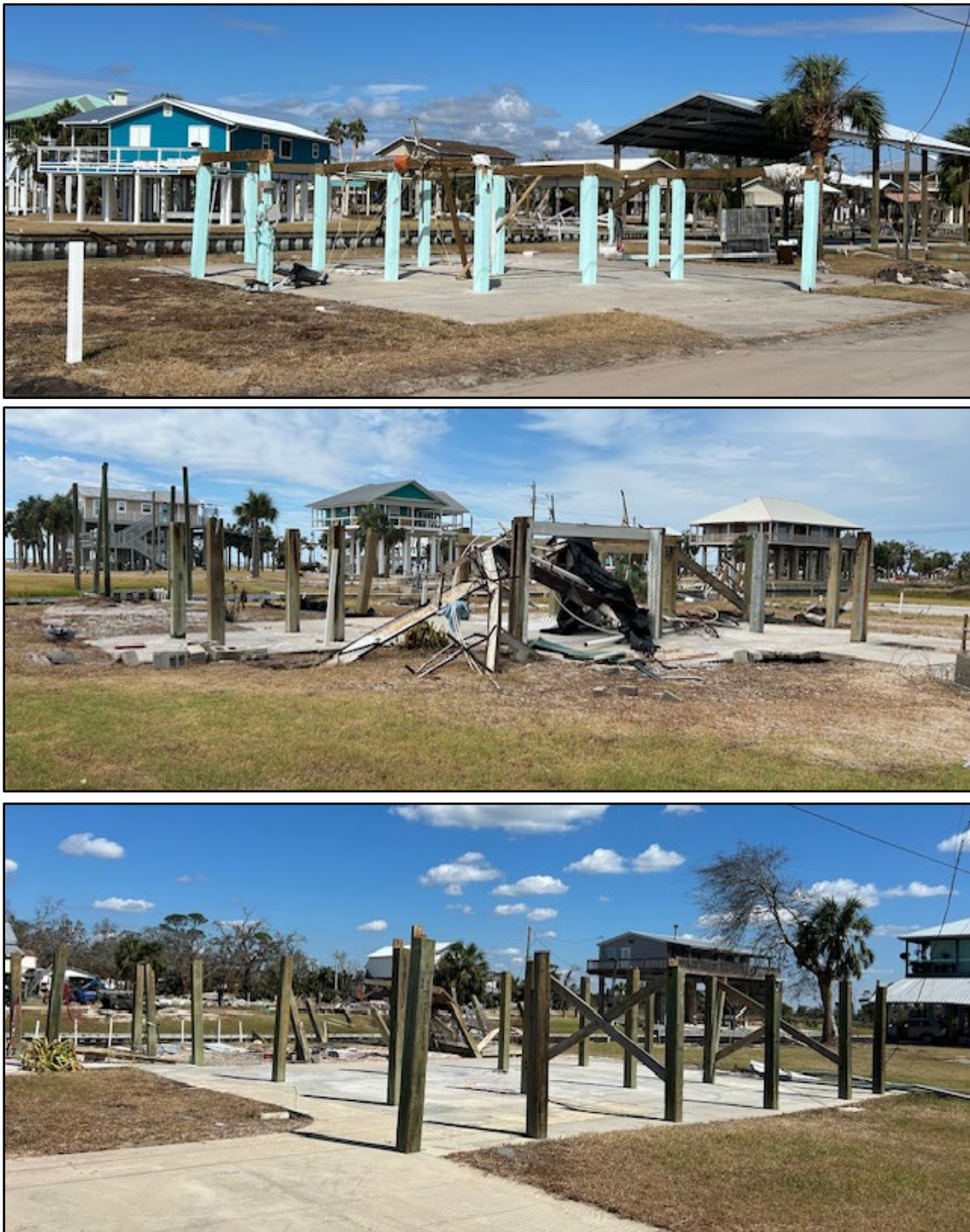
Figure 44. Three pile supported dwellings in Horseshoe Beach destroyed due to insufficient elevation for Helene’s storm surge and waves.
