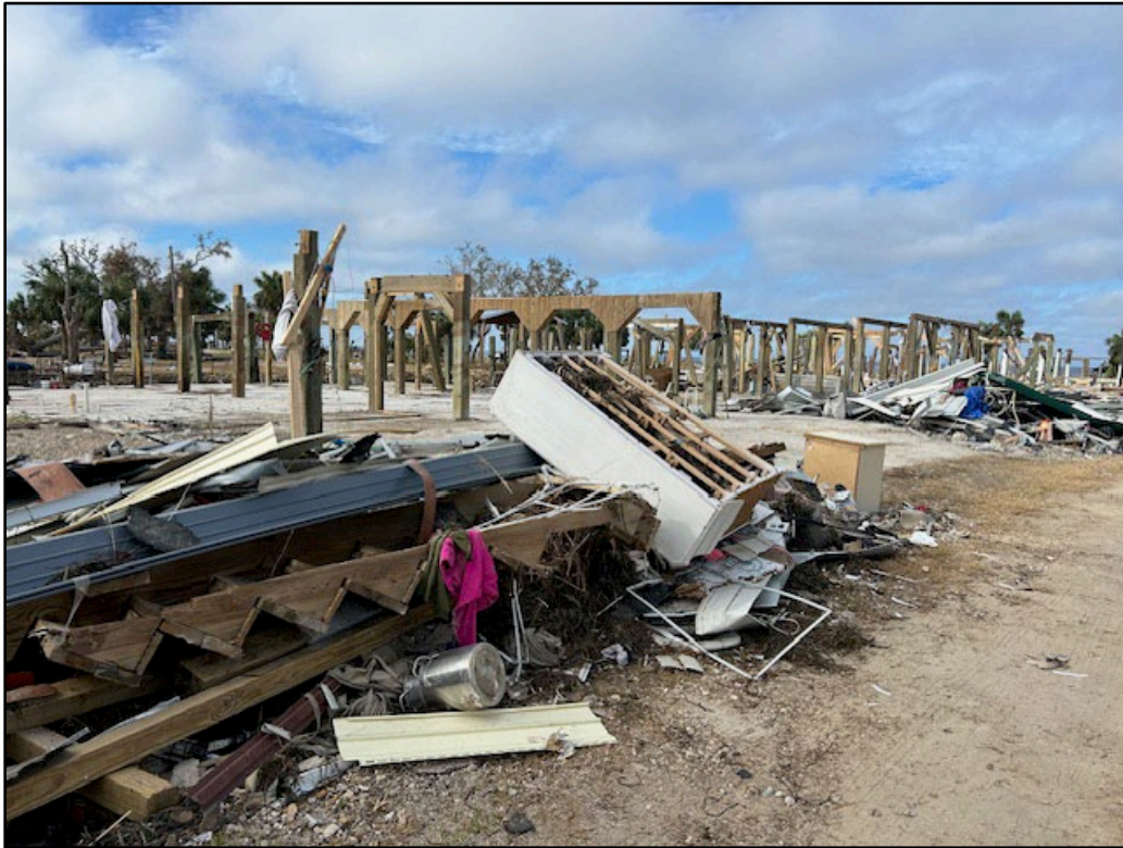
Figure 20. Catastrophic damage on Cedar Island.
