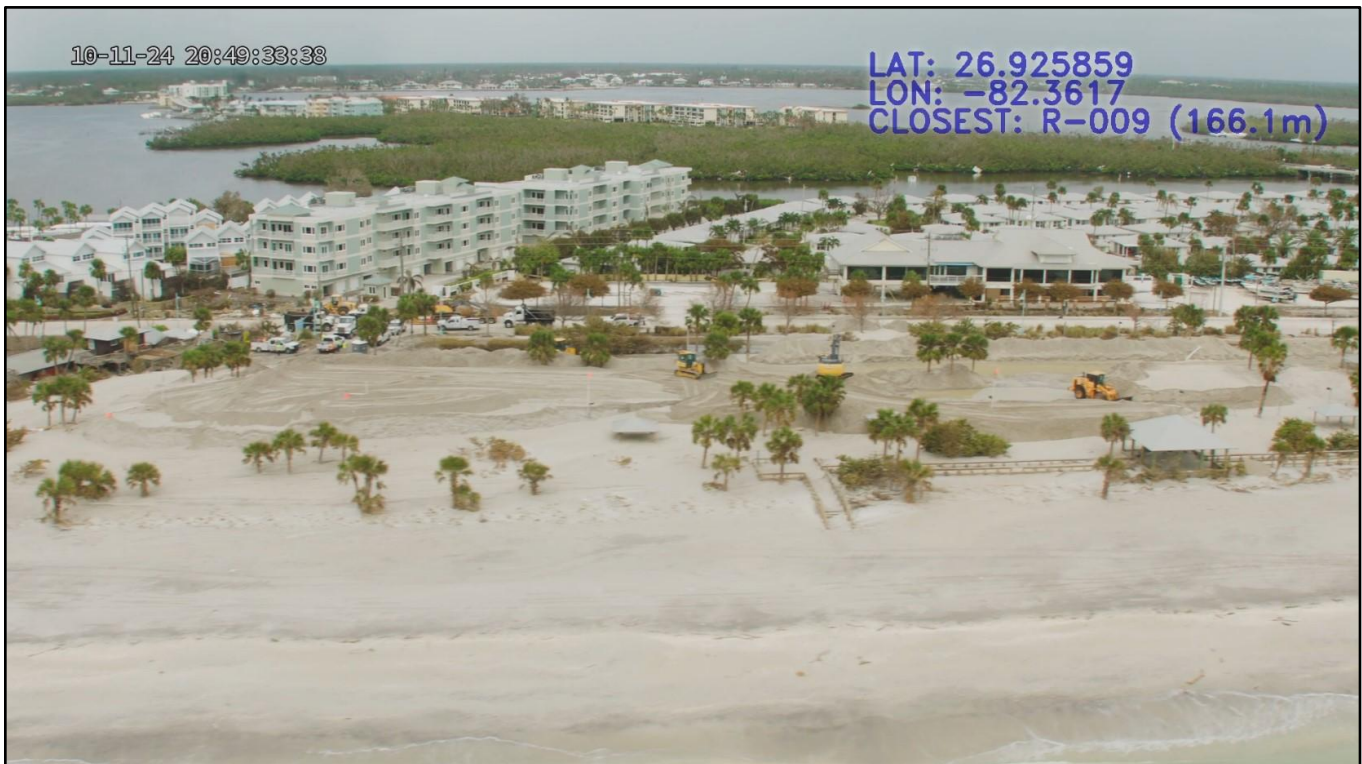
Figure 109. Major beach erosion and sand overwash deposited in parking lot at Englewood Beach Park due to Helene and Milton near R-9.
