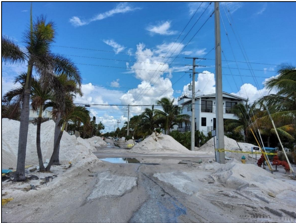
Figure 28. Beach sand piled up on either side of roadway following road scraping of Helene’s overwash deposit at 66 th Street, Anna Maria Island near R-14.
