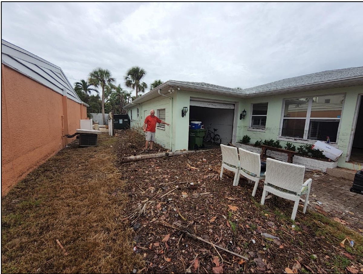
Figure 56. High water mark above a garage window base on home near St. Armands Circle off North Boulevard of the Presidents, Lido Key.
