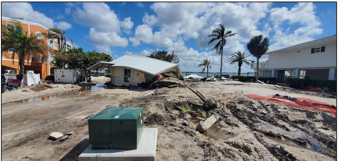
Figure 44. Helene’s storm surge carried a dwelling into the middle of 12th Street South To the bayside from the Gulfside near R-35 on Anna Maria Island.
