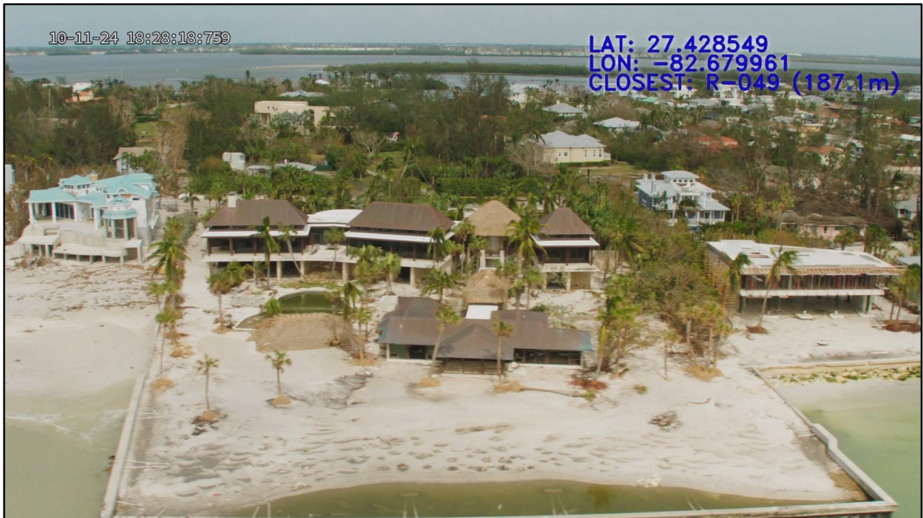
Figure 48. First floor flooding damage, seawall damage and major erosion (condition IV) following Helene and Milton on northern Longboat Key near R-49.
