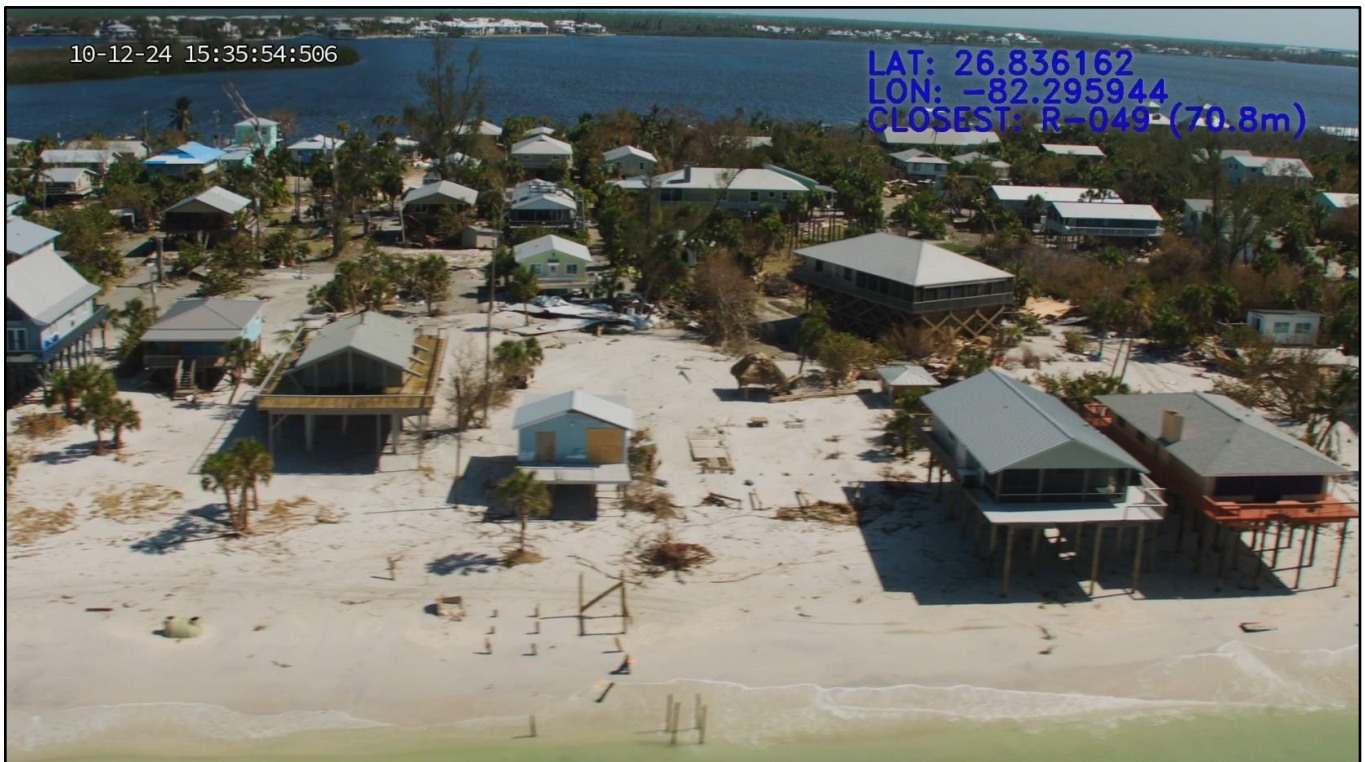
Figure 119. Single-family dwellings destroyed on Little Gasparilla Island by Milton near R-49.
