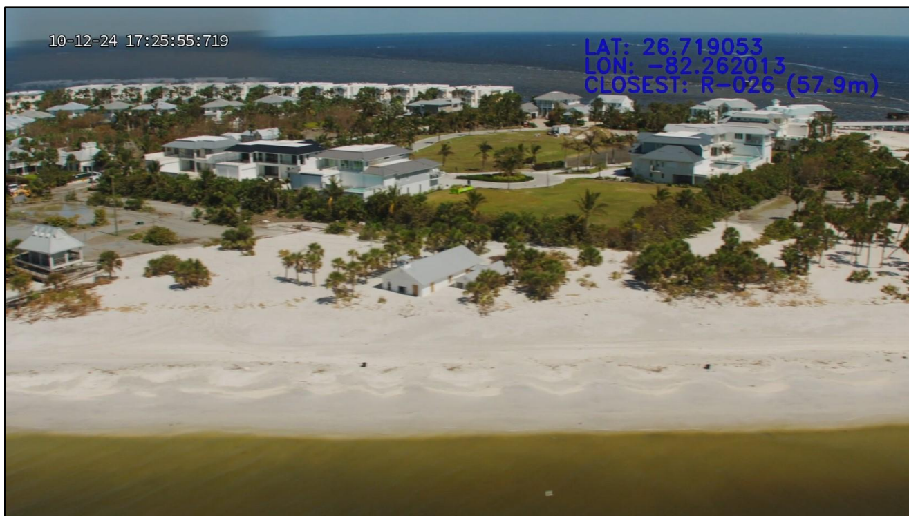
Figure 127. Major beach and dune erosion and storm surge overwash due to Helene and Milton at Gasparilla Island State Park and at a historic church building at R-26.
