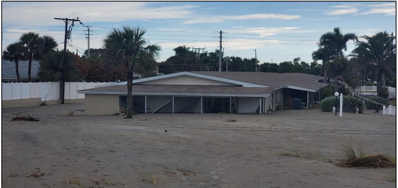
Figure 100. Storm surge damages to Venice Beach apartments near R-117.
