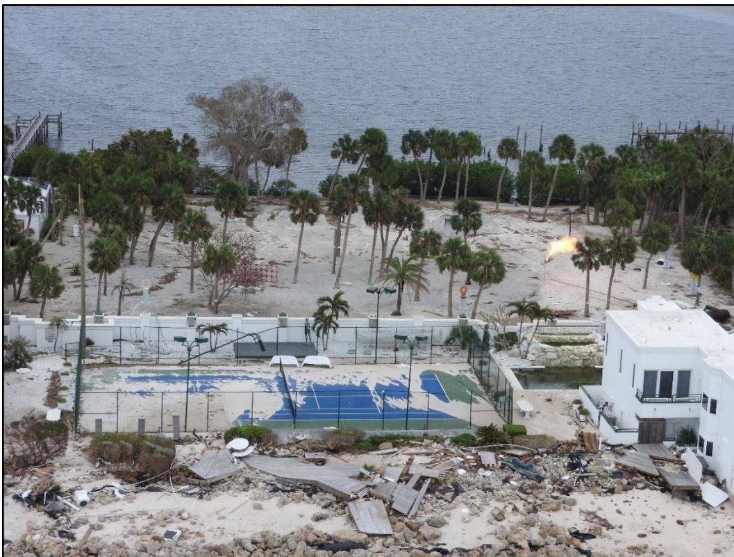
Figure 70. Storm surge overwash impacts including a ruptured gas line on Casey Key near R-87.
