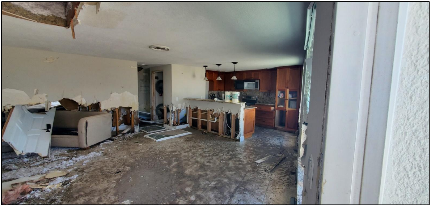
Figure 43. The interior of a single-family dwelling flooded by Helene’s storm surge on Anna Maria Island near R-34.
