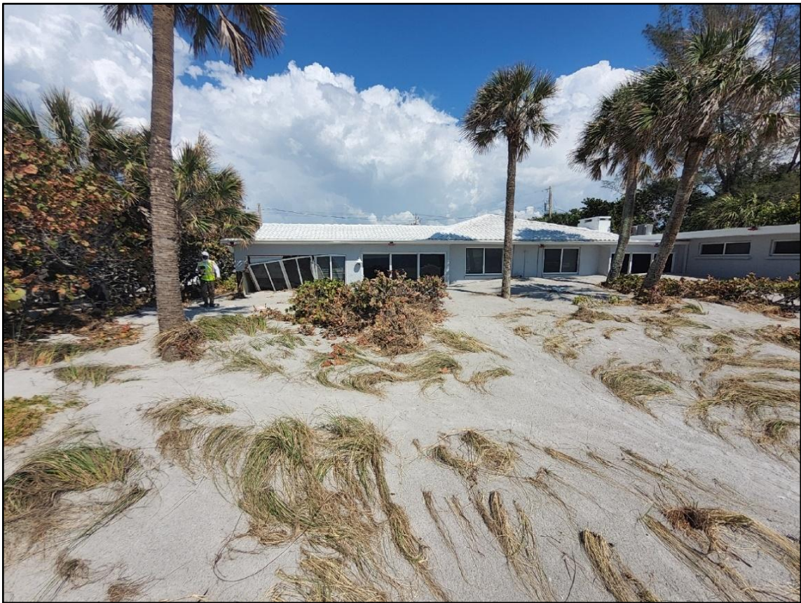
Figure 83. Single-family dwelling damaged by Helene’s storm surge on Longboat Key near R-10.
