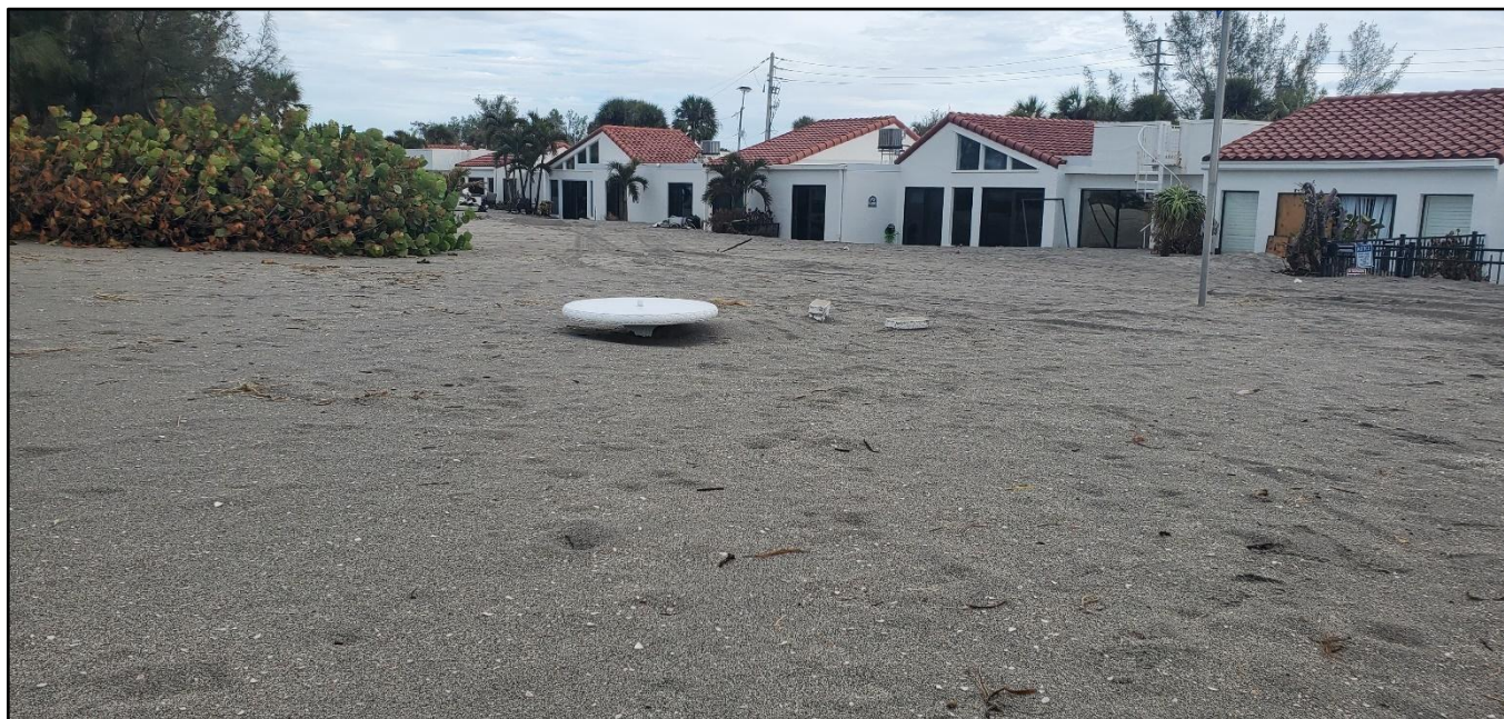
Figure 71. Approximately 2 feet of sand overwash covering concrete table leg and impacting buildings due to Helene’s storm surge at Venice Beach near R-116.
