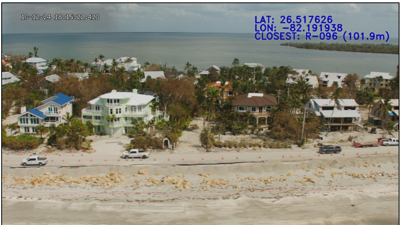
Figure 143. 500 feet of road damage along Captiva Drive on Captiva Island near R-96.
