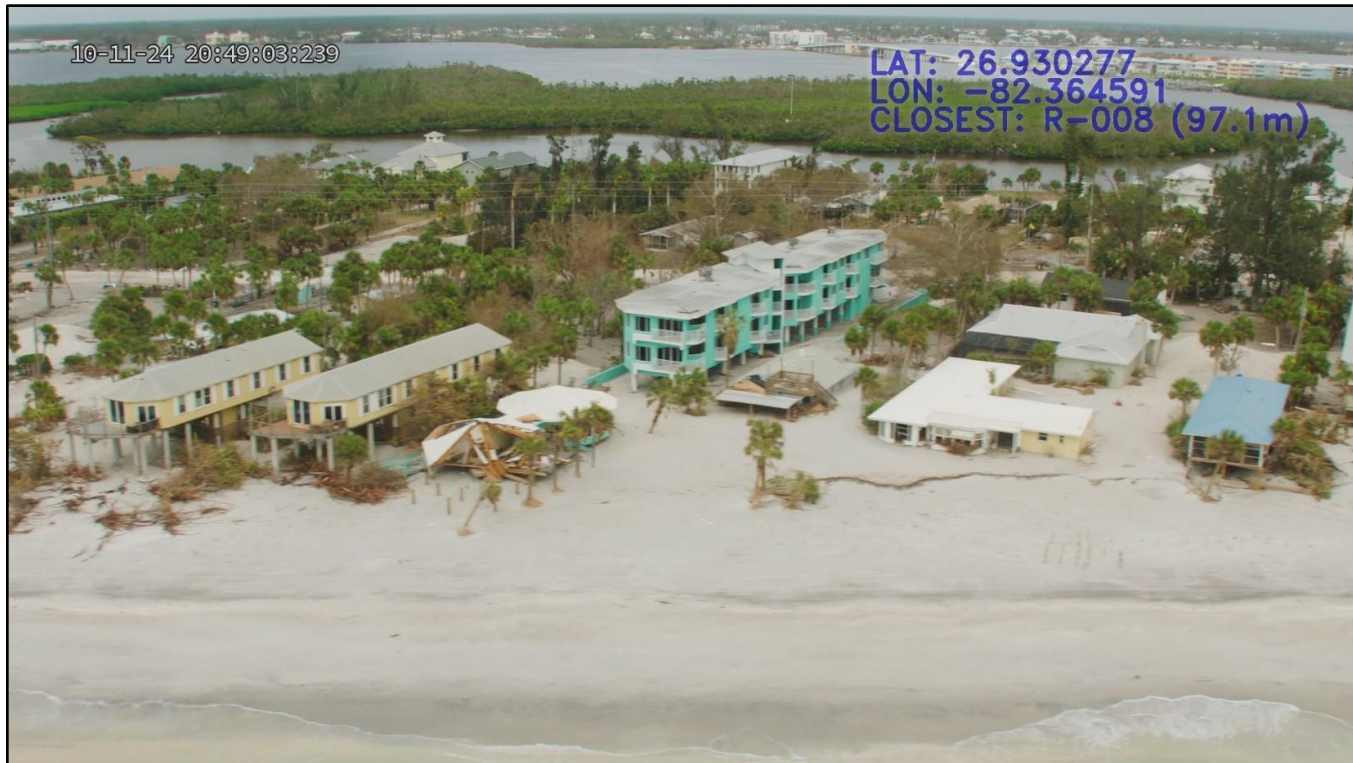
Figure 116. Multi-family dwellings damaged and destroyed by Milton at Englewood Beach near R-8.
