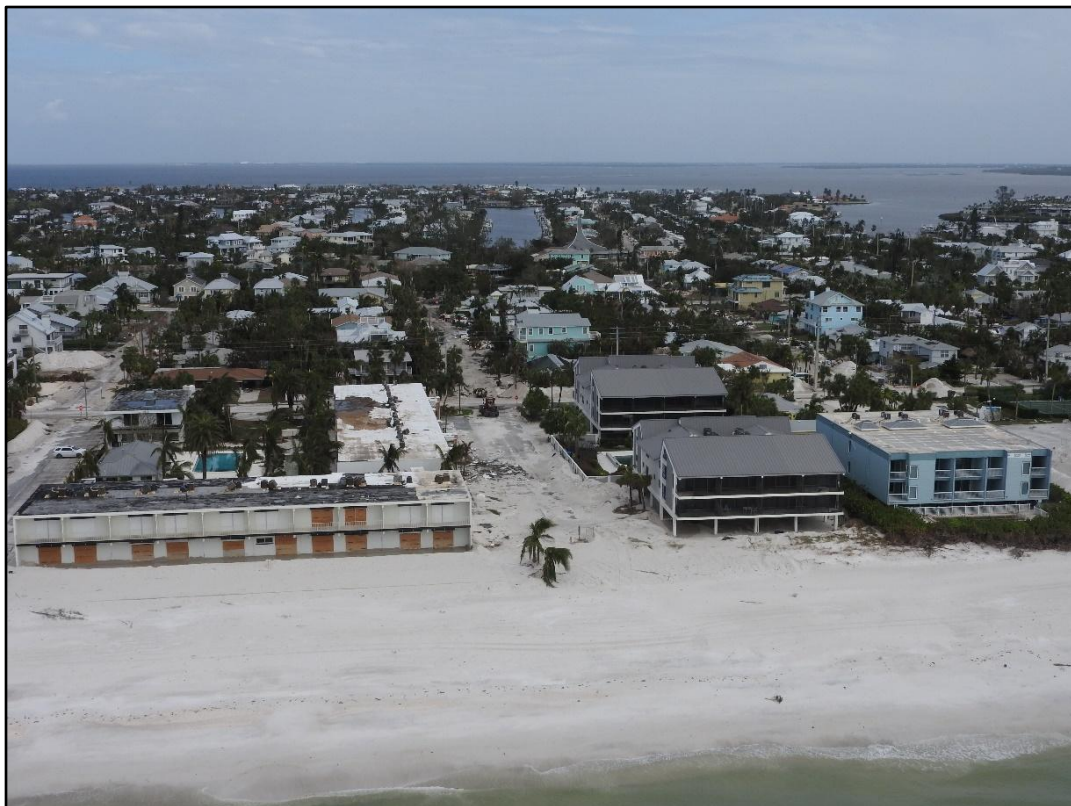
Figure 27. Major beach and dune erosion (condition IV) following Helene and Milton at 68 th Street, Anna Maria Island near R-14.
