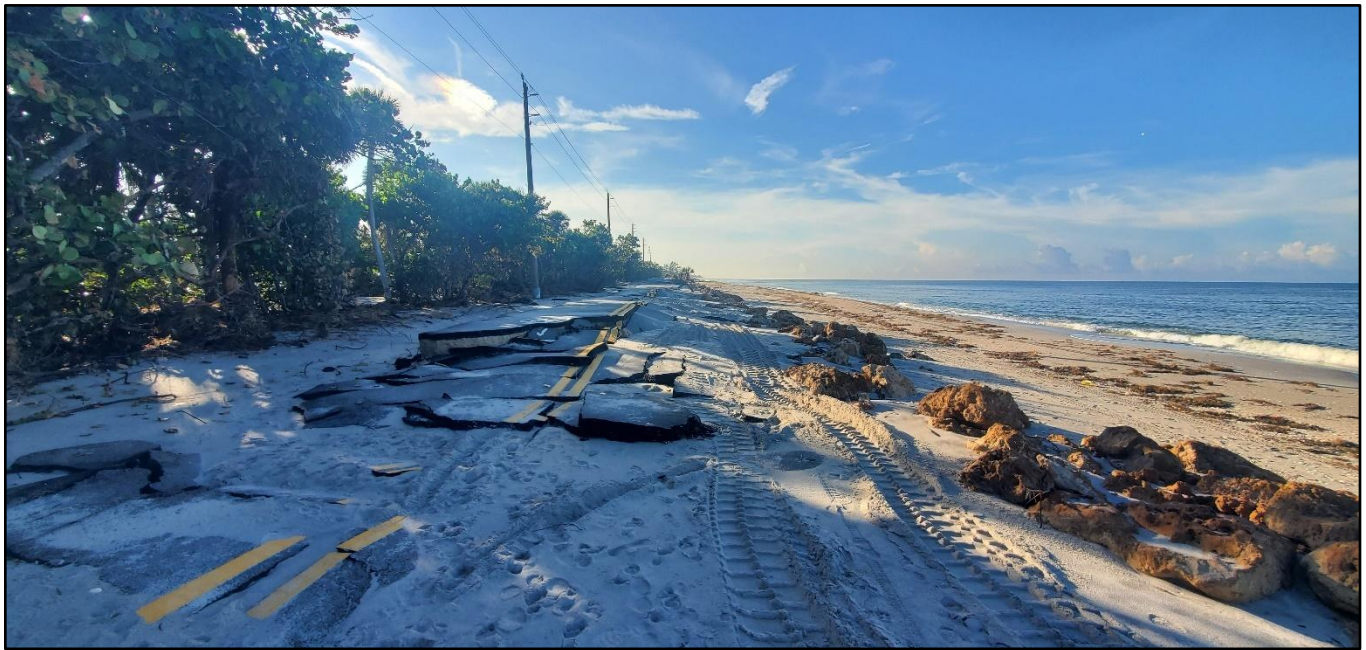
Figure 78. Major beach and dune erosion (condition IV) and major road damage at Blind Pass County Park near R-174.5.
