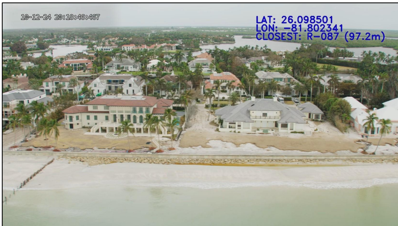
Figure 148. Major beach and dune erosion (condition IV) at Naples near R-87.
