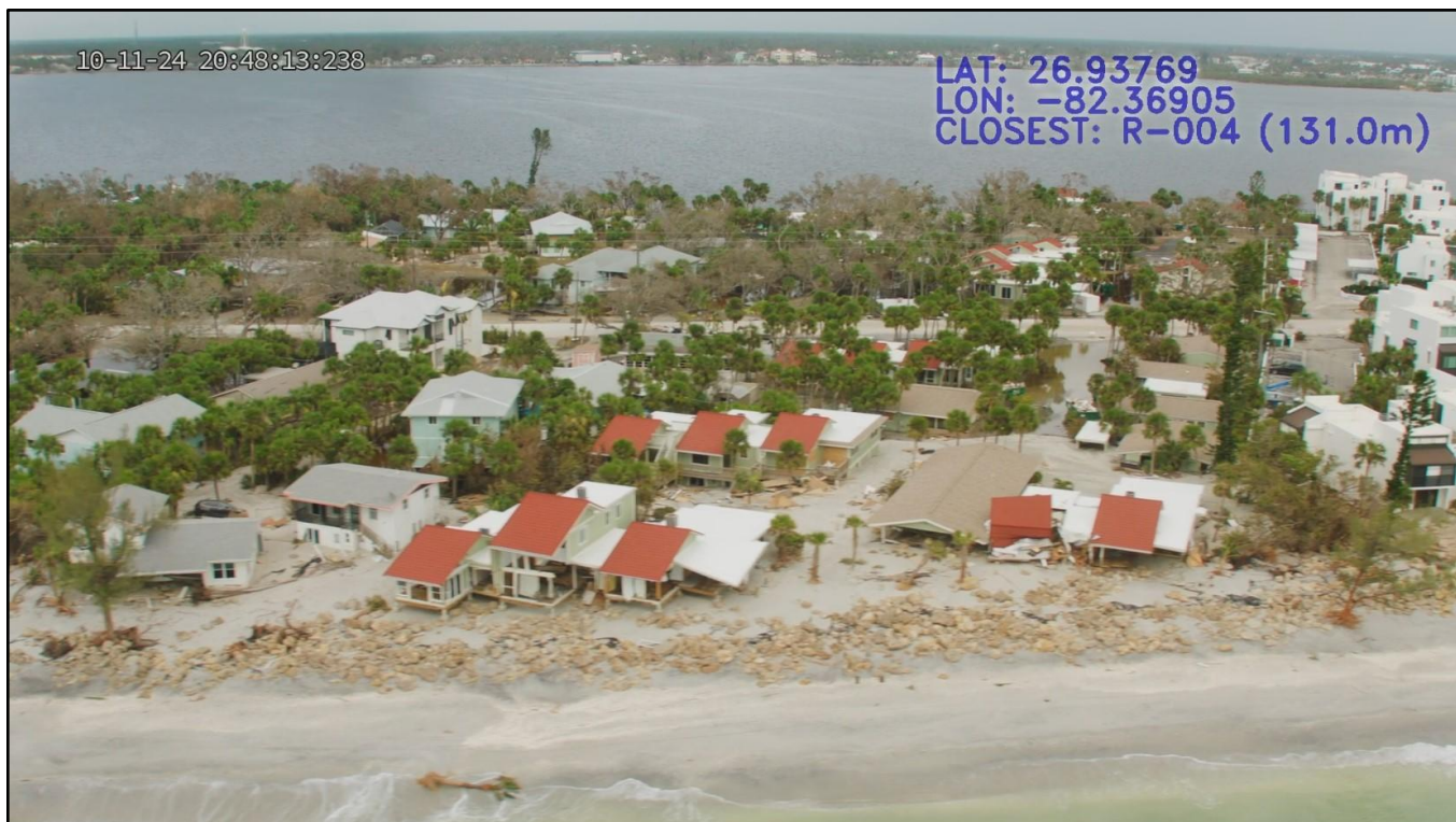
Figure 115. Multi-family dwellings damaged by Milton at Englewood Beach near R-4.
