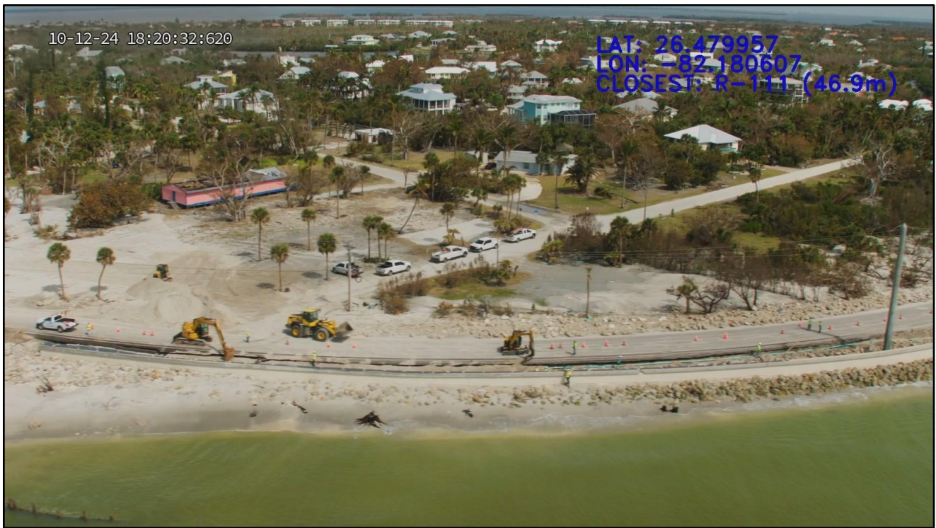
Figure 144. 120 feet of road damage on northern Sanibel Island near R-110.
