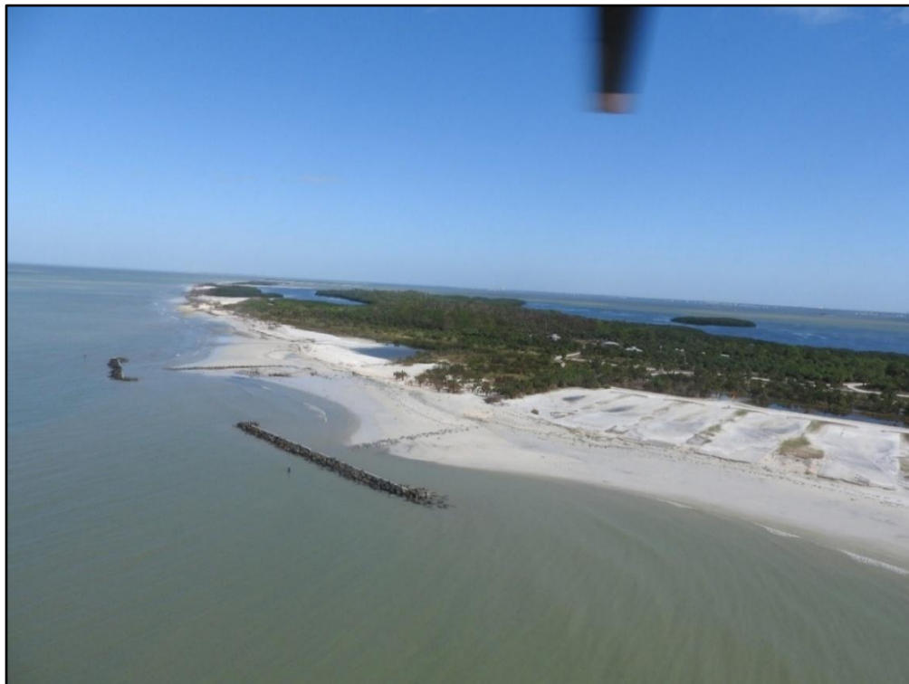
Figure 13. Major beach and dune erosion (condition IV) at Honeymoon Island State Park following Hurricanes Helene and Milton (R-8.5). Note overwash sand on the park's parking areas.
