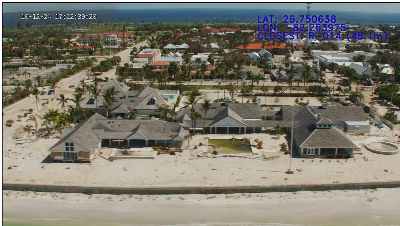
Figure 139. Major structural damage to the Gasparilla Inn Beach Club following Milton on Gasparilla Island near R-14.
