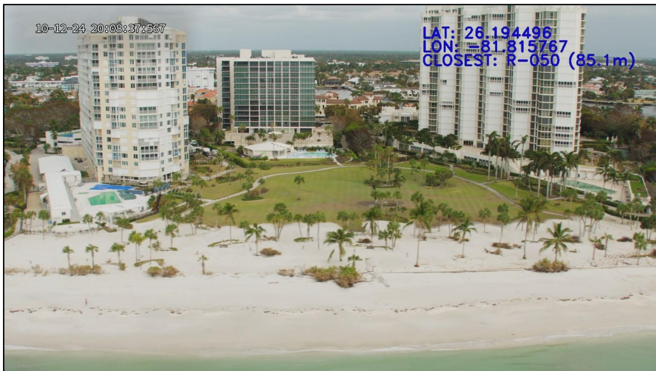
Figure 147. Major beach and dune erosion (condition IV) and storm surge overwash due to Helene and Milton at Park Shore/Naples near R-50.
