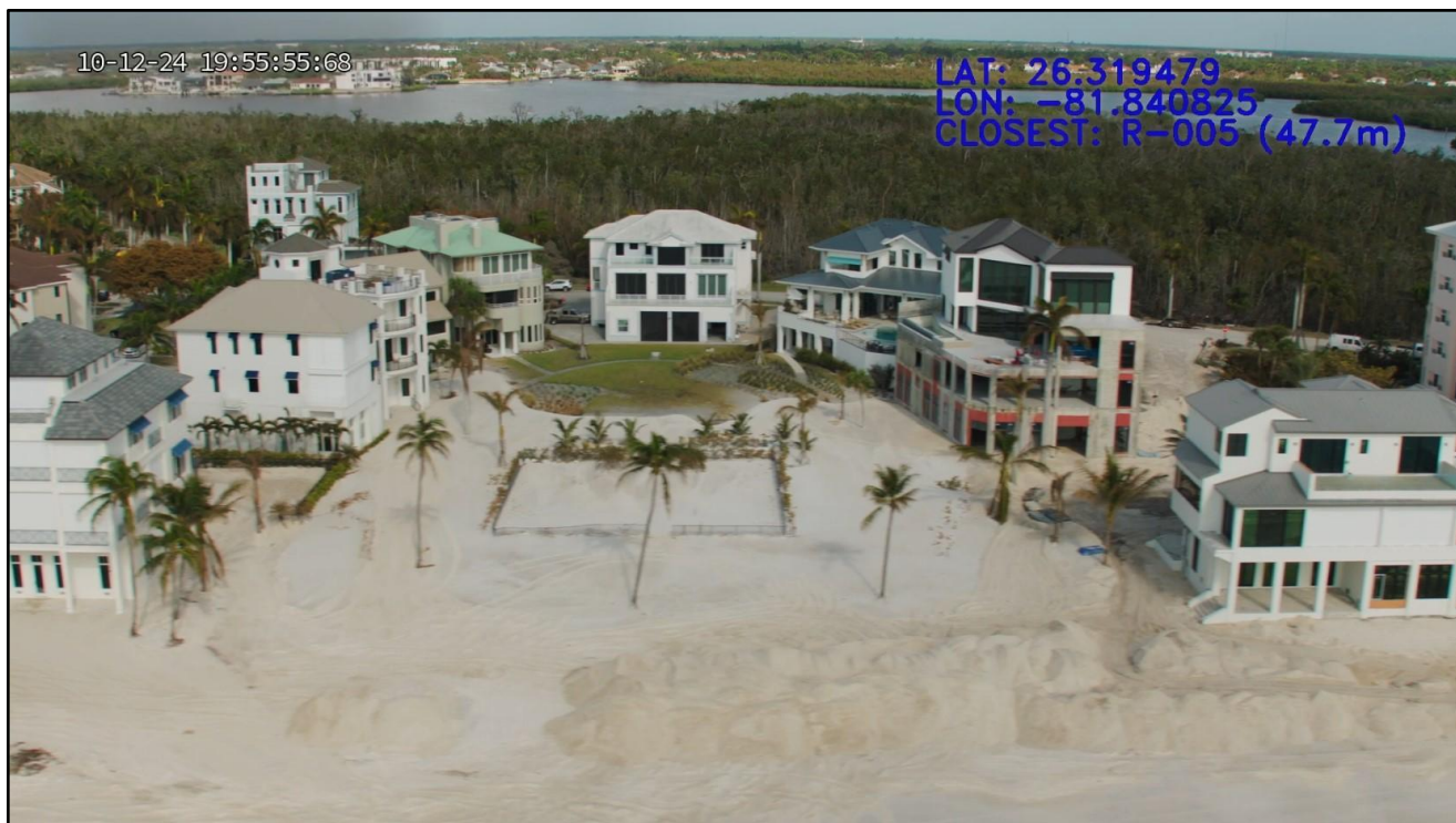
Figure 146. Major beach and dune erosion (condition IV) from Helene and Milton’s storm surge which filled the pool with overwash sand at Barefoot Beach near R-5.
