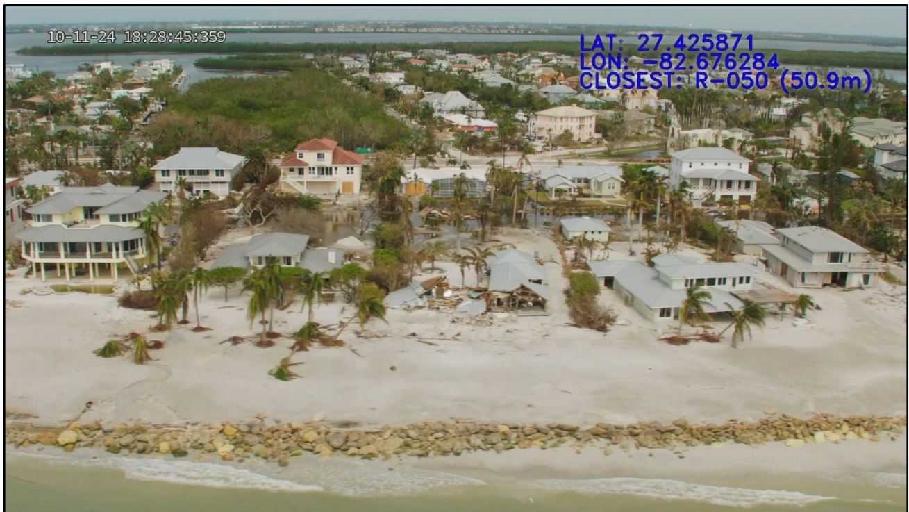
Figure 49. A single-family dwelling destroyed, armoring damage and major beach and dune erosion (condition IV) following Helene and Milton on Longboat Key near R-50.
