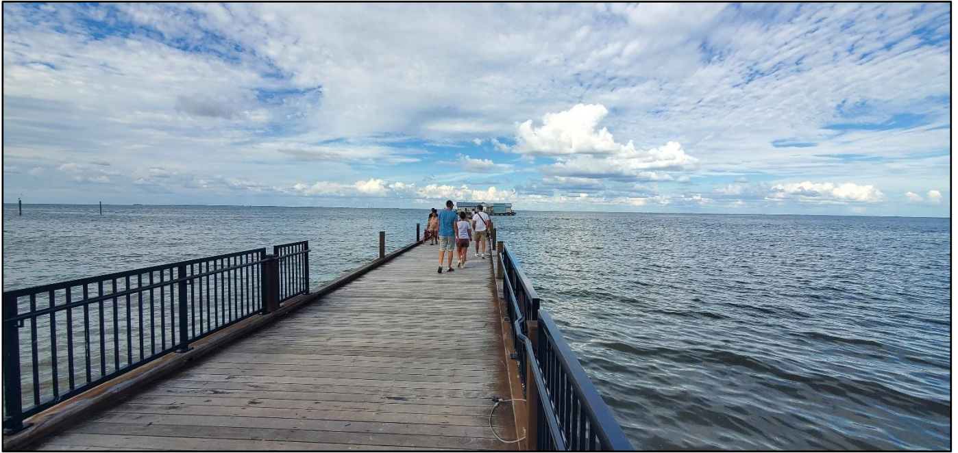
Figure 37. The Anna Maria Island City Pier was still operational after Helene along with the restaurant and bait shop at Pine Avenue.
