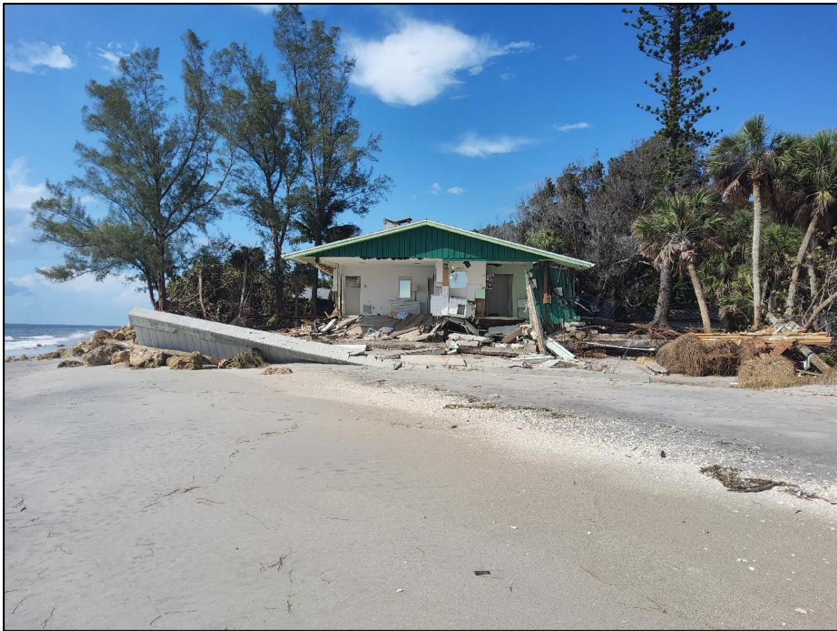
Figure 101. Single-family dwelling and seawall destroyed by Helene on Manasota Key near R-171.
