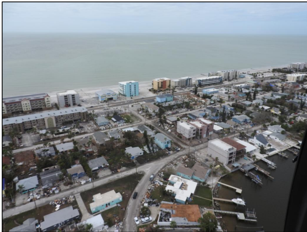
Figure 24. Back barrier damage to buildings in Madeira Beach due to Milton near R-121.
