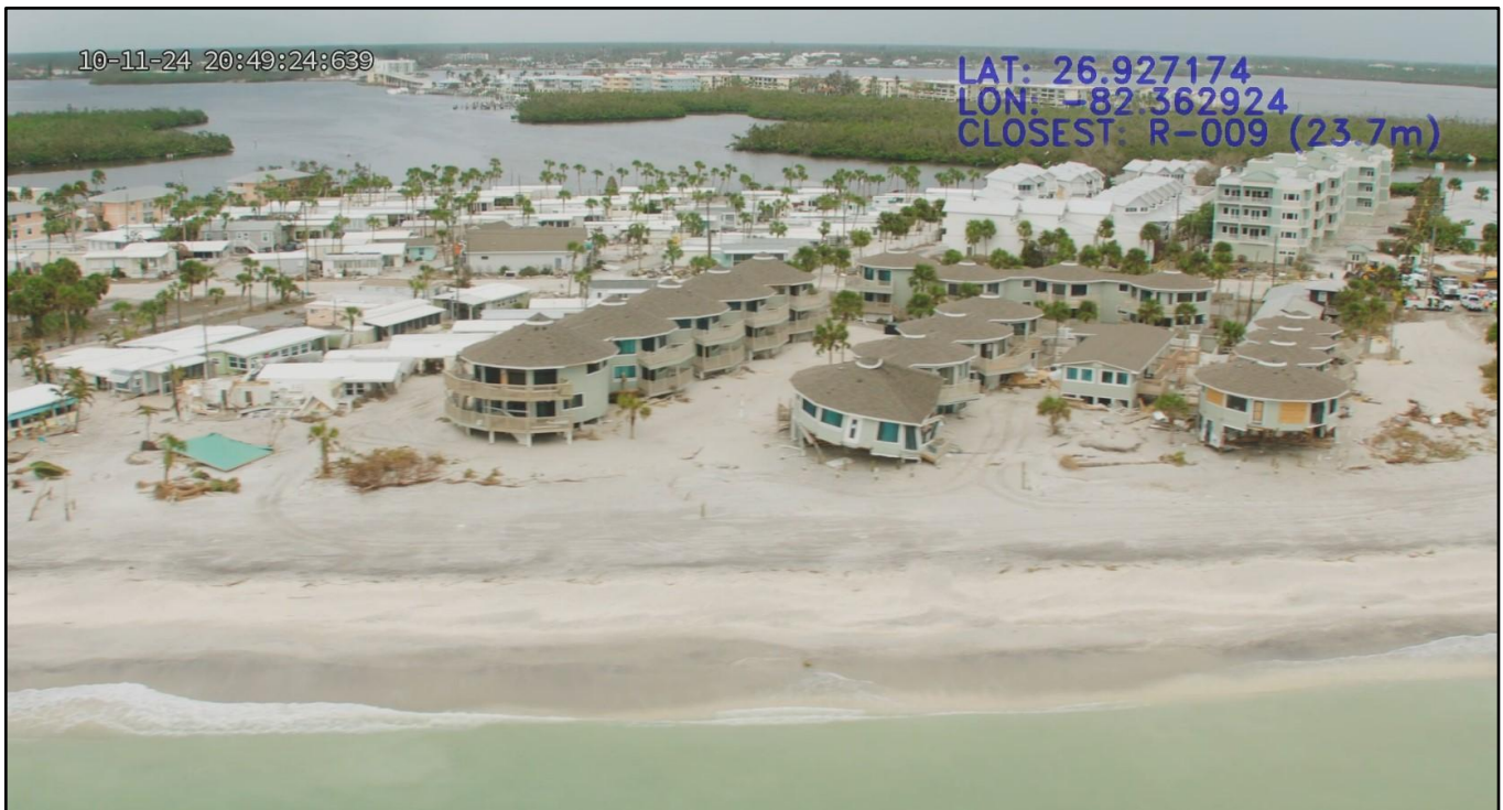
Figure 117. Multifamily dwellings with major damages due to Milton at Englewood Beach near R-9.
