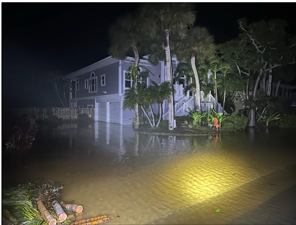
Figure 125. Helene’s storm surge flooding at R-18, typical of the island-wide flooding of 1 to 2 feet on Gasparilla Island (Photo courtesy of a Gasparilla Island resident).
