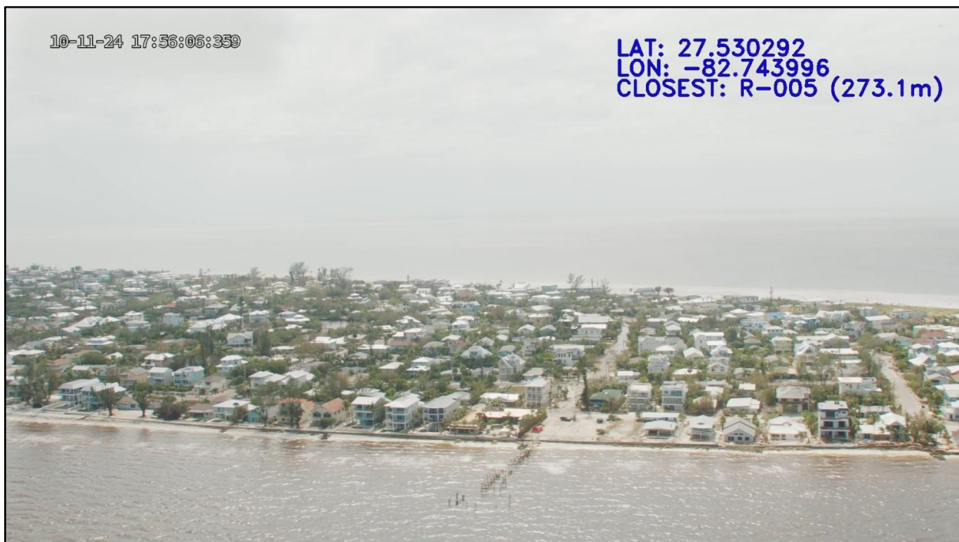
Figure 36. The northeast end of Anna Maria Island following both Hurricanes Helene and Milton showing the Rod & Reel Pier and two-story restaurant destroyed.
