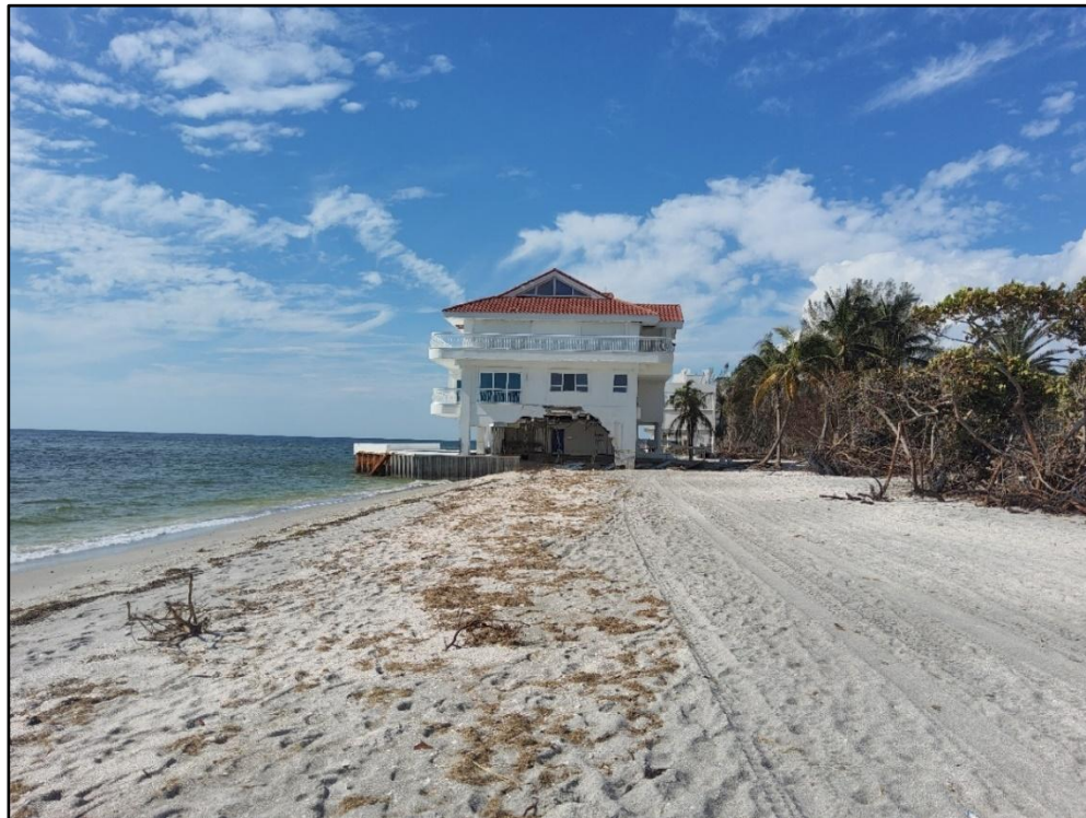
Figure 65. Single-family dwelling with ground floor damage on Siesta Key at Turtle Beach north of Midnight Pass near R-77.
