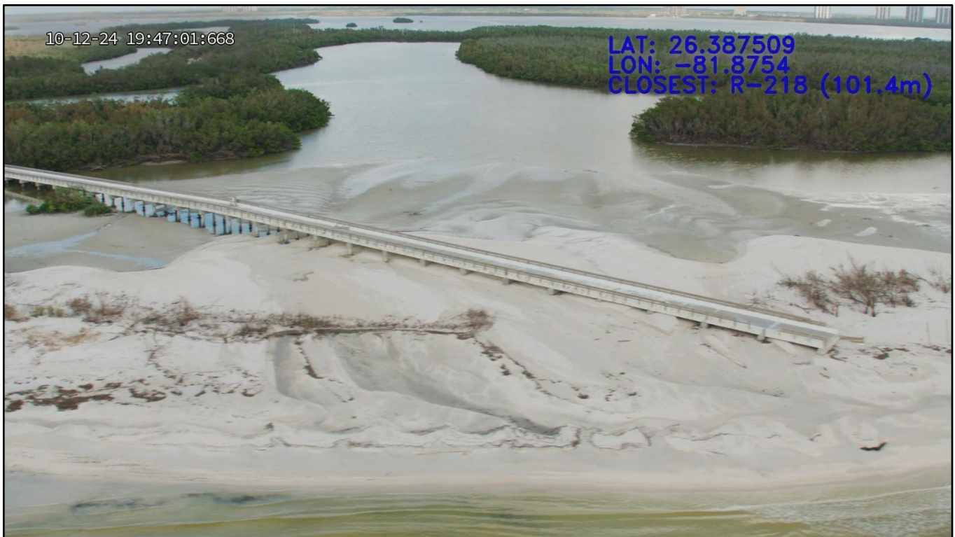
Figure 138. Major beach and dune erosion (condition IV) due to Helene and Milton at Lover’s Key State Park near R-218.
