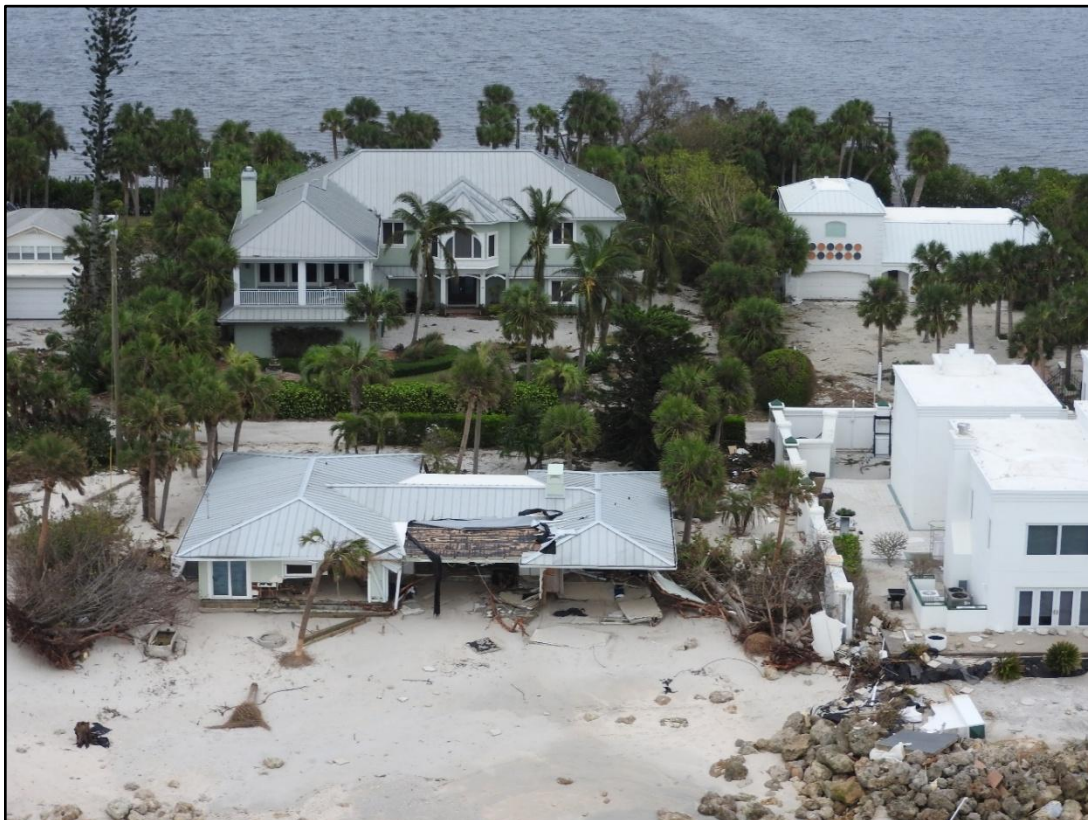
Figure 90. Single-family home substantially destroyed on Casey Key near R-87.
