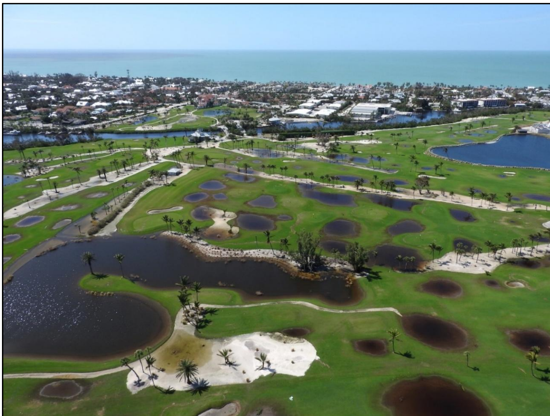
Figure 123. Water hazards on the Gasparilla Golf Club Course due to Milton near R-12.
