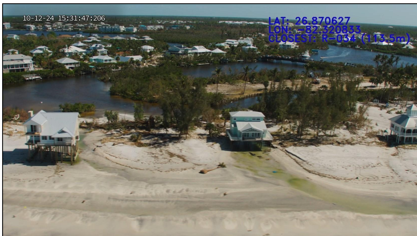
Figure 112. Storm surge discharge gullies on Don Pedro Island near R-34.
