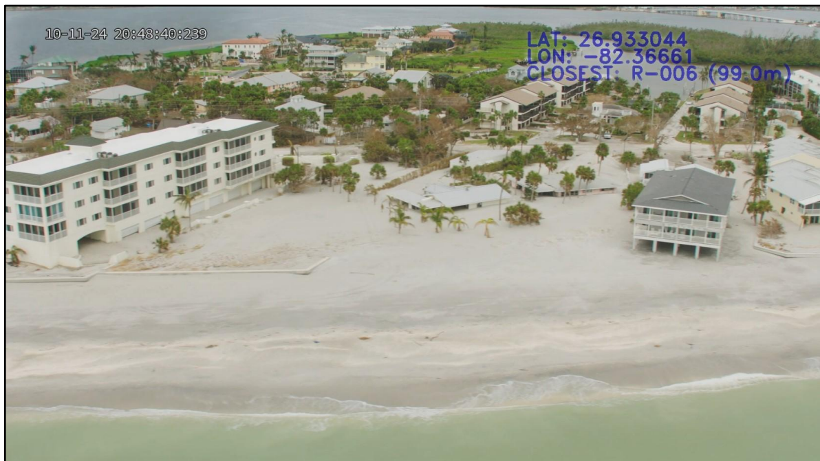
Figure 108. Major beach erosion and storm surge overwash following Milton at Englewood Beach near R-6.
