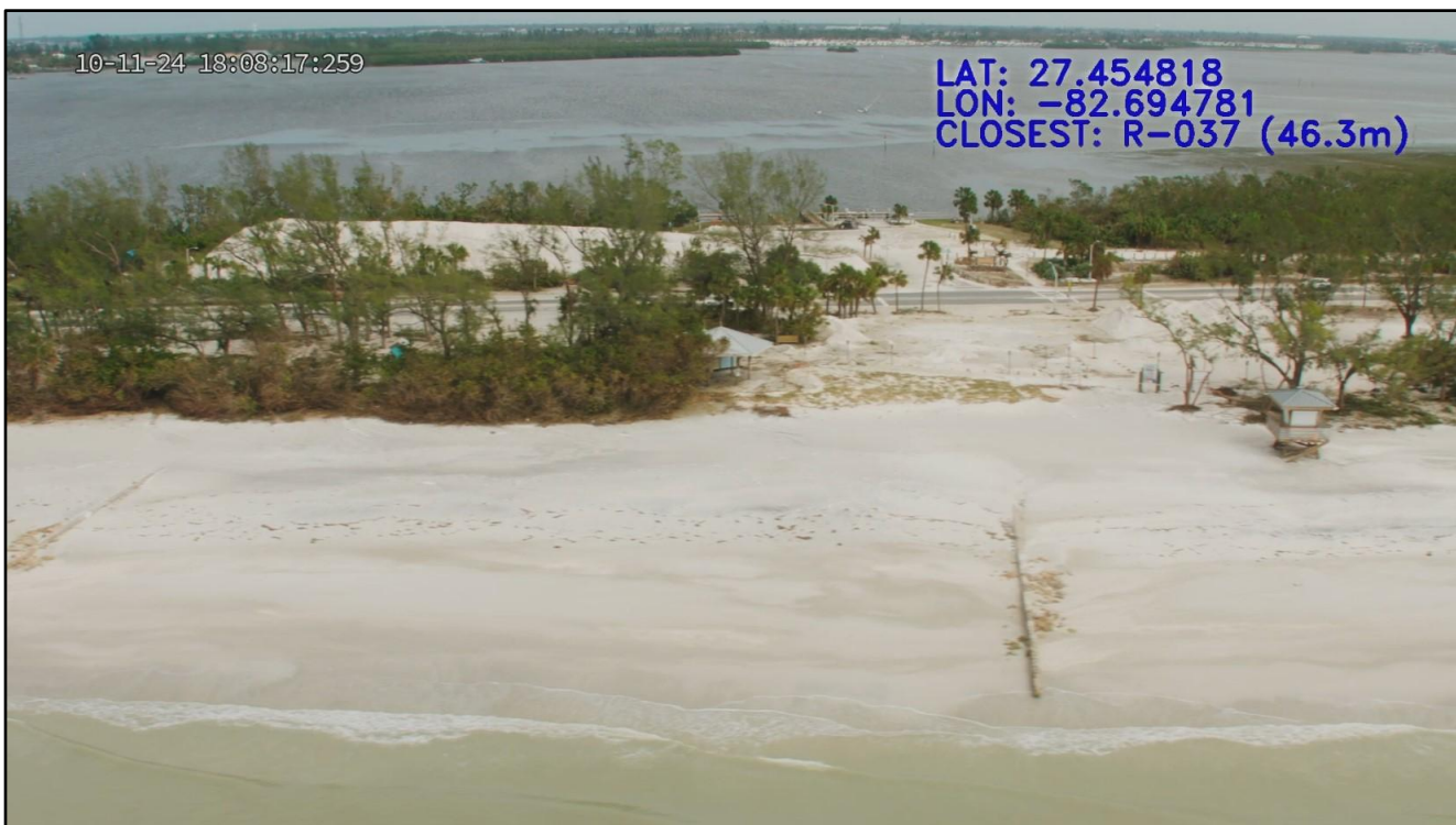
Figure 31. Major beach and dune erosion (condition IV) and stock-piled sand after Helene and Milton, at Coquina Beach, Anna Maria Island near R-37.
