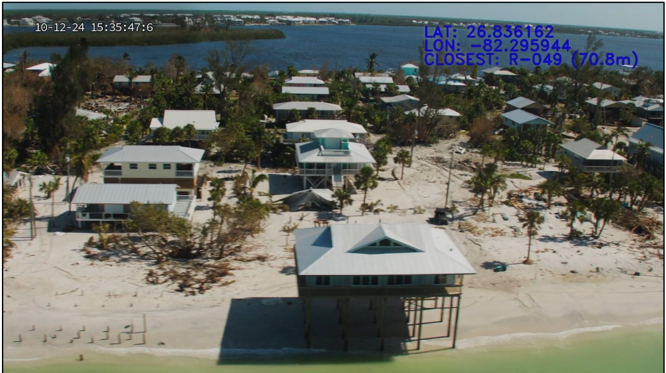
Figure 118. Single-family dwellings destroyed on Little Gasparilla Island by Milton near R-49.
