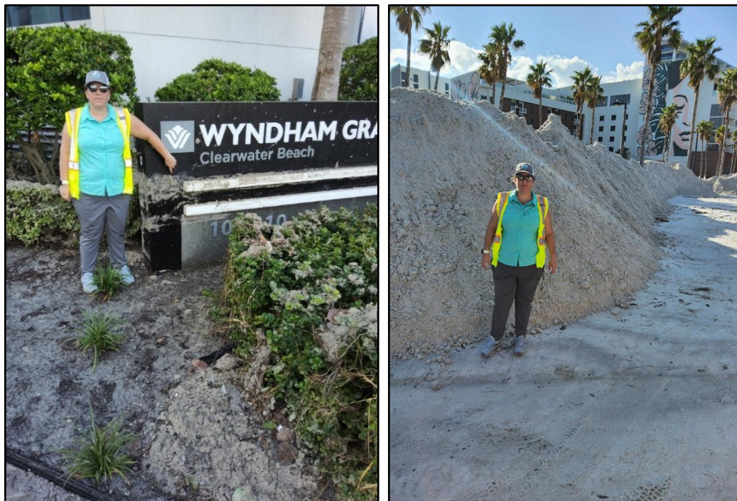
Figure 14. Flooding water mark (left) and overwash sand (right) along Gulf Boulevard following Helene’s storm surge, Clearwater Beach (R-44 to R-46).
