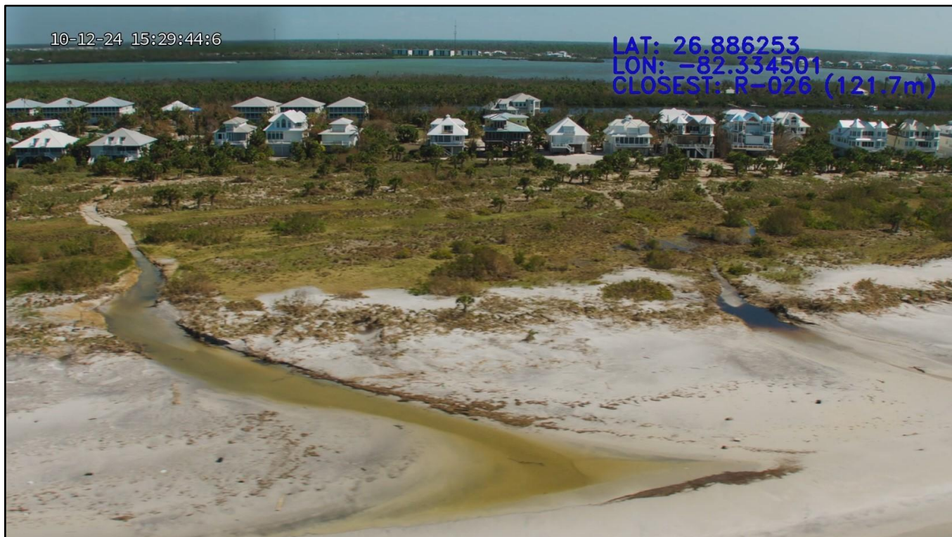
Figure 111. Storm surge discharge gullies at the Palm Island development on Don Pedro Island (R-26).
