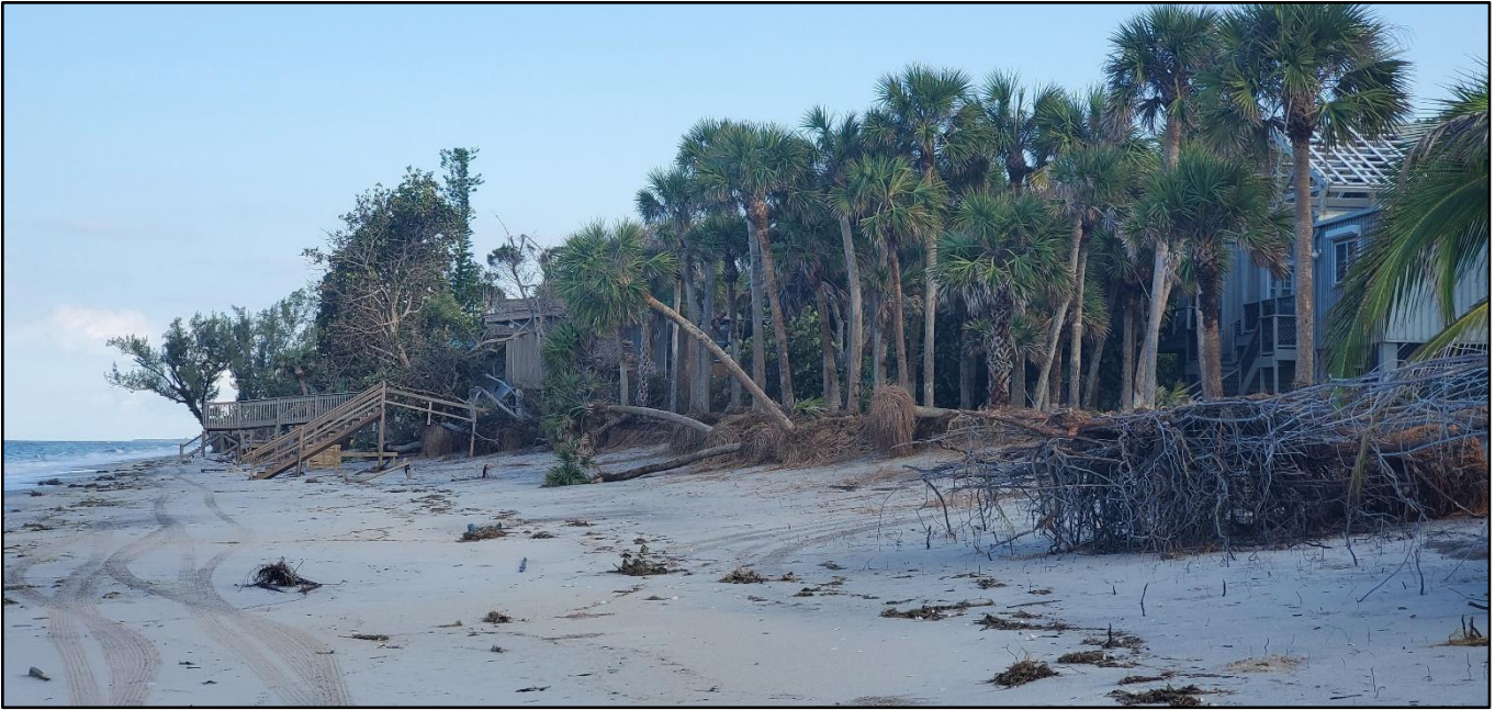
Figure 76. Major beach and dune erosion (condition IV) due to Helene on Manasota Key near R-173.
