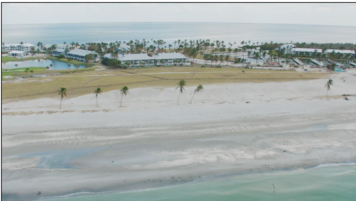
Figure 132. Major beach and dune erosion (condition IV) due to Helene and Milton at South Seas Plantation on Captiva Island near R-85.
