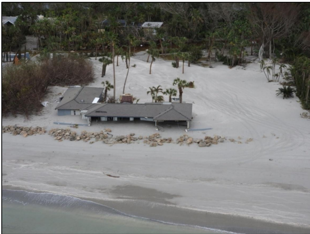
Figure 84. Major structural damage to single-family dwelling due to the storm surges of Helene and Milton on Siesta Key near R-67.
