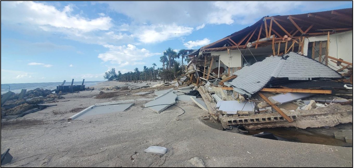
Figure 103. Single-family dwelling destroyed by Helene on Manasota Key near R-172.
