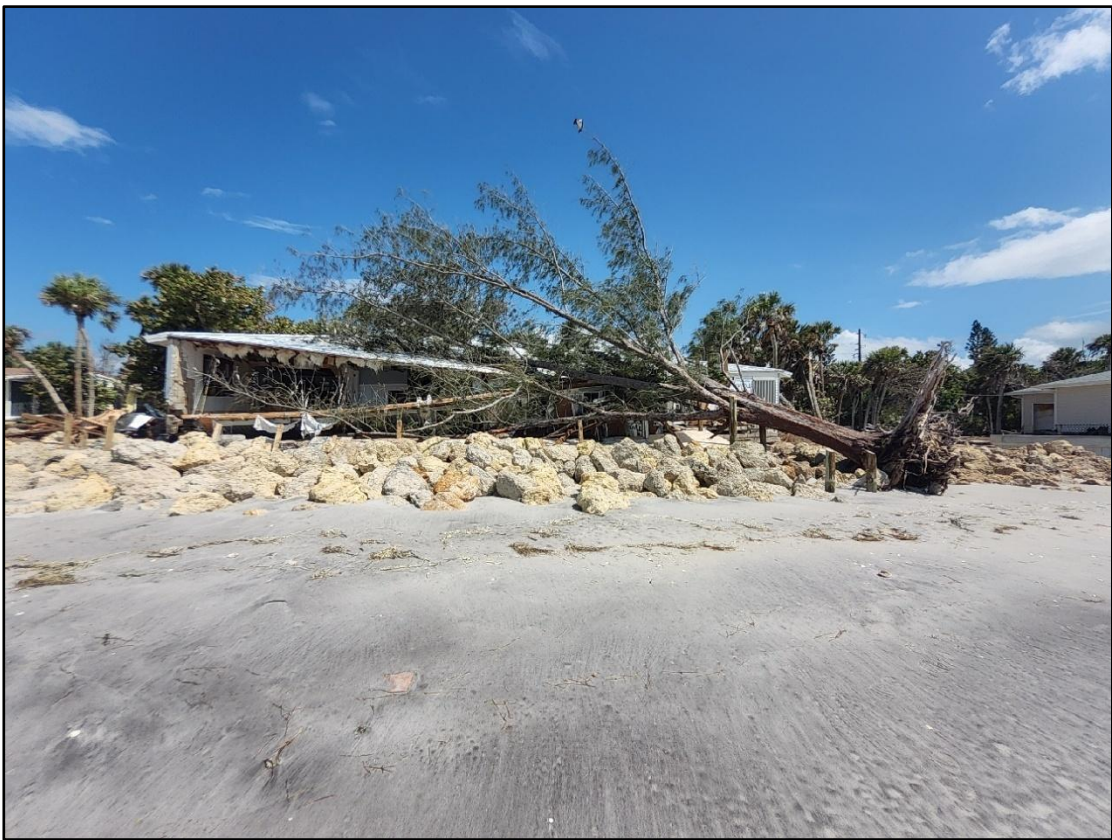
Figure 104. Single-family dwelling destroyed by Helene on Manasota Key near R-173.
