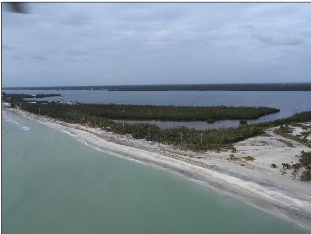
Figure 79. Major beach and dune erosion (condition IV) and major road damage at Blind Pass County Park near R-176.
