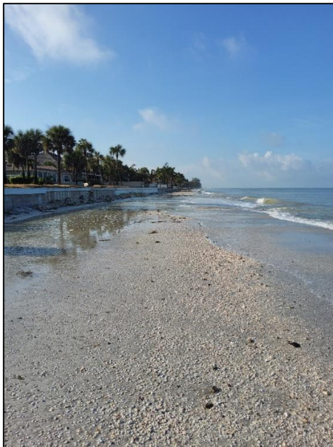
Figure 15. Major beach erosion (condition IV) along Belleair Beach due to Helene (R-66 to R-67).
