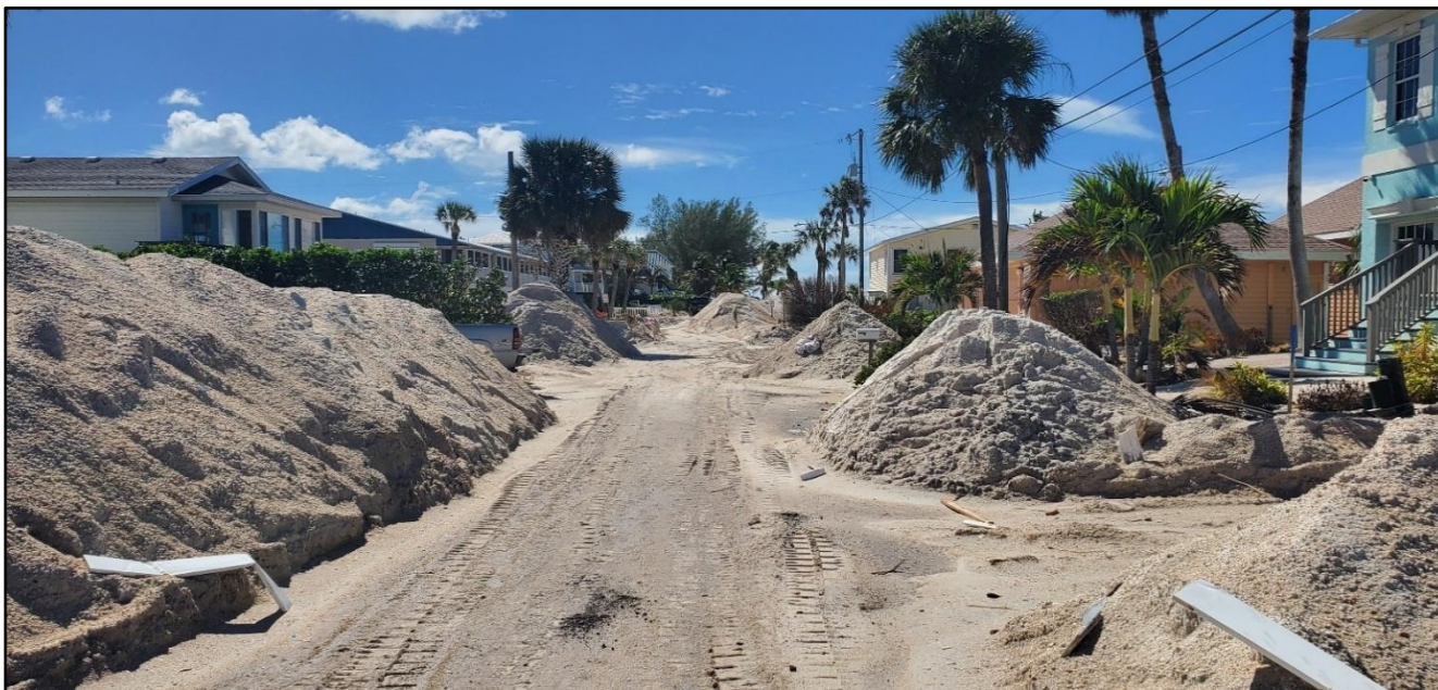
Figure 30. Beach sand piled up on either side of roadway following road scraping of Helene’s overwash deposits on Anna Maria Island.
