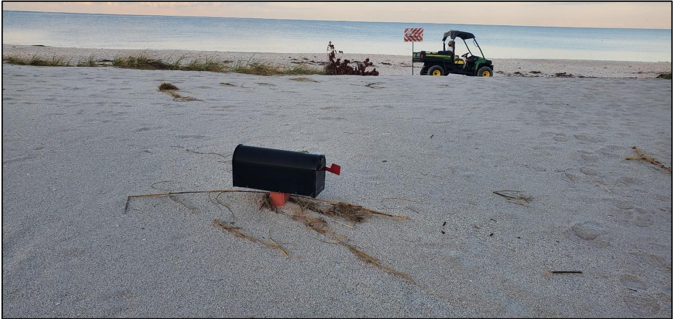
Figure 74. Mailbox post buried Helene’s overwash at Venice Beach near R-130.
