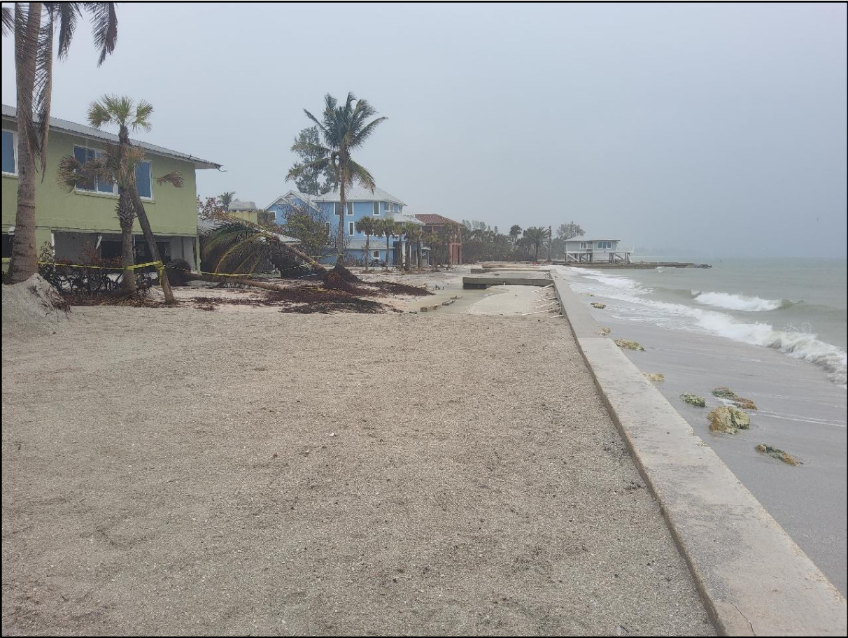
Figure 32. Major beach erosion (condition IV) due to Helene on northern Longboat Key near R-48.
