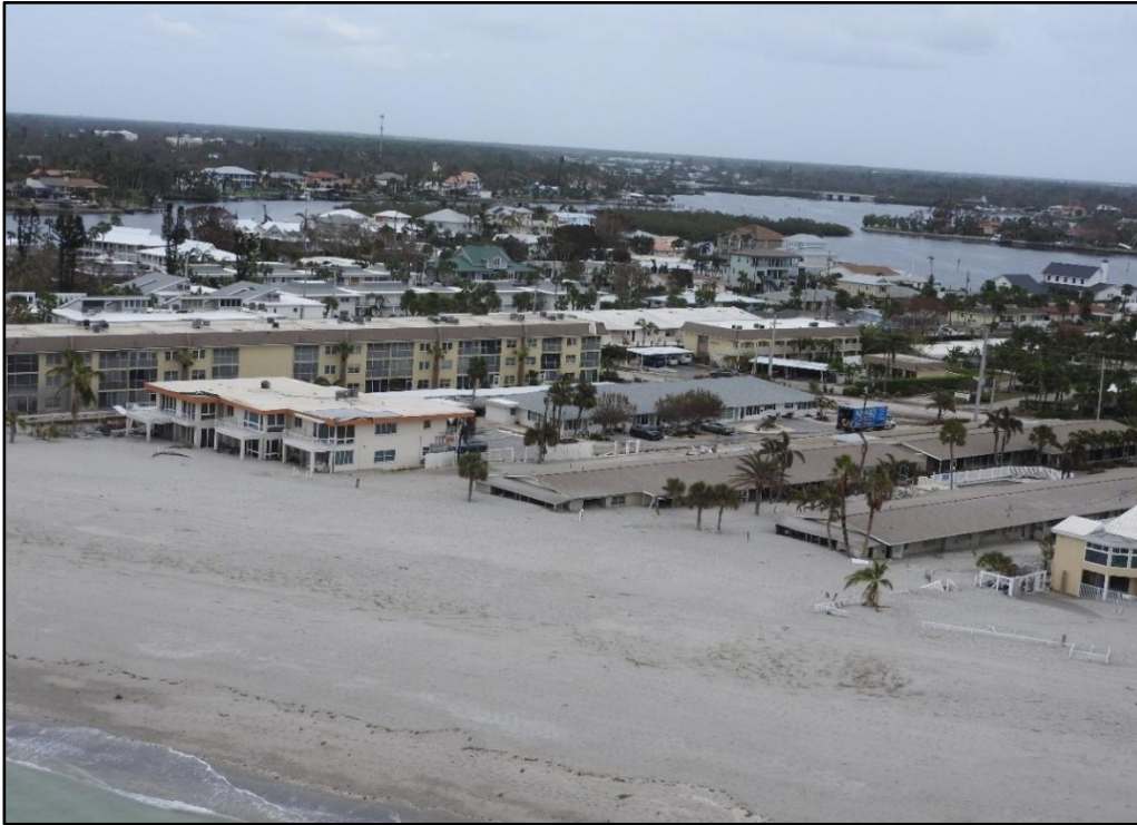
Figure 72. Major beach and dune erosion (condition IV) and storm surge overwash following Helene and Milton on Venice Beach near R-117.
