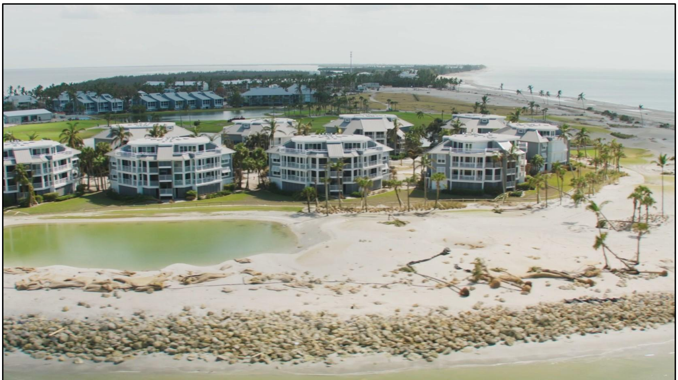
Figure 141. Rock revetment damage at South Seas Plantation at Redfish Pass on Captiva Island near R-84.
