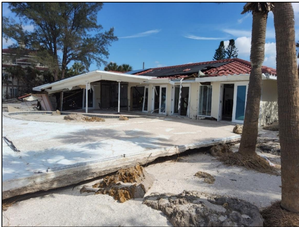
Figure 92. Single-family dwelling destroyed and a pool filled with sand by Helene on Casey Key near R-91.
