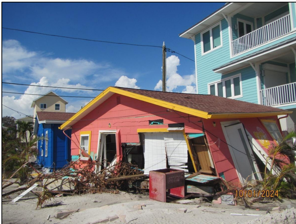
Figure 21. Damage to single family dwelling on Treasure Island due to Hurricane Helene near R-141.
