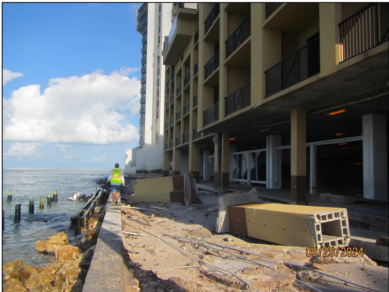
Figure 20. Coastal armoring damage at Clearwater Pass due to Hurricane Helene near R-47.
