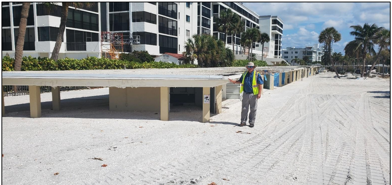
Figure 57. Major damage to a Lido Key hotel from Helene's storm surge and overwash deposit of approximately three to four feet of beach sand near R-40.
