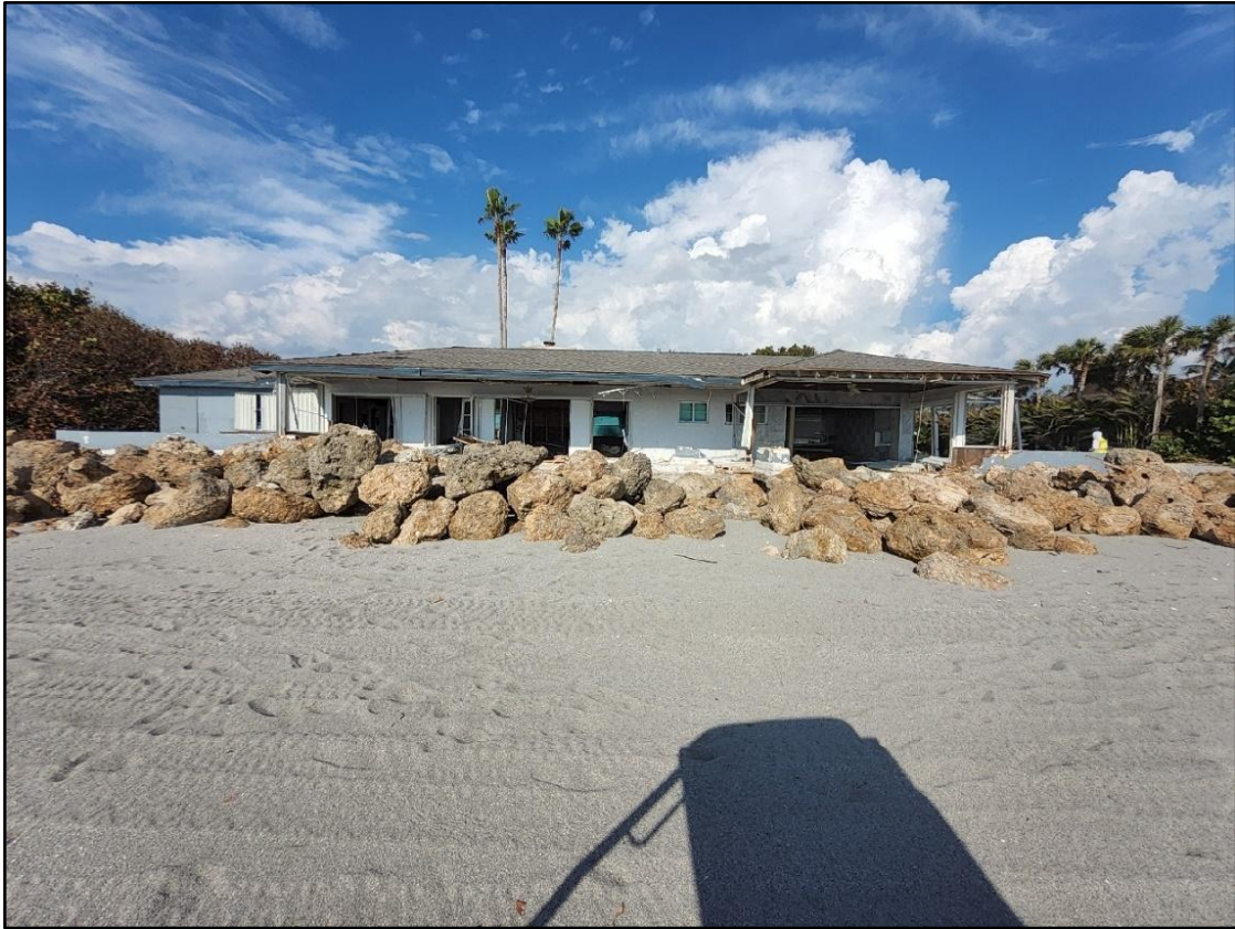
Figure 85. Major damage to rock revetment (level III) and to single-family dwelling on Siesta Key near R-67.
