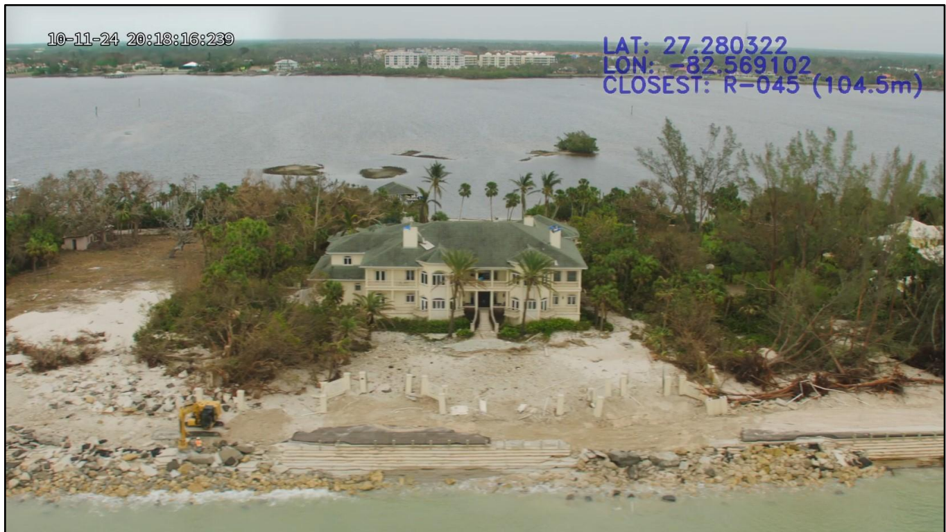
Figure 89. Major road and revetment damages from Helene’s storm surge on Casey Key near R-85.
