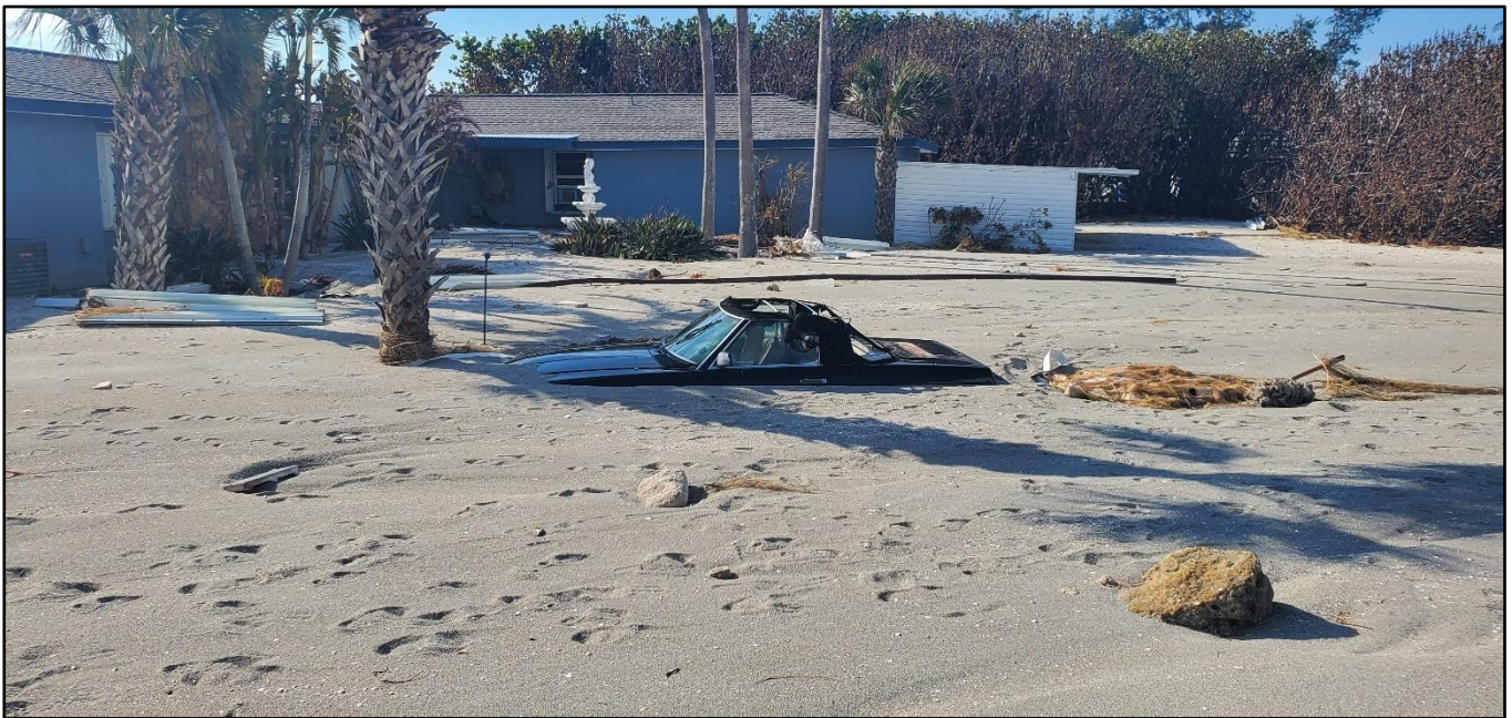
Figure 63. Storm surge damages to home and yard from Helene and Milton on Siesta Key near R-67. Note: Mercedes convertible buried in 3 to 4 feet of overwash sand.
