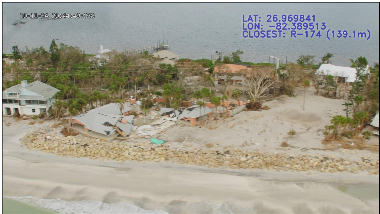
Figure 105. Single-family dwelling destroyed and major revetment damage by Milton on Manasota Key, R-173.
