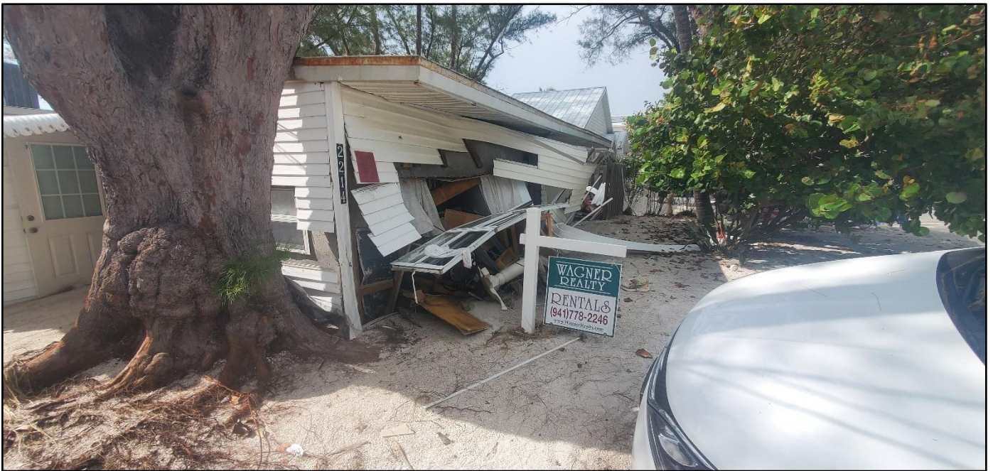
Figure 42. A single-family dwelling on Anna Maria Island with major first floor damage from Helene's storm surge near 23 rd Street North at R-28.
