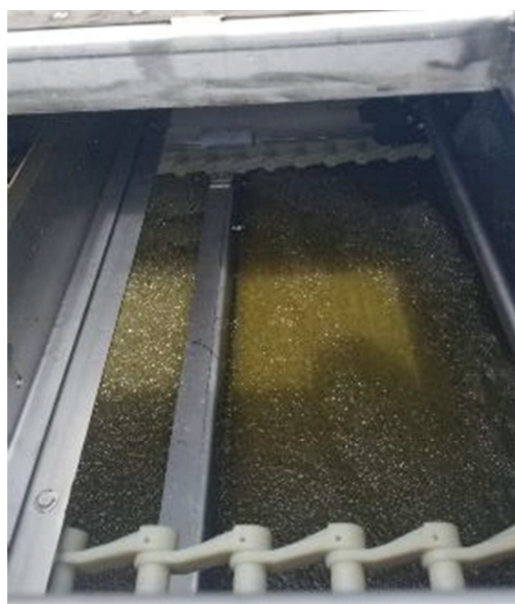
Flotation chamber showing float blanket skim bar.
