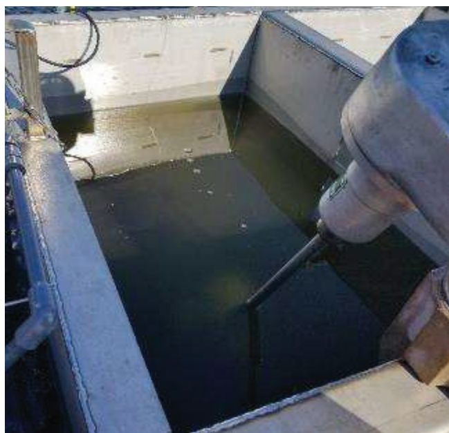
Coagulant chamber showing mixer.
