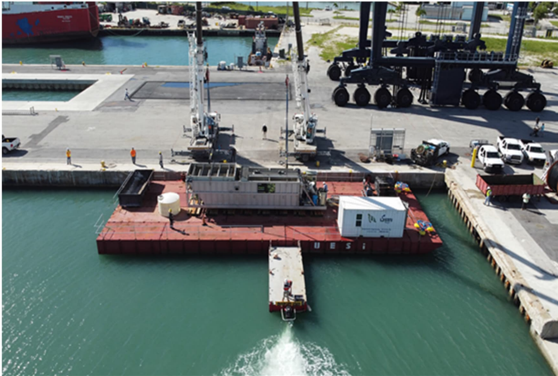
Algae harvester and ancillary equipment loaded onto the barge at Derecktor Shipyards, Fort Pierce, FL
