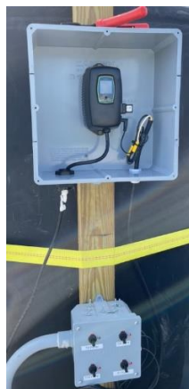
Figure 8. UV control and power control and indicator enclosure.
