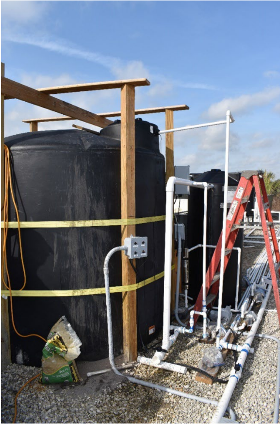
Figure 15. Sand filter (3/23/22)
