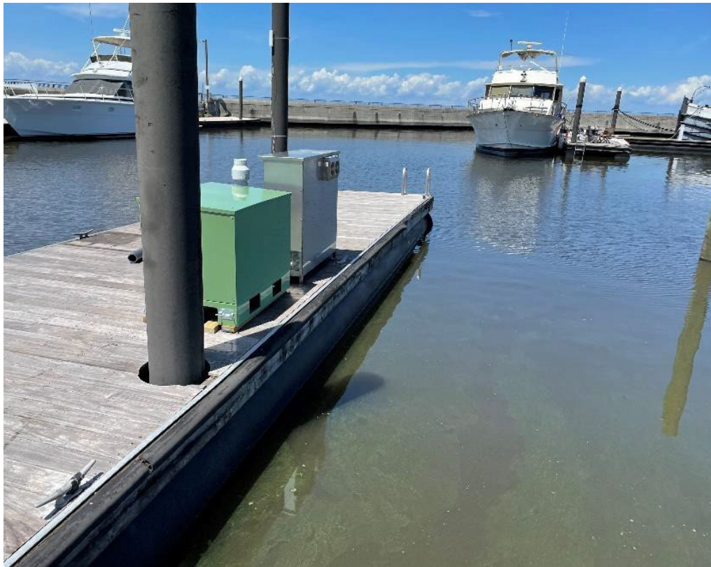
Figure 4: Photo of nanobubble generator located at dock space B14.
