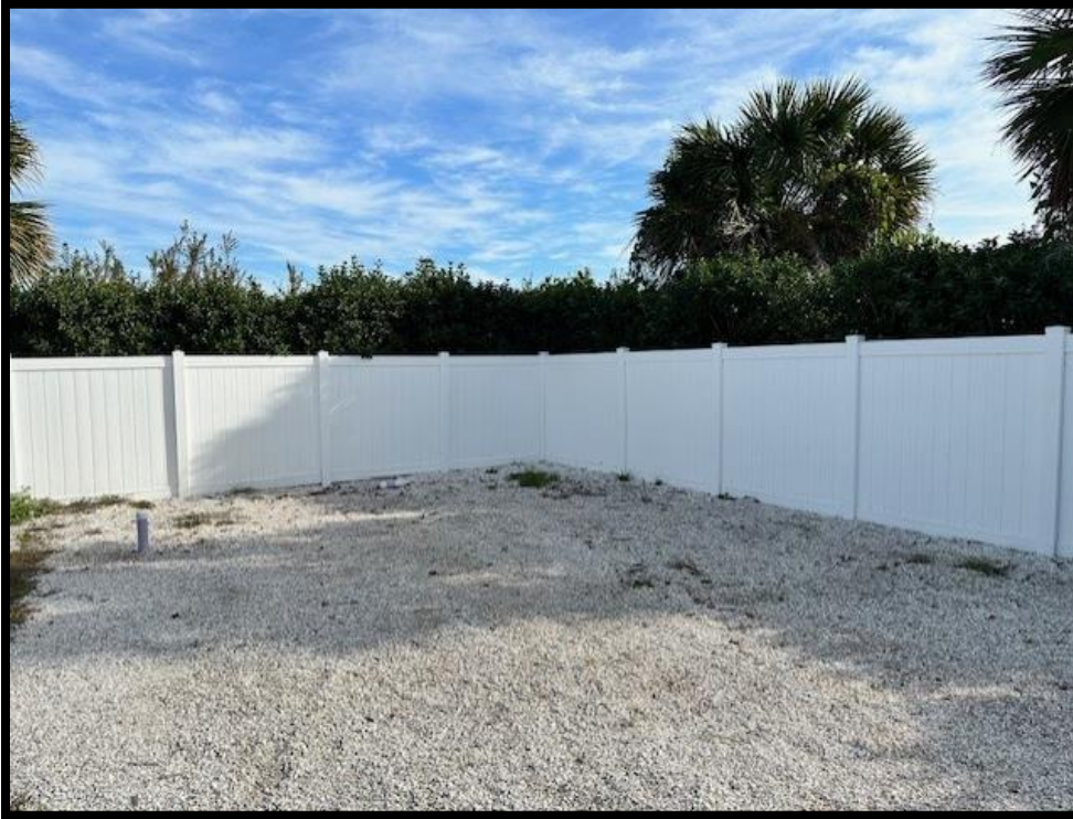
Figure 18. Site restored with plumbing capped (Task 5 – Demobilization).
