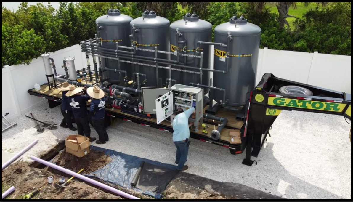
Figure 14. Aerial image of Vessels being installed (Task 3 – Start up).
