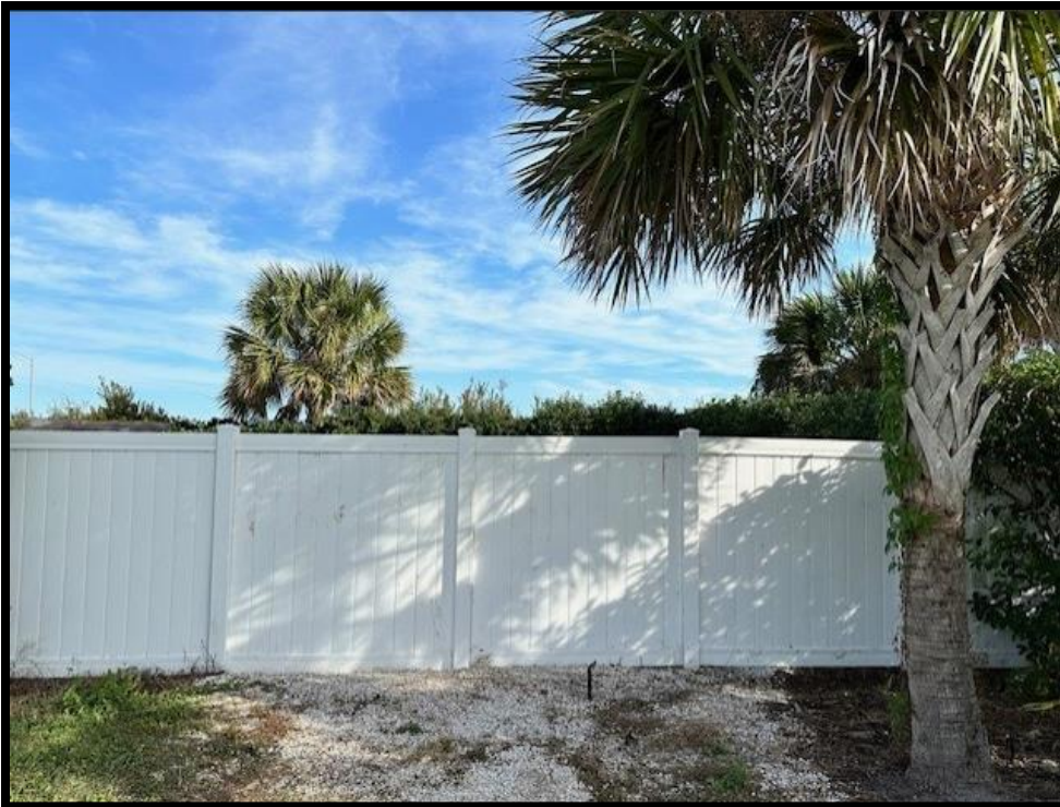
Figure 19. Fencing reinstated surrounding site (Task 5 – Demobilization).
