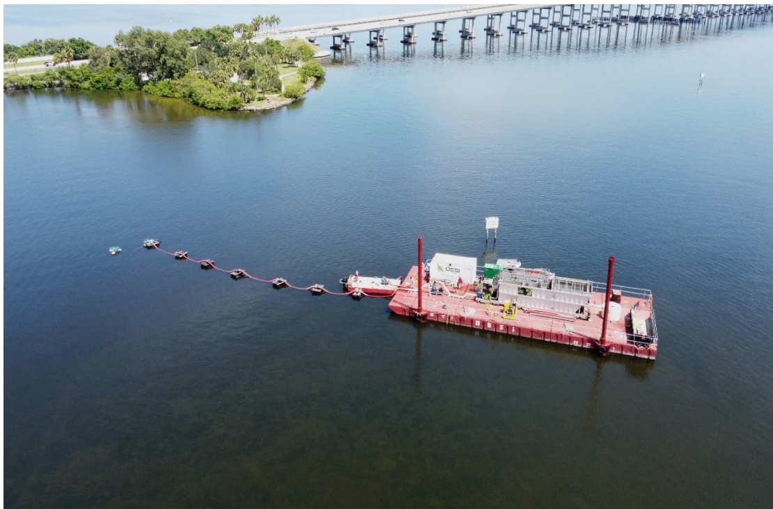
Fully assembled algae harvesting system at Barge Station 1, Melbourne, FL.
