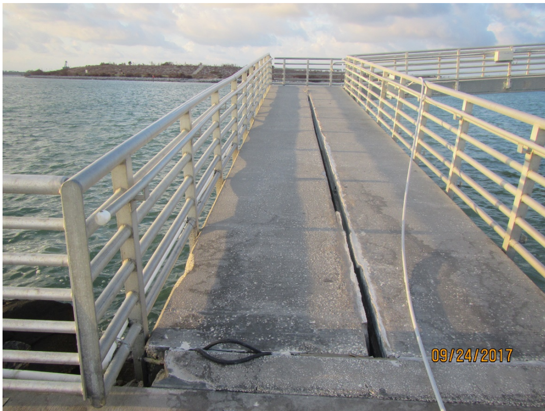
Figure 35. Jetty Park fishing pier damage where concrete deck slabs were separated, R1.
