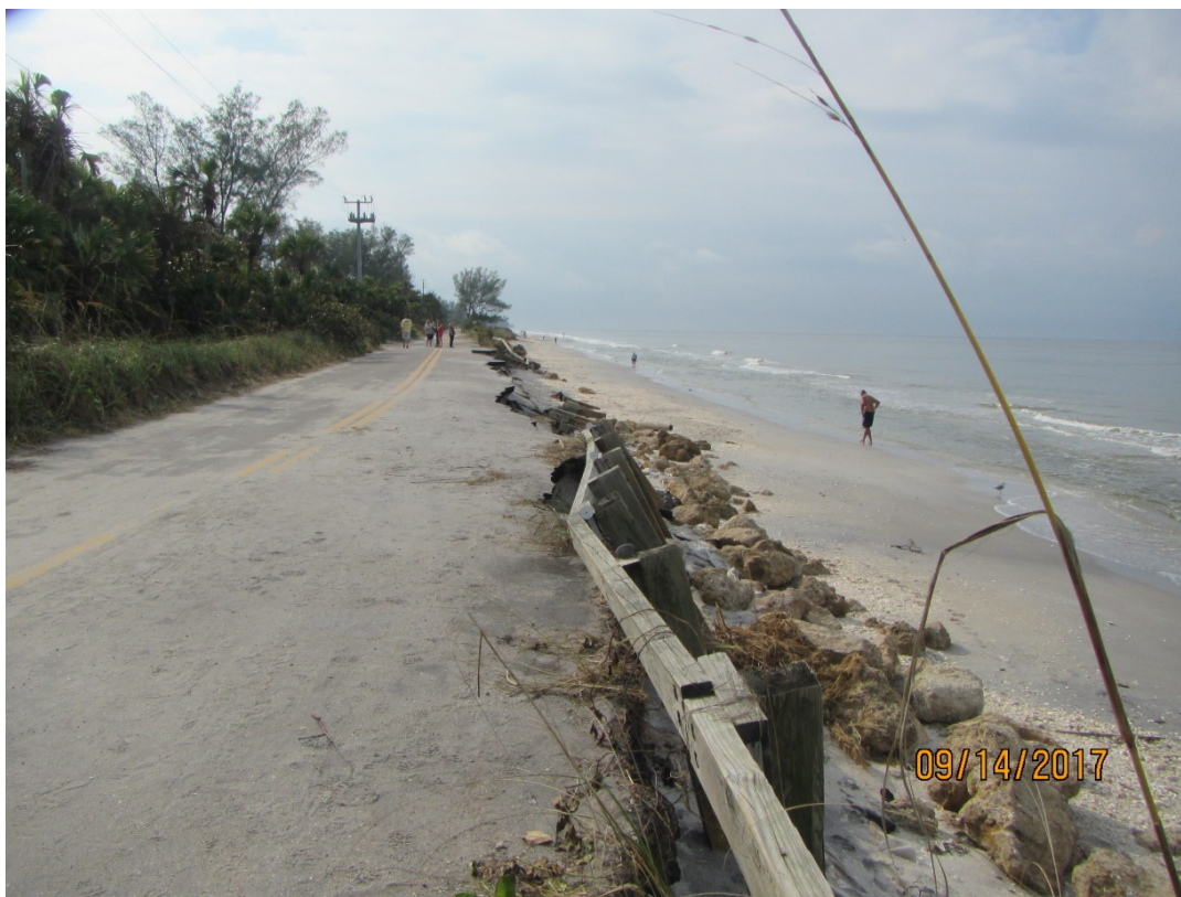
Figure 55. Dune erosion that damaged Manasota Key Road near R175.
