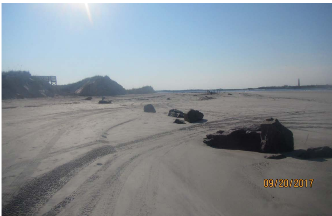
Figure 26. South jetty breach and overwash into Ponce de Leon Inlet (looking northwest), R149.
