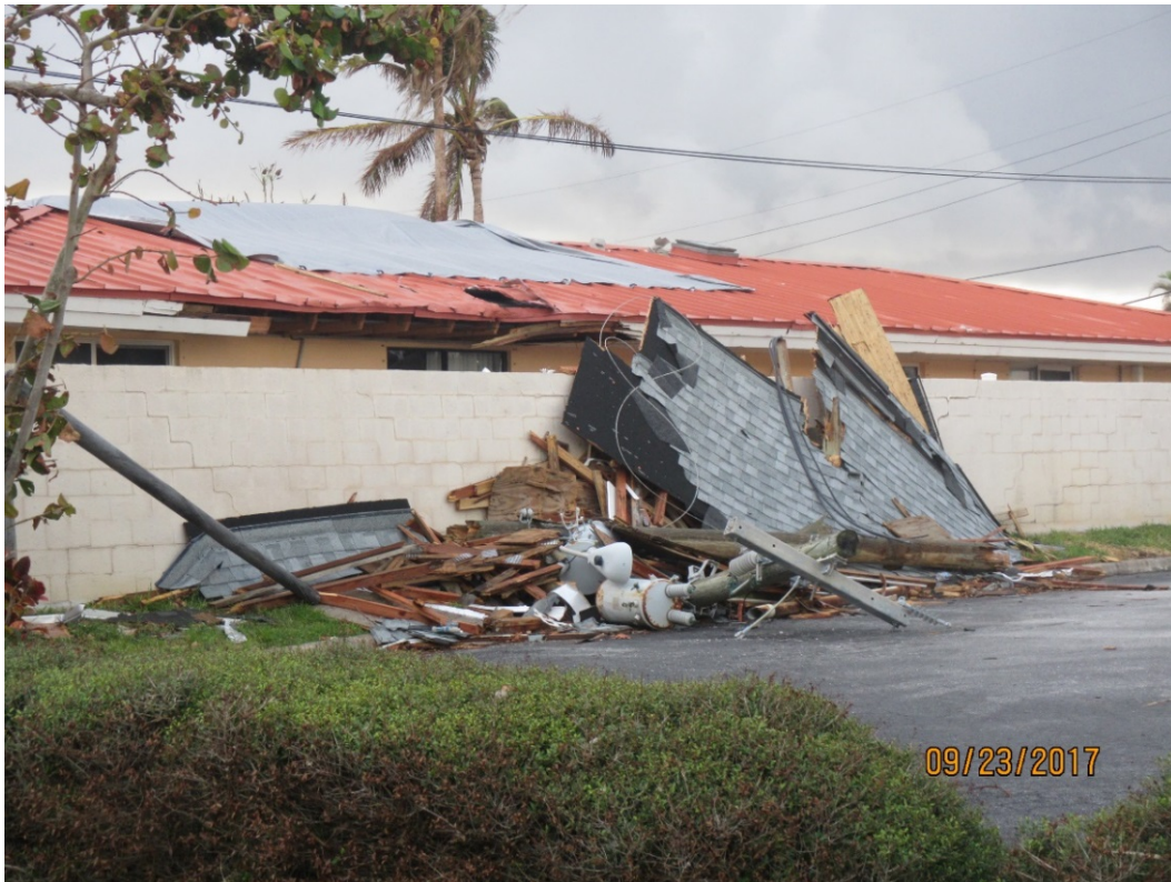
Figure 33. Condominium roof section blown across State Road A1A onto single-family dwelling by tornado at R122, Indialantic.
