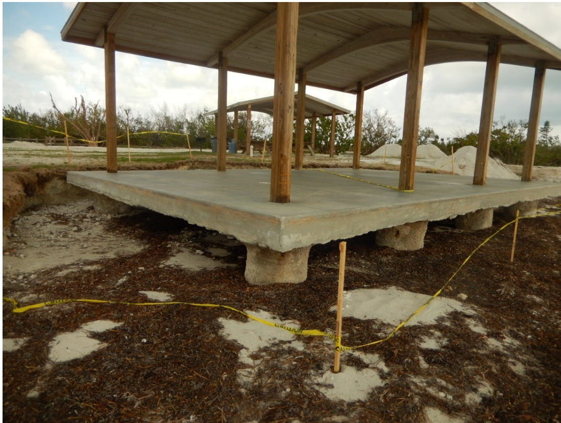
Figure 66. Undermined pavilion at Curry Hammock State Park.
