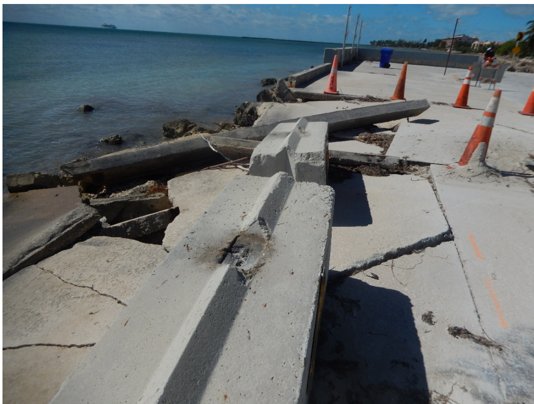
Figure 97. Bertha Street end seawall damage, Key West.
