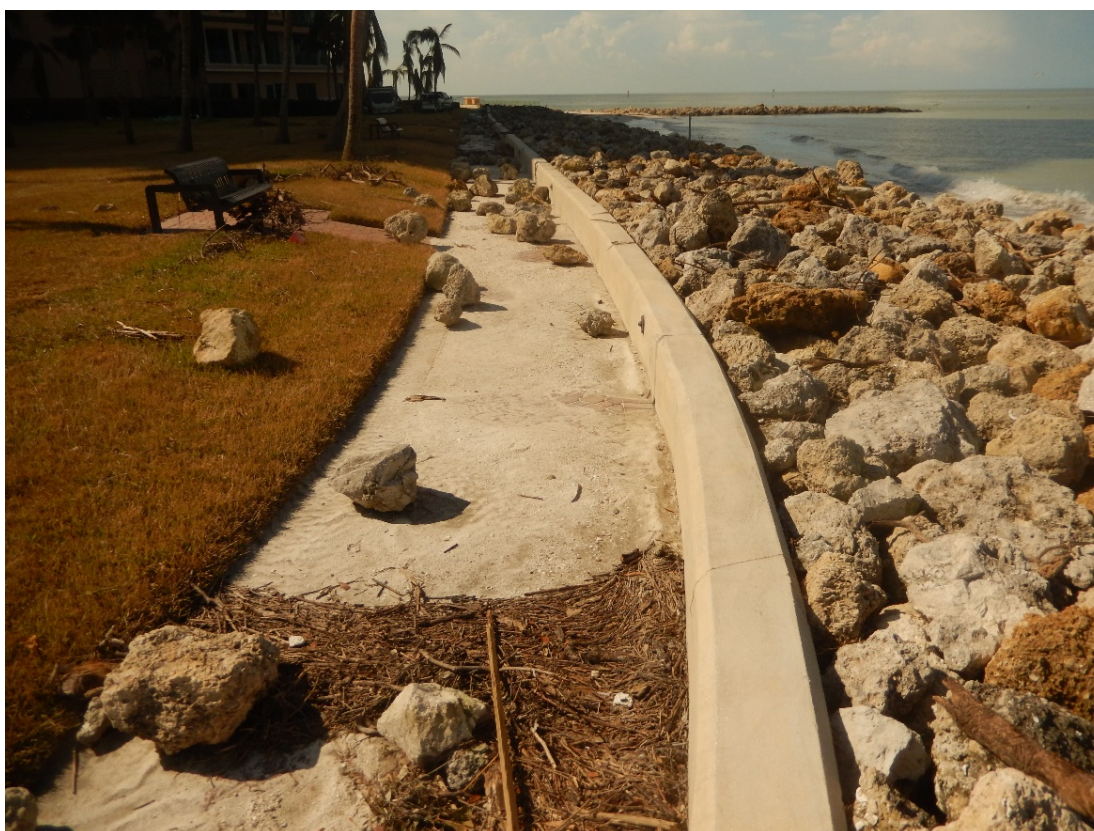
Figure 41. South Marco Island revetment damage near R148.
