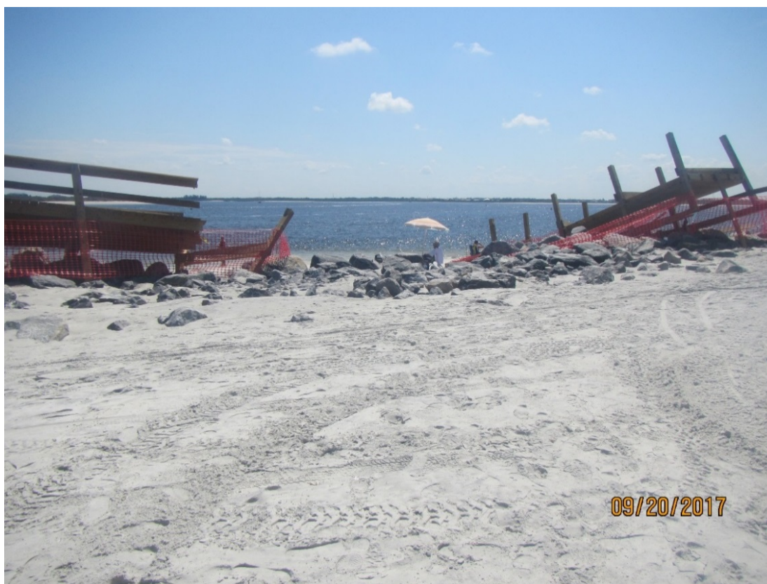
Figure 28. Major damage to north jetty and boardwalk at Ponce de Leon Inlet, R148.
