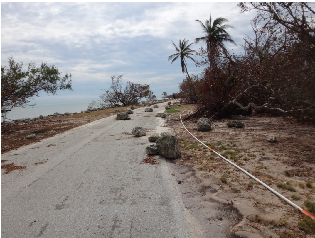
Figure 63. The park road in Long Key State Park with overwash of revetment boulders.
