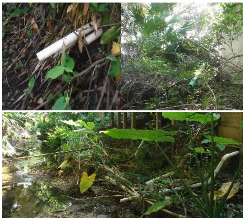
Figure 20. Illicit connections to Poinciana ditch
