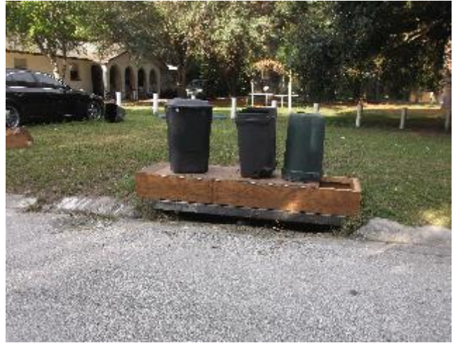
Figure 19. Leaky trash cans stored on top of storm drain.
