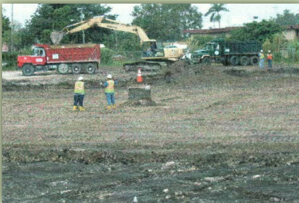
Soil and ash removal
