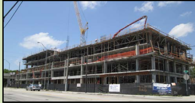
Site construction (May 2014)
