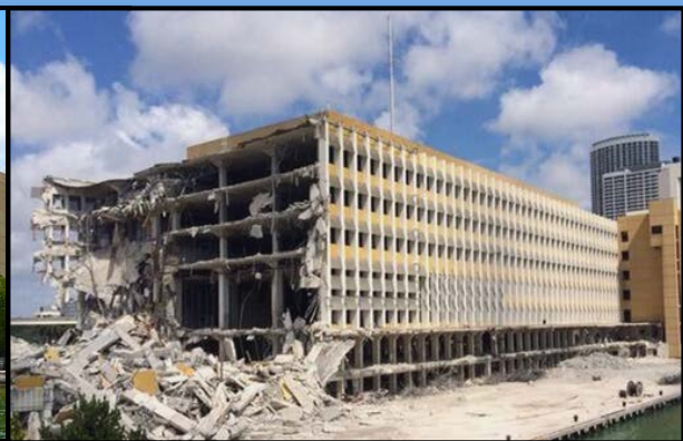
Demolition of Miami Herald Building (2014)
