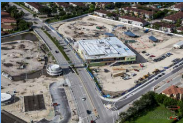
Site development - September 2016
