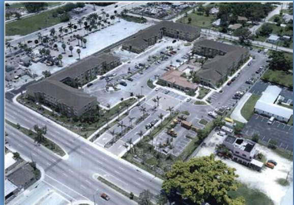
The Corinthian completed (June 8, 2007)
