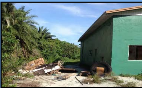
Dumping near former maintenance building
