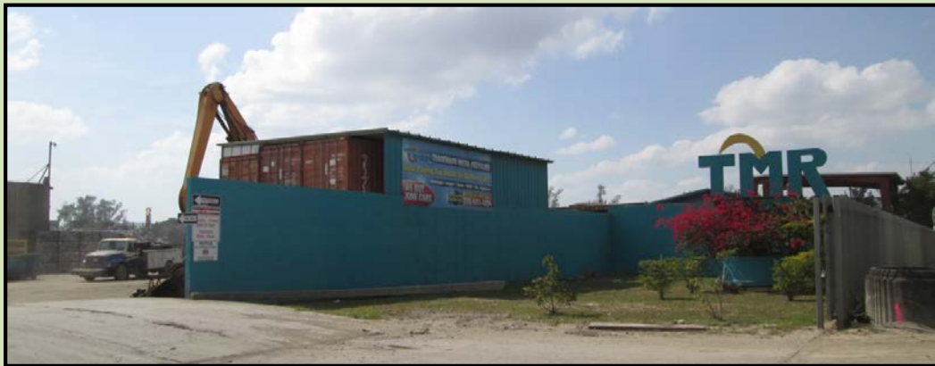
Trademark Metals Recycling Facility
