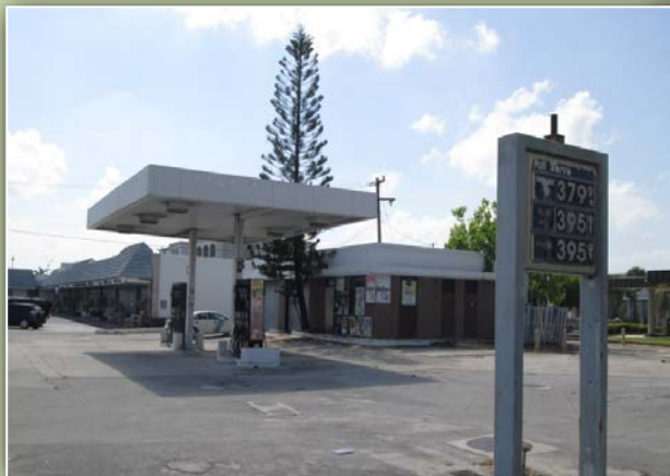
Out of service gas station (2014)
