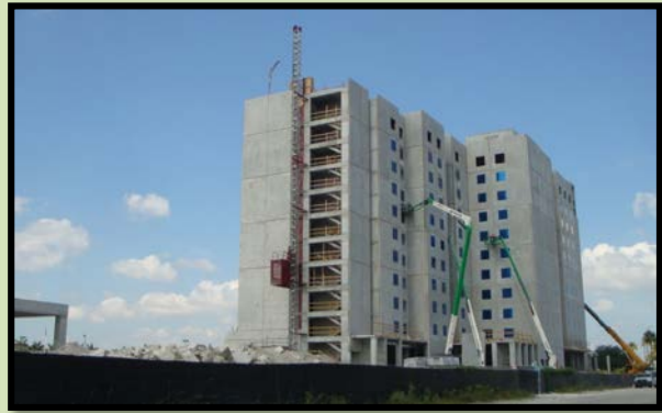
Adjacent building construction (2015)
