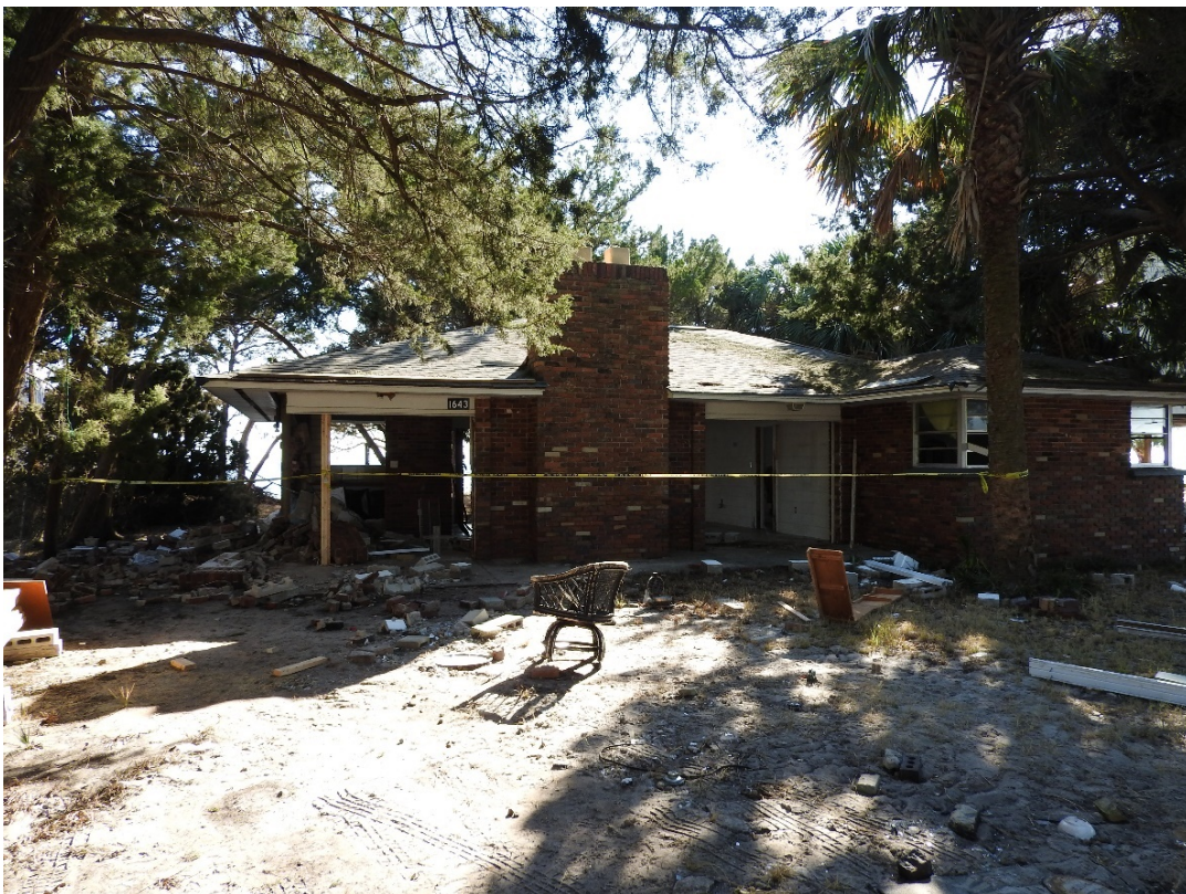
Figure 95. Dwelling with major damage from the storm surge at Shell Point, V342.
