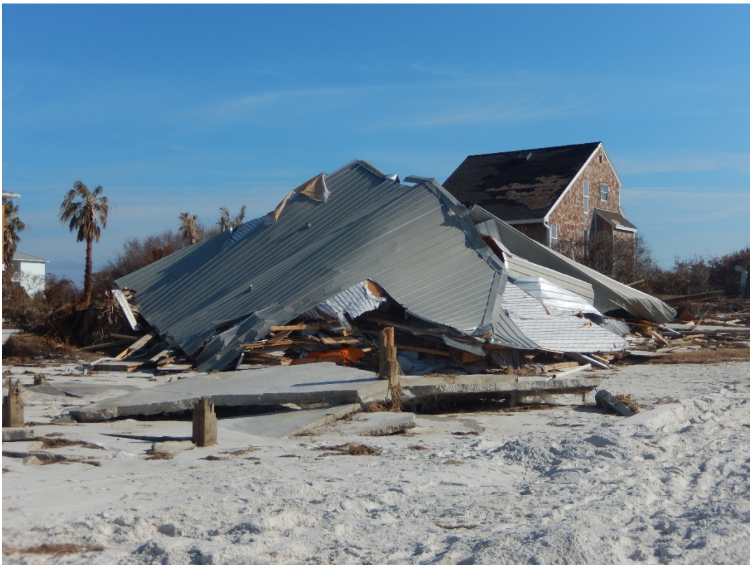
Figure 60. Dwelling destroyed near R99.5, St. Joseph Peninsula.
