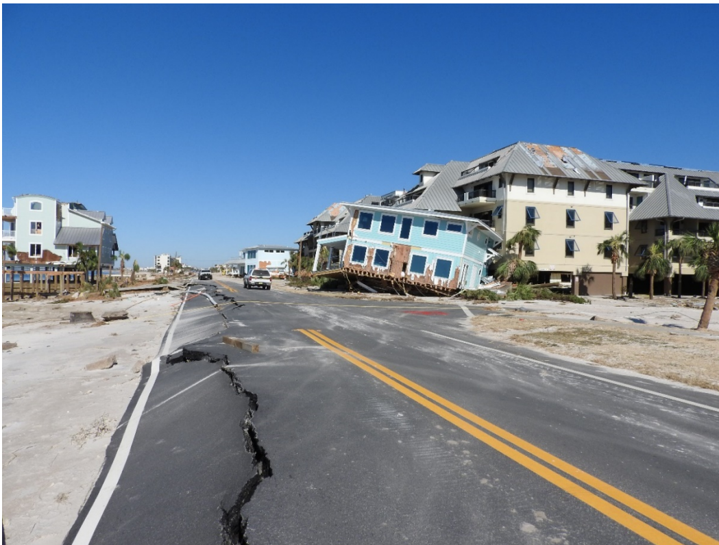
Figure 32. Dwelling transported across U.S. 98 by the storm surge near R136.
