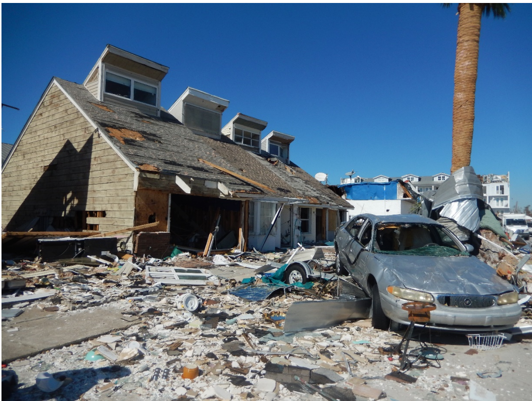
Figure 26. Multifamily dwelling destroyed near R129, Mexico Beach.
