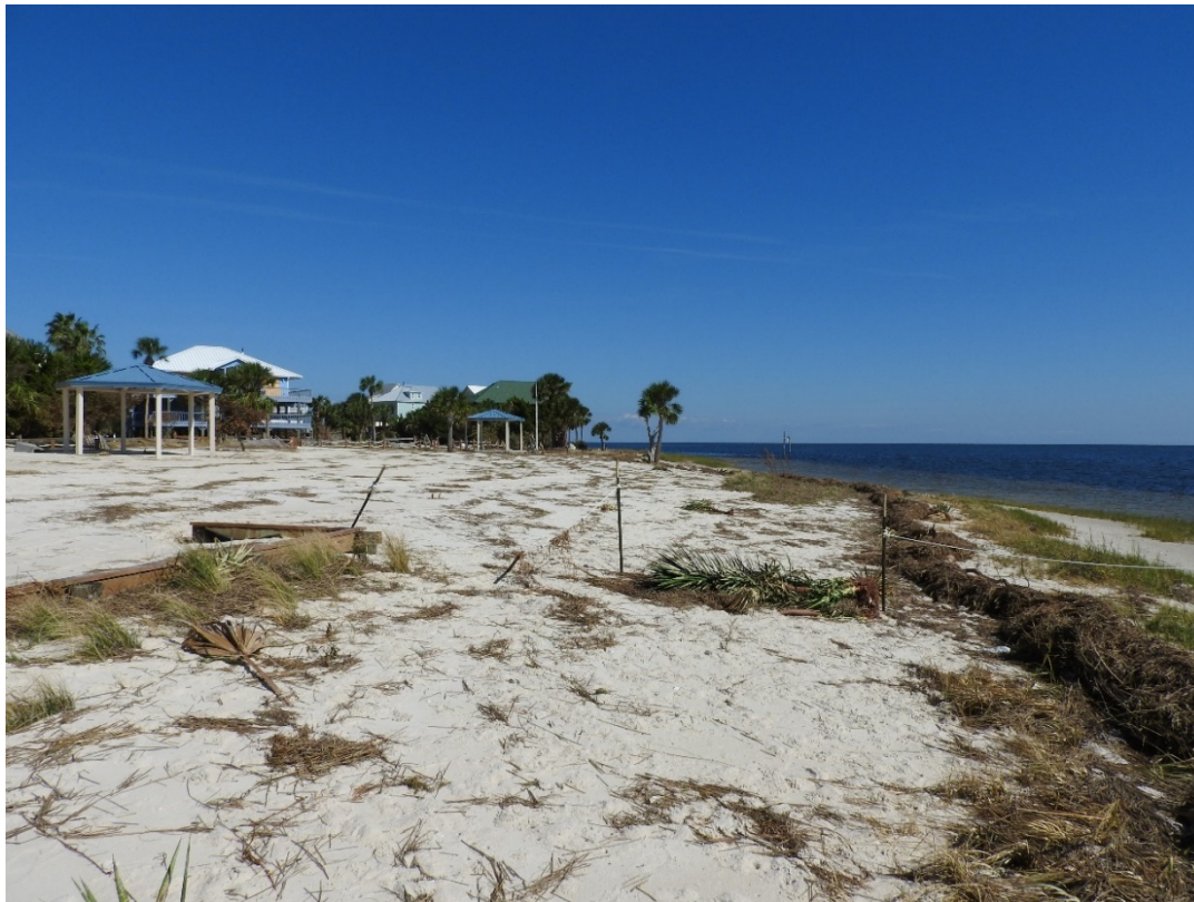
Figure 96. Minor erosion to public beach at Shell Point, V355.
