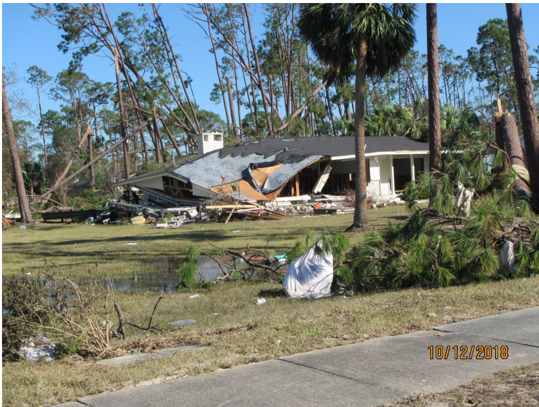
Figure 52. Dwelling destroyed by the storm surge from St. Joseph Bay, Port St. Joe.
