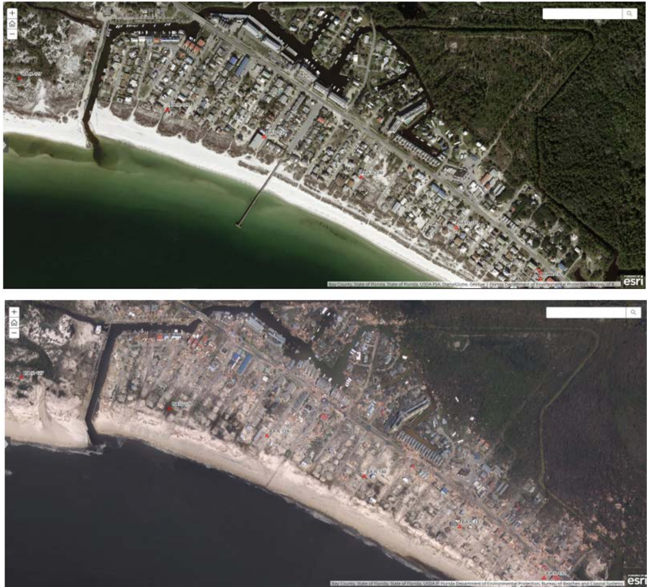
Figure 8. Aerial photo comparison of the severe damage in Mexico Beach (R127-R132).
