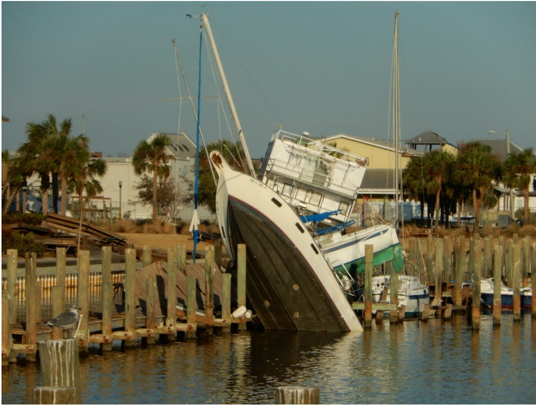
Figure 49. Marina damage due to the storm surge, Port St. Joe.
