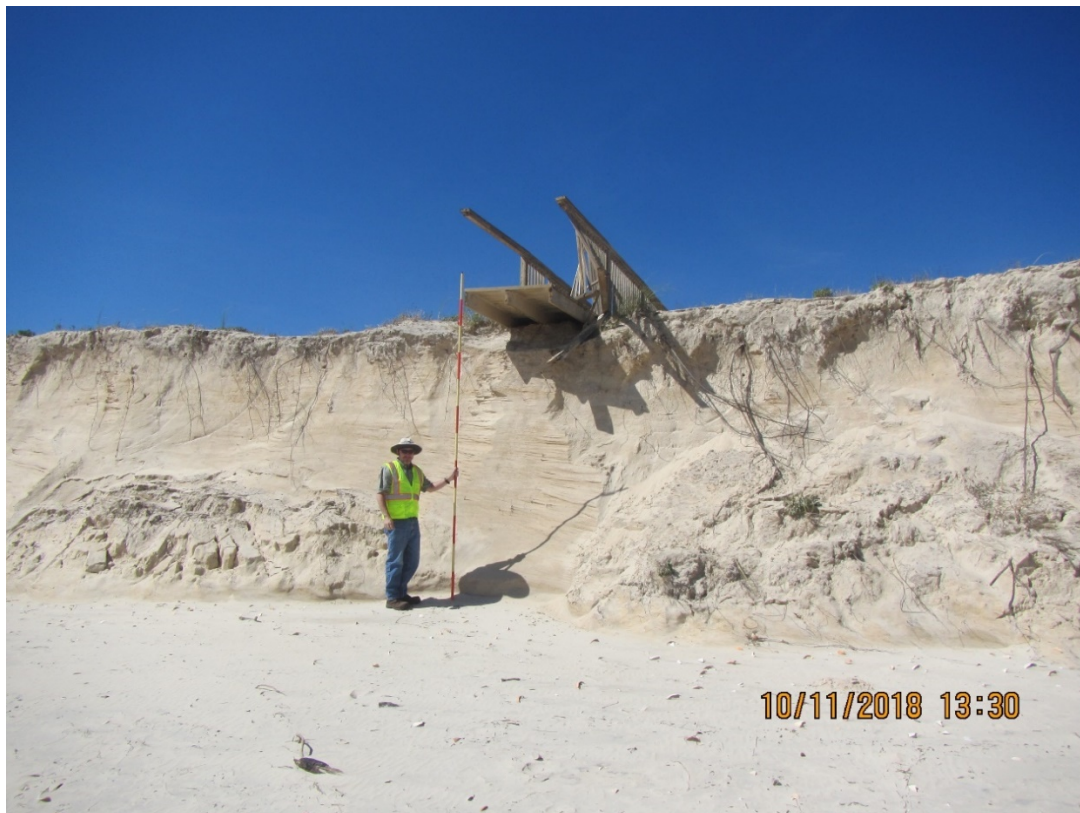
Figure 73. Major dune erosion at R72, St. George Island.
