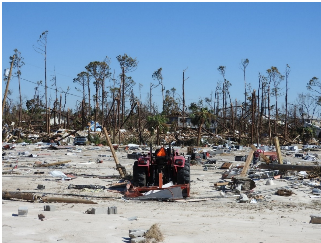
Figure 38. Storm surge transported debris and sand overwash across U.S. 98 near R135, Mexico Beach.
