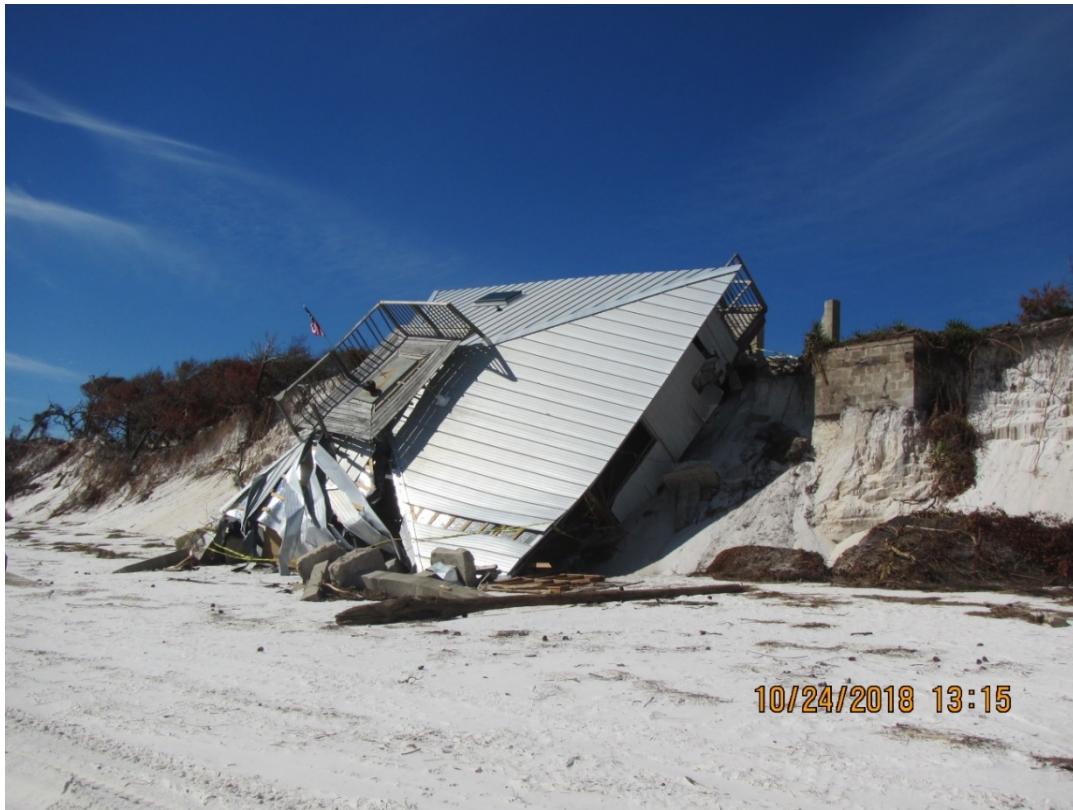
Figure 82. Dwelling destroyed near R173, Dog Island.
