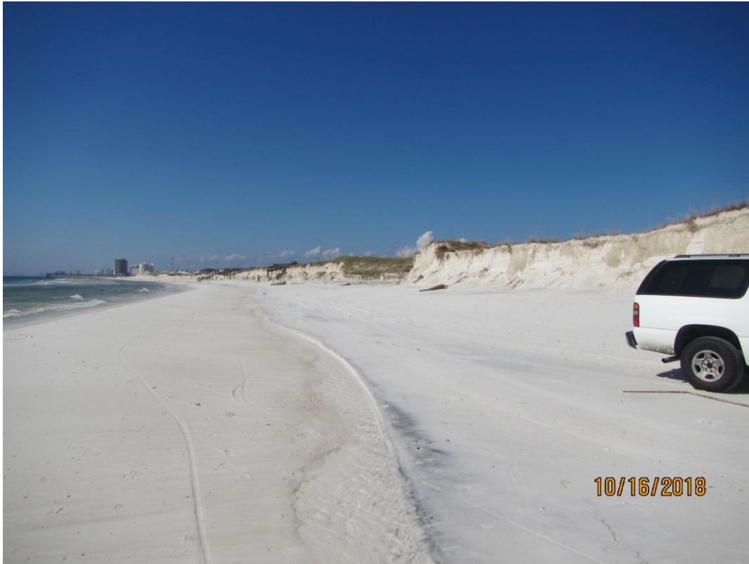
Figure 18. Beach and dune erosion near R97, St. Andrews State Park.
