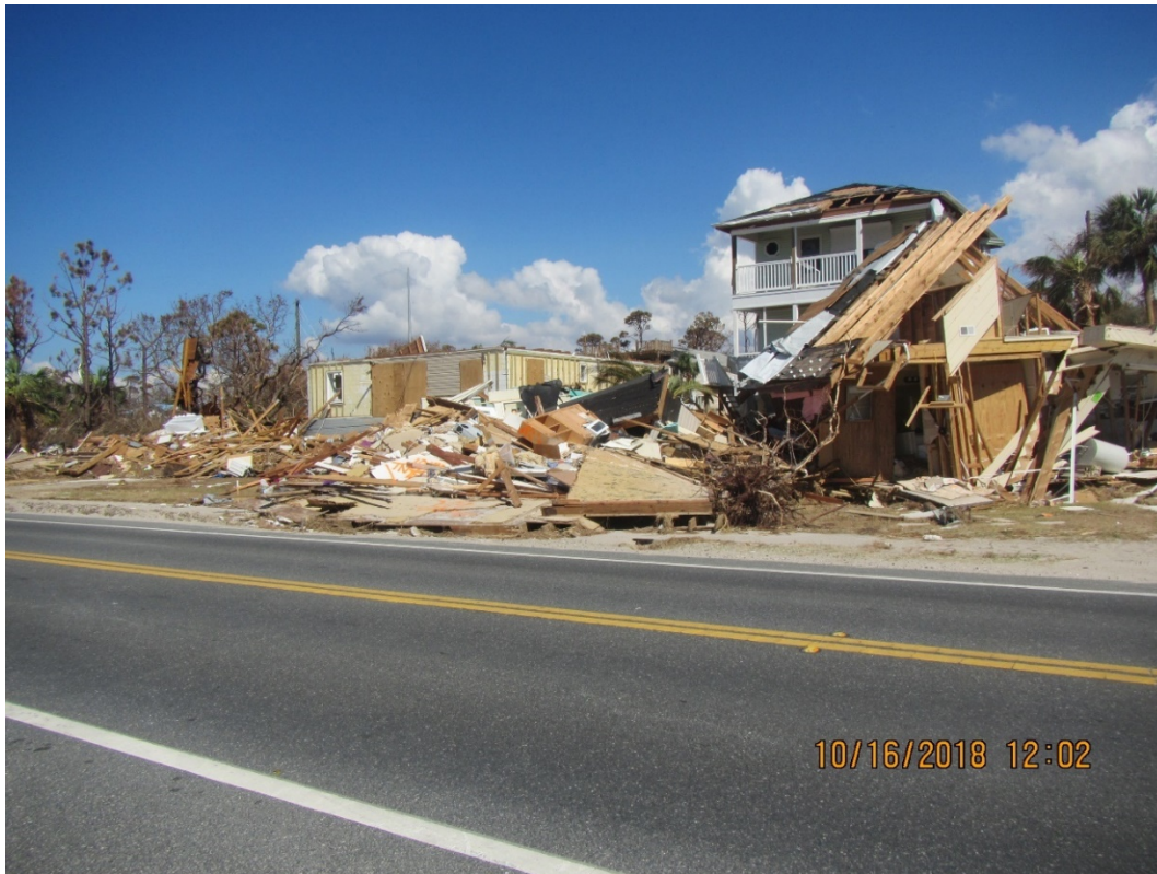
Figure 42. Dwellings along U.S. 98 destroyed near R3, Beacon Hill.
