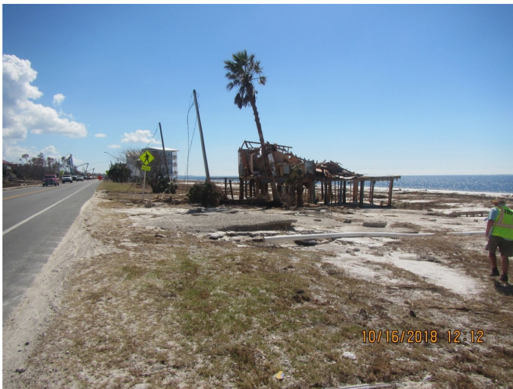
Figure 43. Dwellings destroyed along U.S. 98 near R3.5, Beacon Hill.
