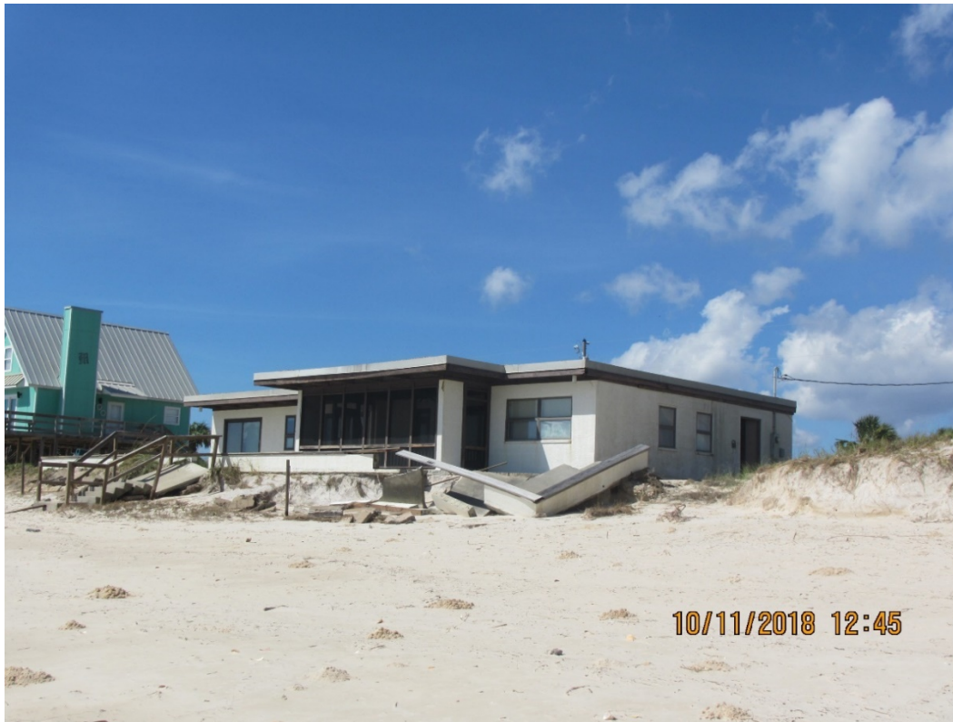
Figure 74. Dwelling damaged near R78, St. George Island.
