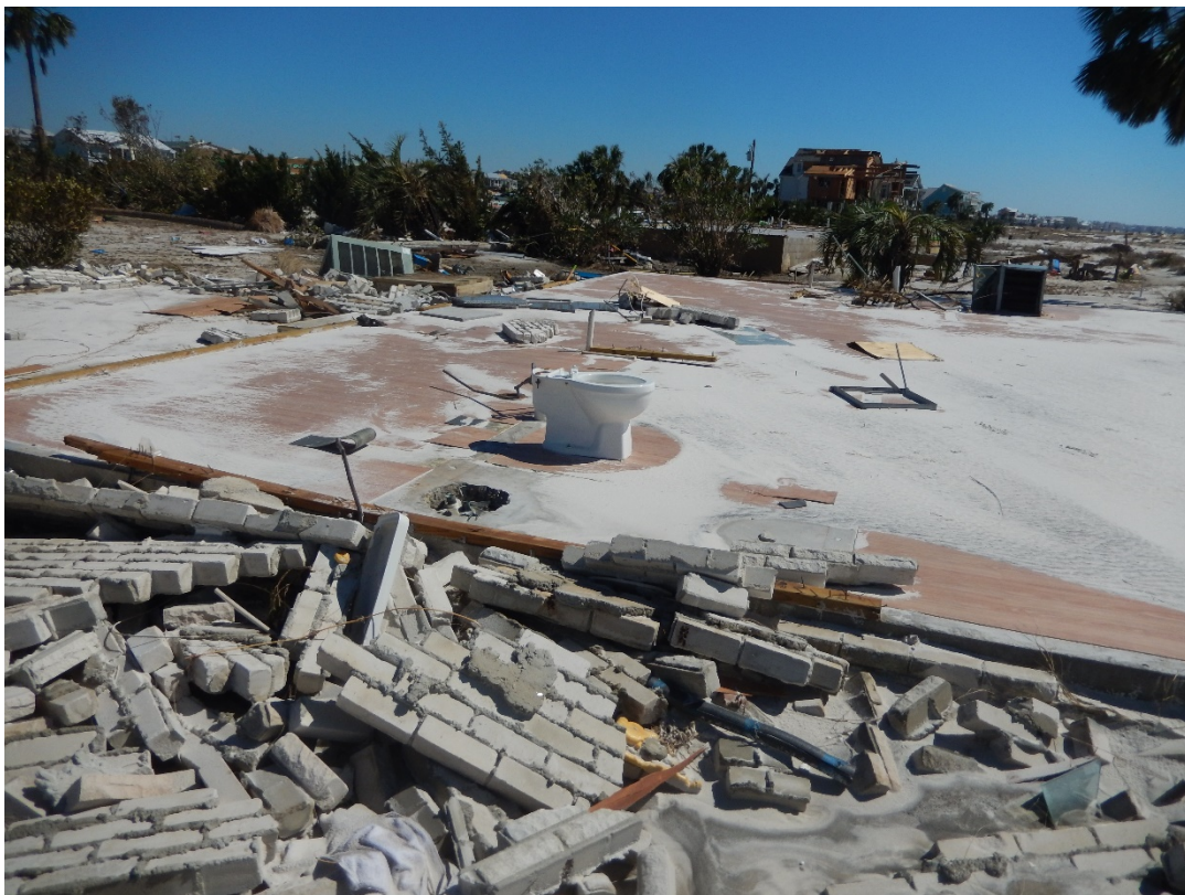
Figure 24. Remains of typical beach house destroyed near R128, Mexico Beach.
