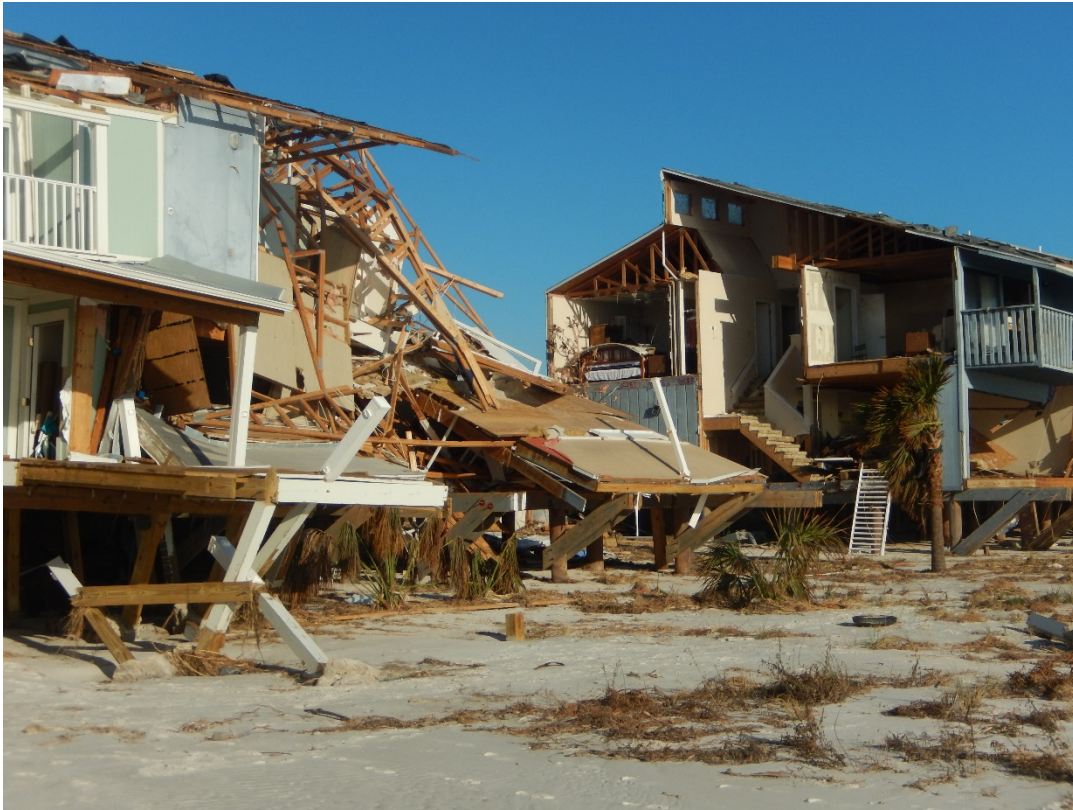
Figure 47. Townhouses destroyed near R7, Beacon Hill.
