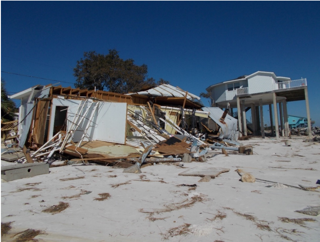
Figure 90. Dwelling destroyed near R211, Southwest Cape.
