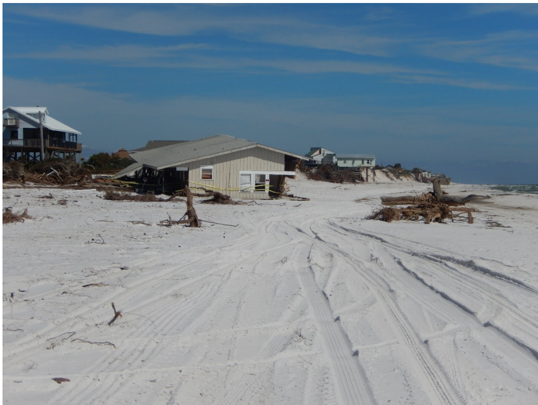
Figure 83. Dwelling destroyed near R174, Dog Island.
