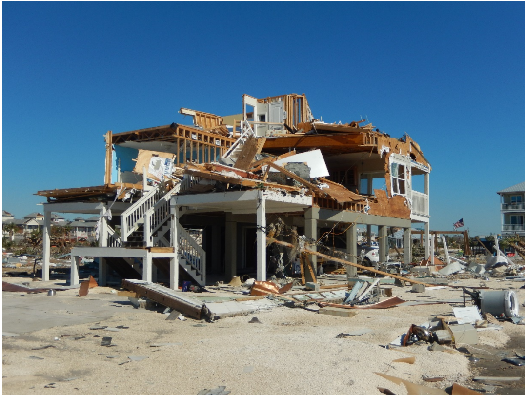
Figure 27. Pile-supported dwelling destroyed near R129, Mexico Beach.
