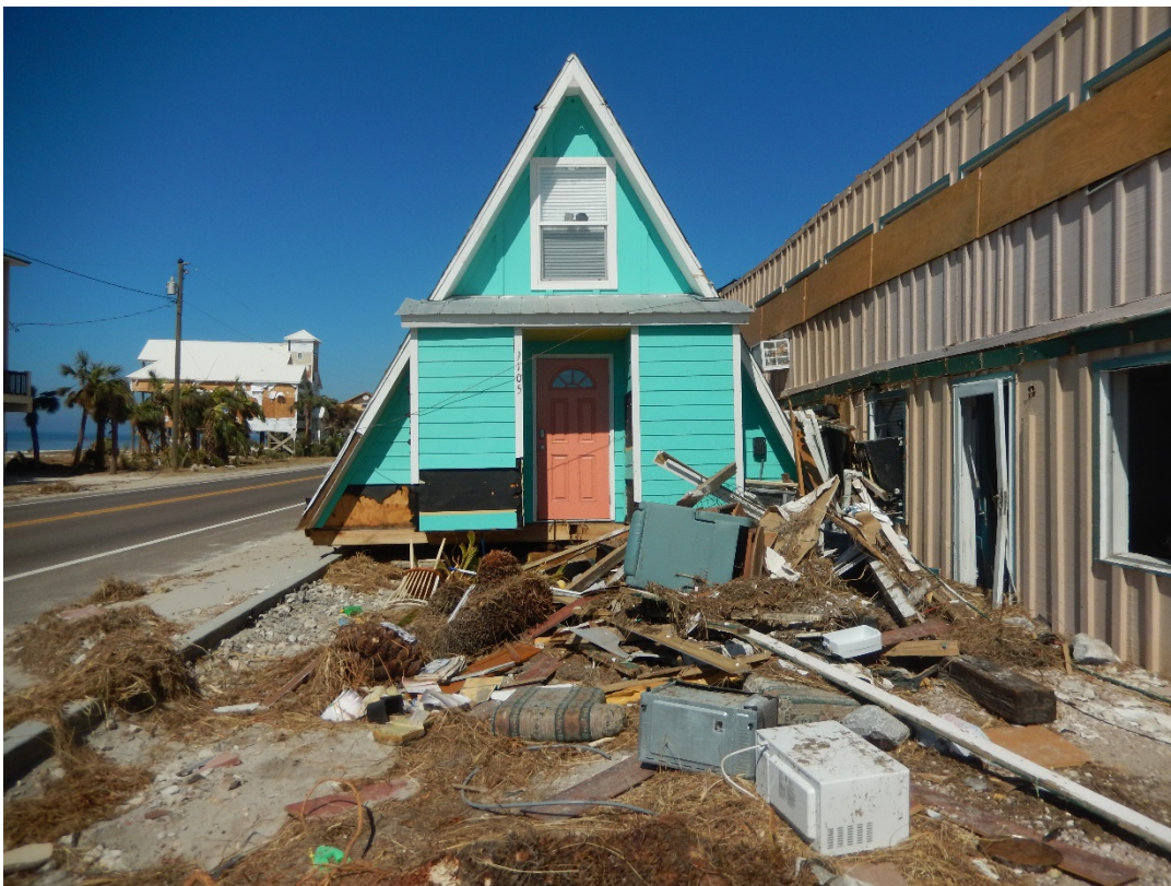
Figure 45. Dwelling transported across U.S. 98 by the storm surge, Beacon Hill.
