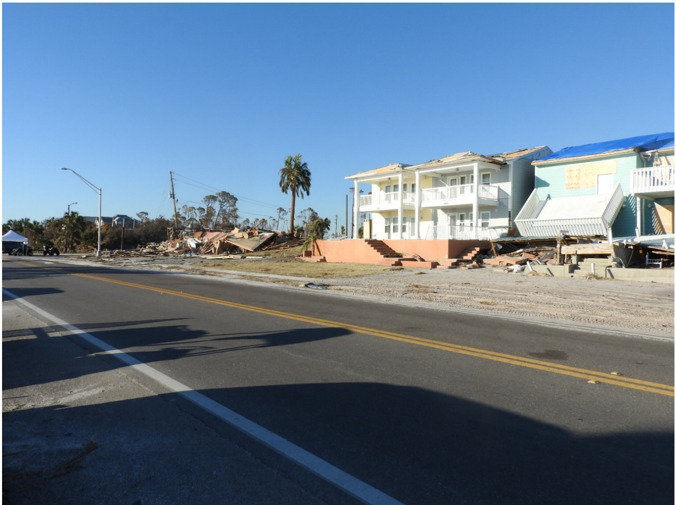
Figure 40. High water mark of +21.2 feet NAVD along U.S. 98 and S.R. 386 near R1, Beacon Hill.
