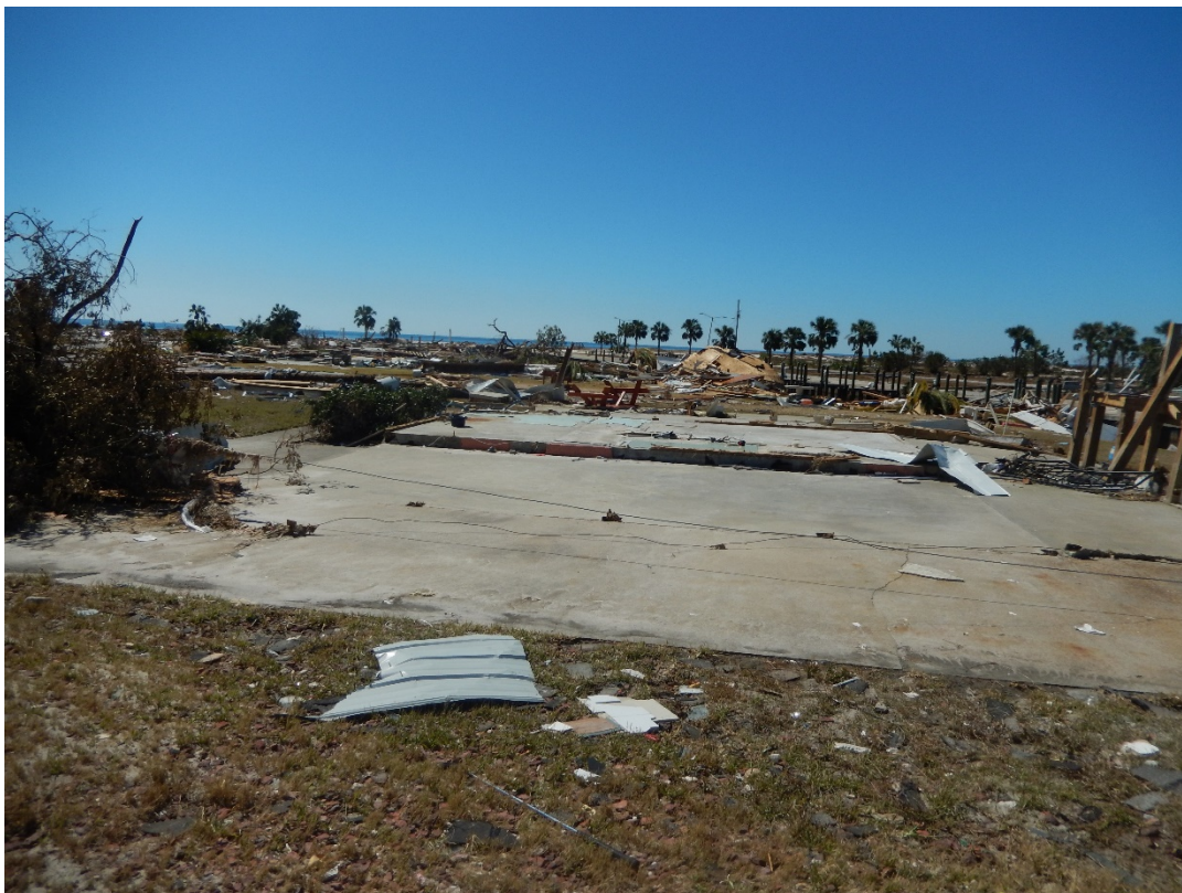
Figure 22. Rows of beach houses destroyed and removed by the storm surge, R127.5.
