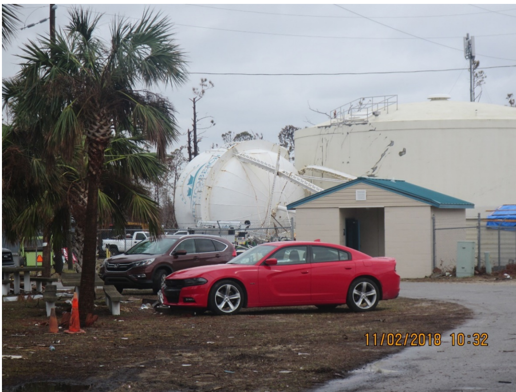
Figure 36. City water tower collapsed under high winds near R134, Mexico Beach.
