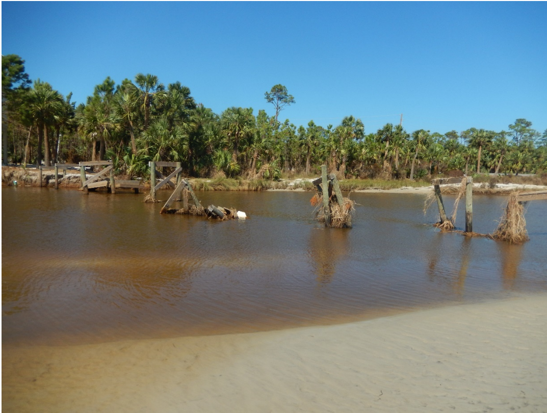
Figure 67. Bridge destroyed across Money Bayou, R140.5.
