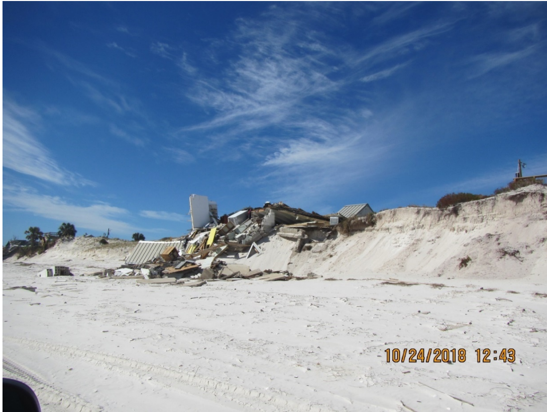
Figure 84. Dwelling destroyed near R176, Dog Island.
