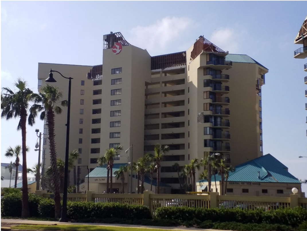
Figure 14. Wind damages on the Sunbird Condominiums near R67, Panama City Beach.
