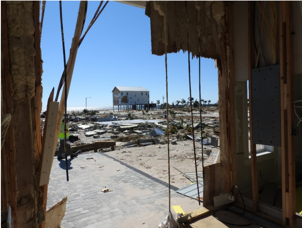
Figure 31. Dwellings destroyed by storm surge near R132, Mexico Beach.
