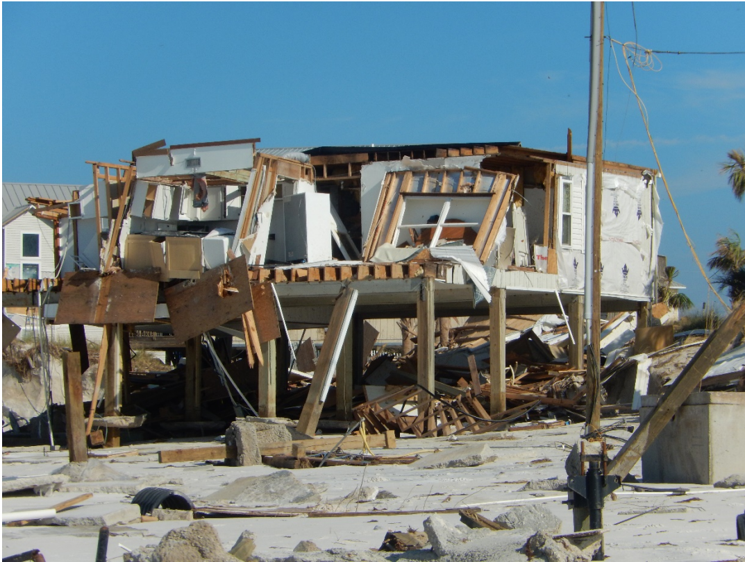
Figure 59. Pile-supported dwelling destroyed near R97.5, St. Joseph Peninsula.
