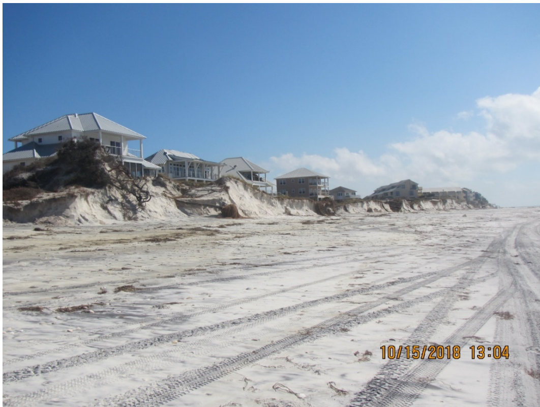
Figure 56. Major dune erosion, R77, St. Joseph Peninsula.
