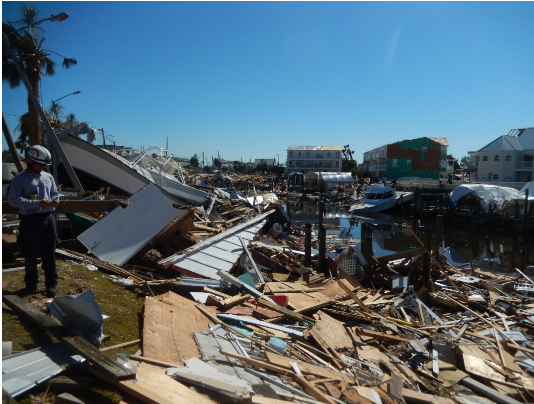
Figure 21. Debris and damages at Mexico Beach Canal, R127.5.
