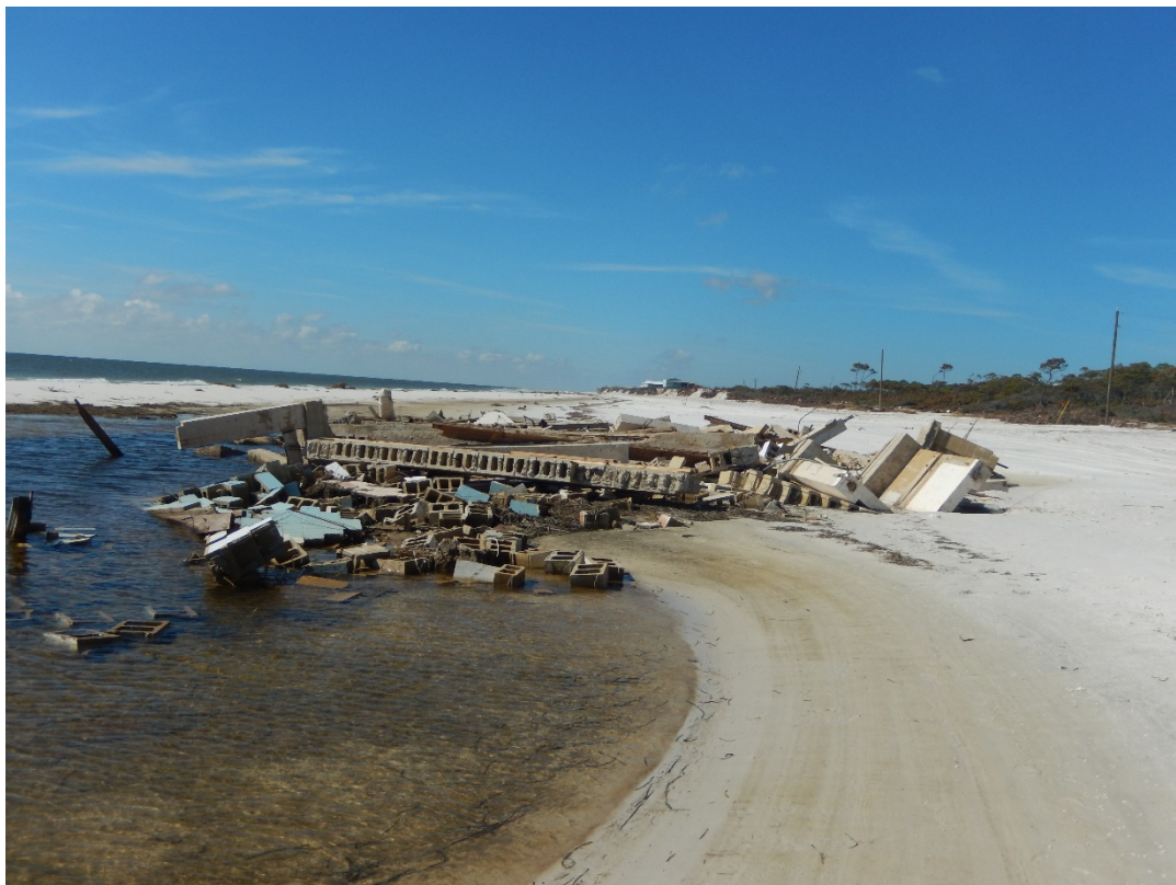
Figure 87. Pelican Inn destroyed near R183, Dog Island.
