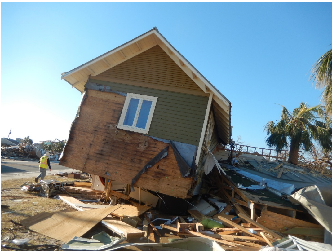
Figure 30. Beach dwelling transported across U.S. 98 by the storm surge.
