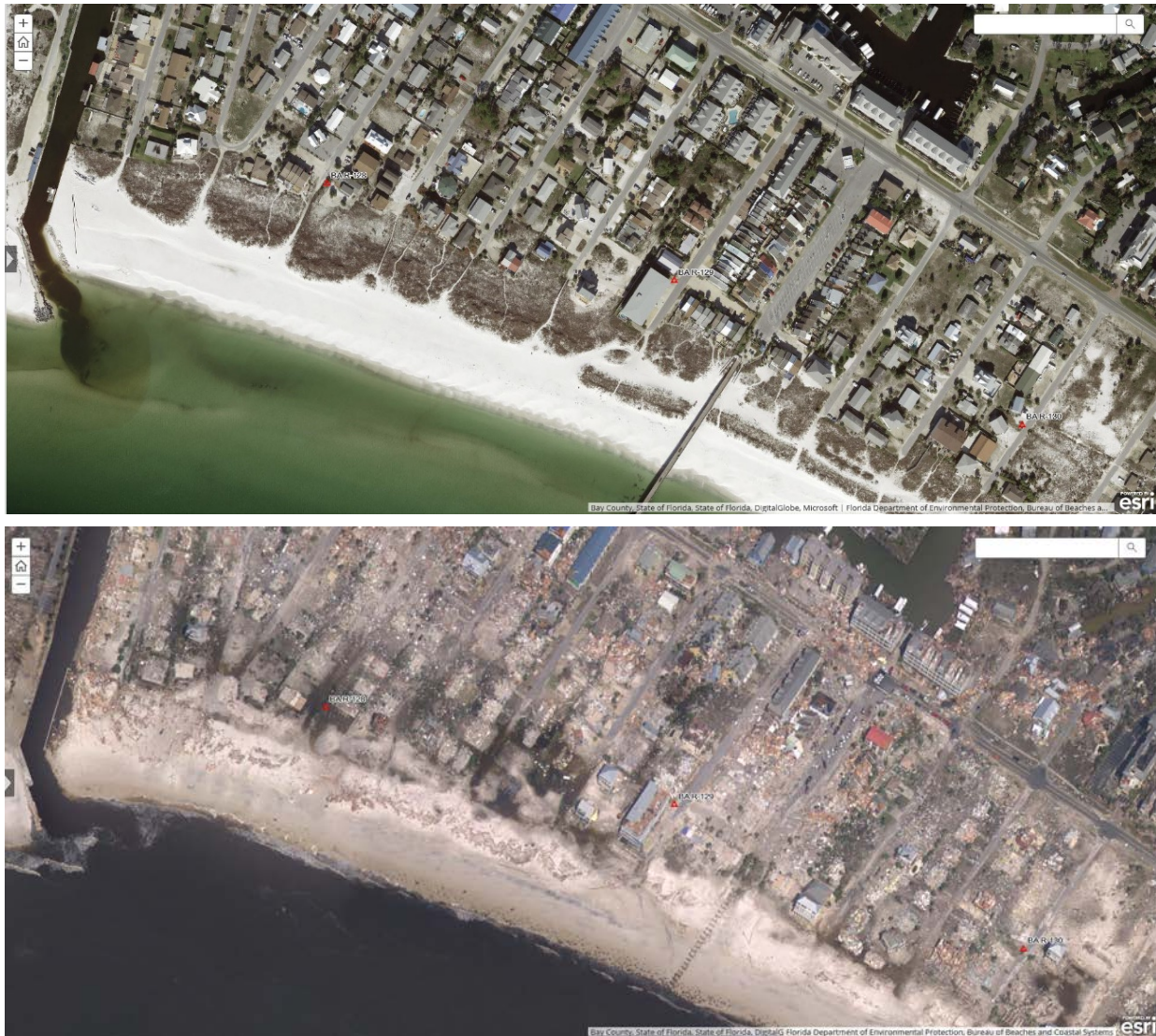
Figure 25. Aerial photo comparison of severe damage in Mexico Beach (R127.5-R130). Source: Vexcel Imaging/ NICB Geospatial Intelligence Center.
