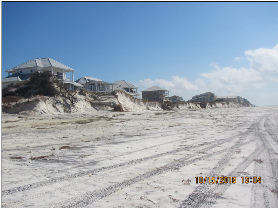
Figure 51. Major dune erosion, R77, St. Joseph Peninsula.
