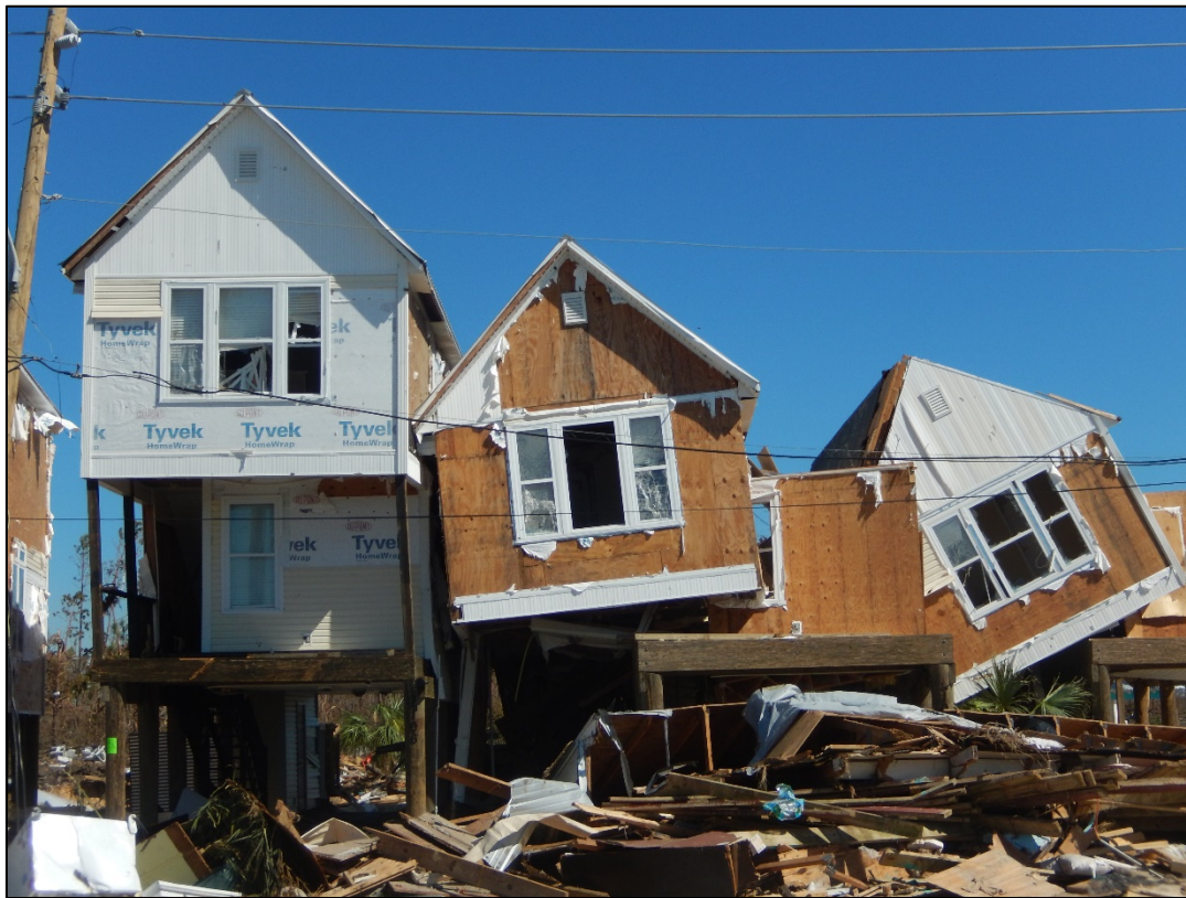
Figure 28. Beach dwellings north of U.S. 98 lifted off their foundations, R128, Mexico Beach.
