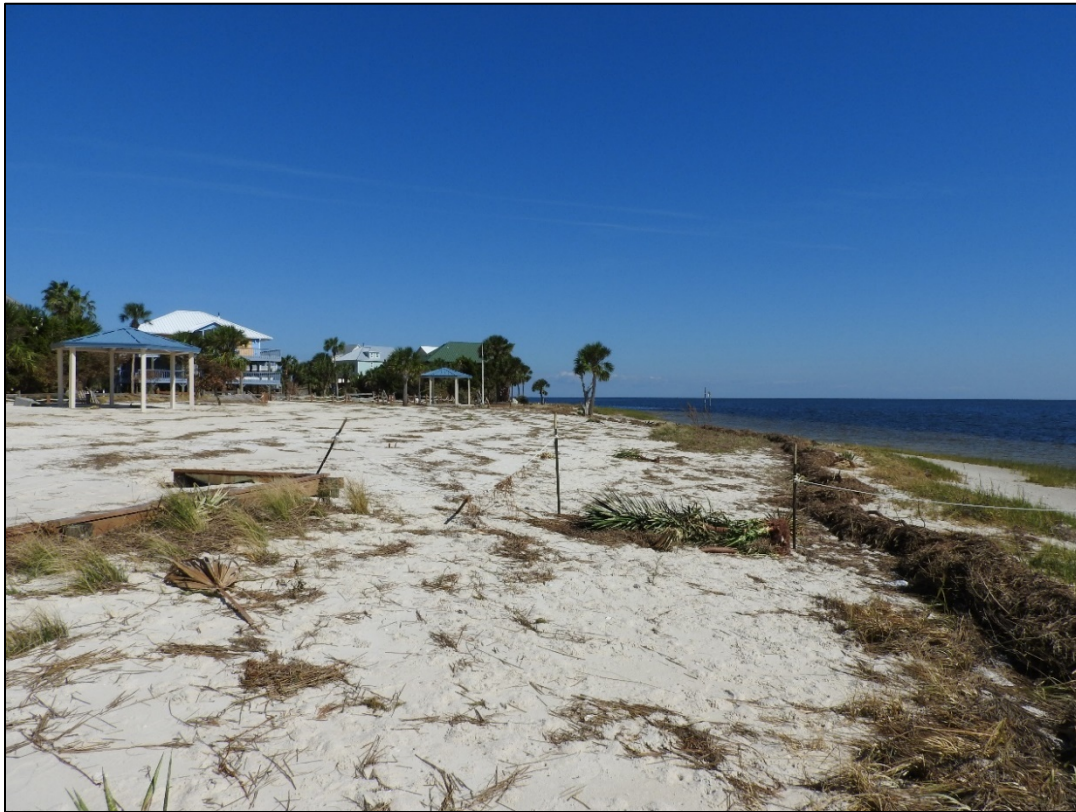
Figure 107. Minor erosion to public beach at Shell Point, V355.
