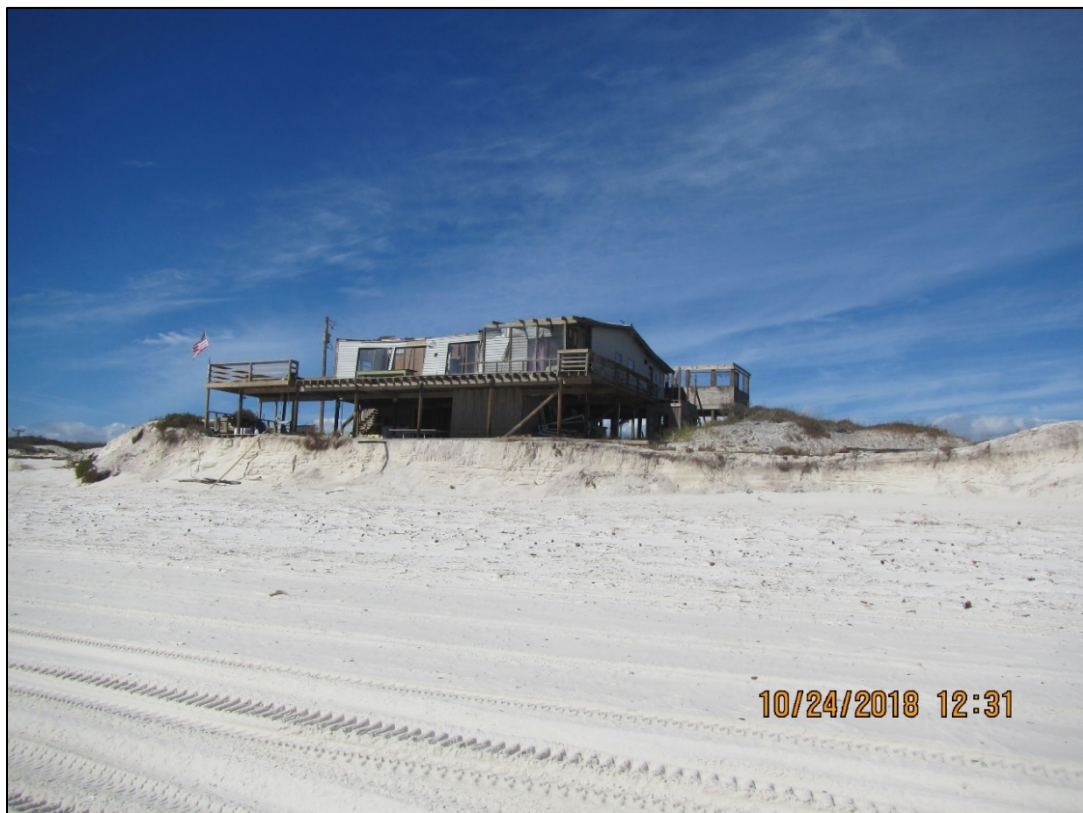
Figure 96. Dwelling destroyed near R178, Dog Island.
