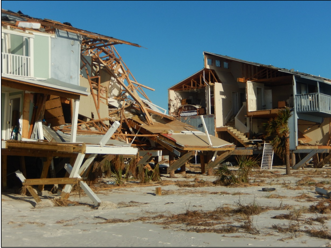
Figure 61. Townhouses destroyed near R7, Beacon Hill.
