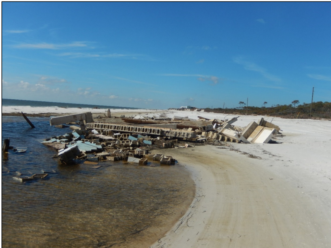
Figure 98. Pelican Inn destroyed near R183, Dog Island.
