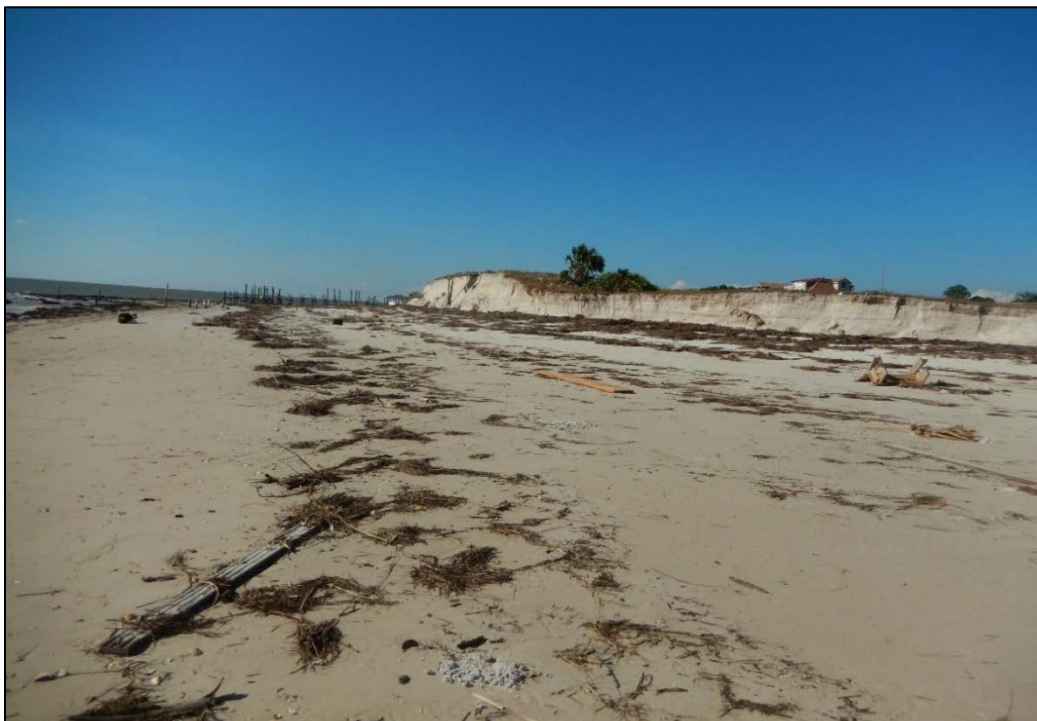
Figure 83. Major beach and dune erosion at Bob Sikes Cut at R52, St. George Island.
