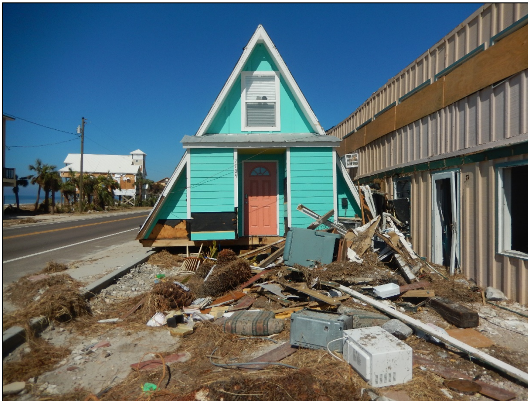
Figure 56. Dwelling transported across U.S. 98 by the storm surge near R2, Beacon Hill.
