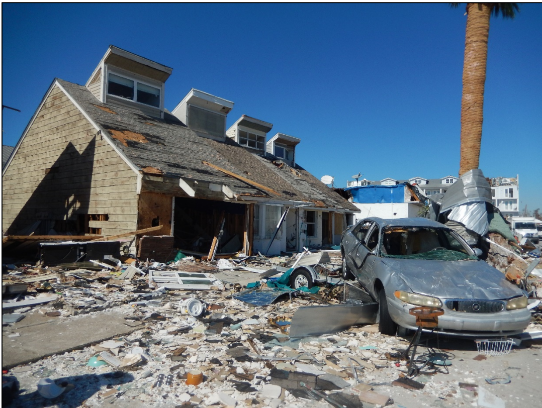
Figure 31. Multifamily dwelling destroyed near R129, Mexico Beach.
