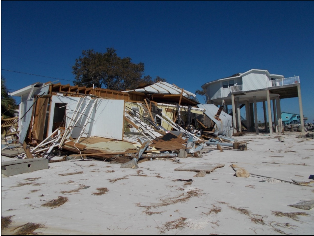
Figure 101. Dwelling destroyed near R211, Southwest Cape.
