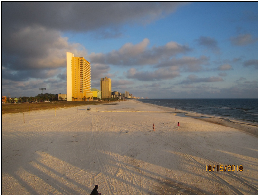
Figure 11. Beach erosion near R57, east of the M.B. Miller Pier, Panama City Beach.
