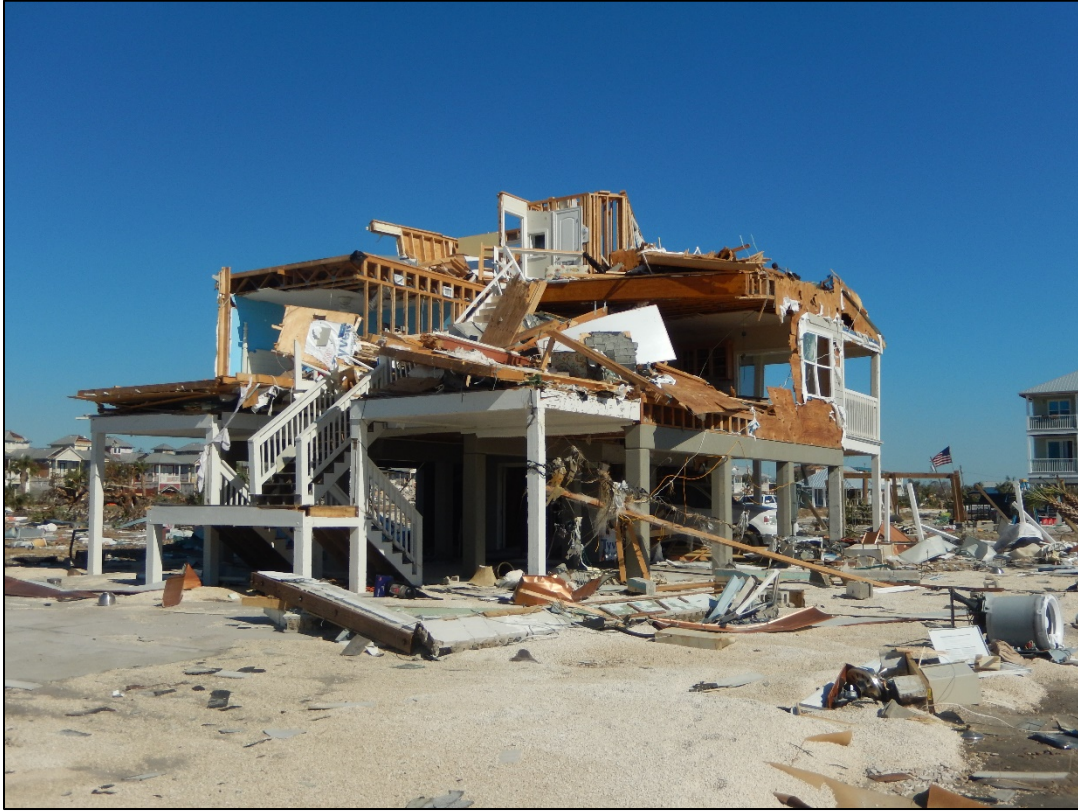
Figure 32. Pile-supported dwelling destroyed near R129, Mexico Beach.
