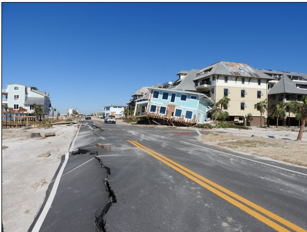
Figure 41. Dwelling transported across U.S. 98 by the storm surge near R136, Mexico Beach.
