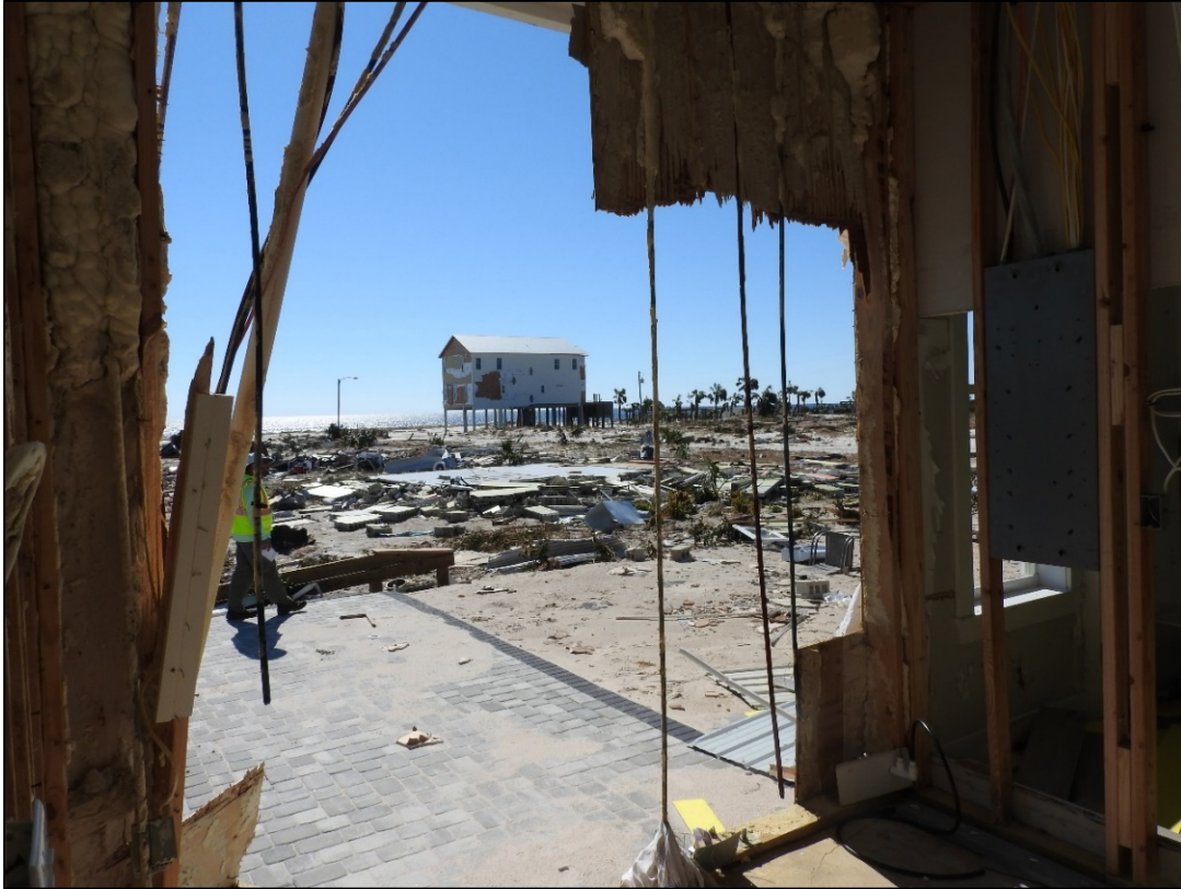
Figure 36. Dwellings destroyed by storm surge near R132, Mexico Beach.
