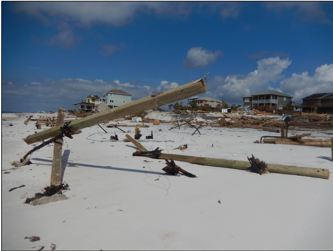
Figure 69. Remains of four destroyed townhouse buildings on Nassau Lane near R90.5, St. Joseph Peninsula.
