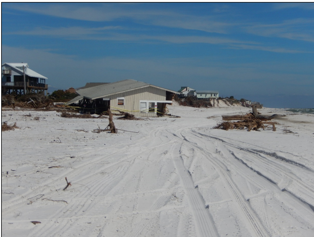
Figure 94. Dwelling destroyed near R174, Dog Island.
