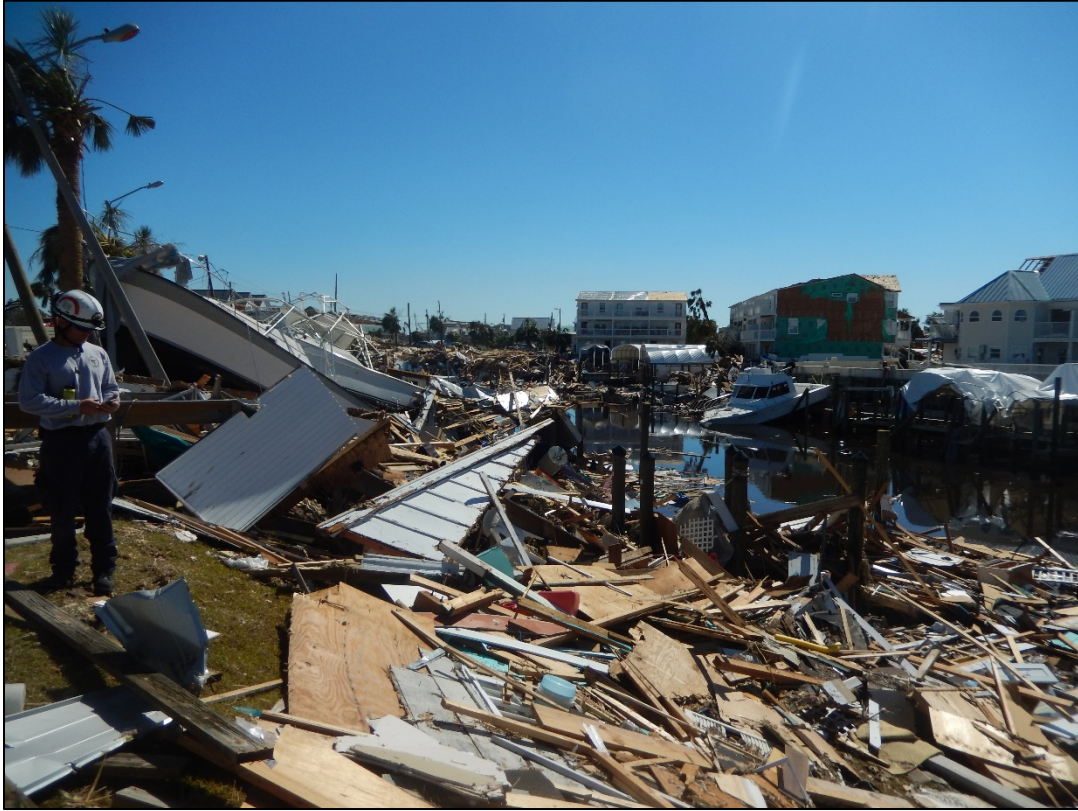
Figure 26. Debris and damages at Mexico Beach Canal, R127.5.
