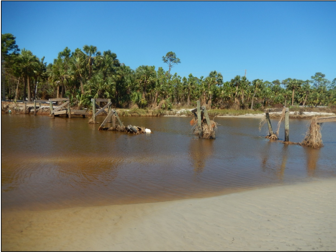
Figure 77. Bridge destroyed across Money Bayou, R140.5.
