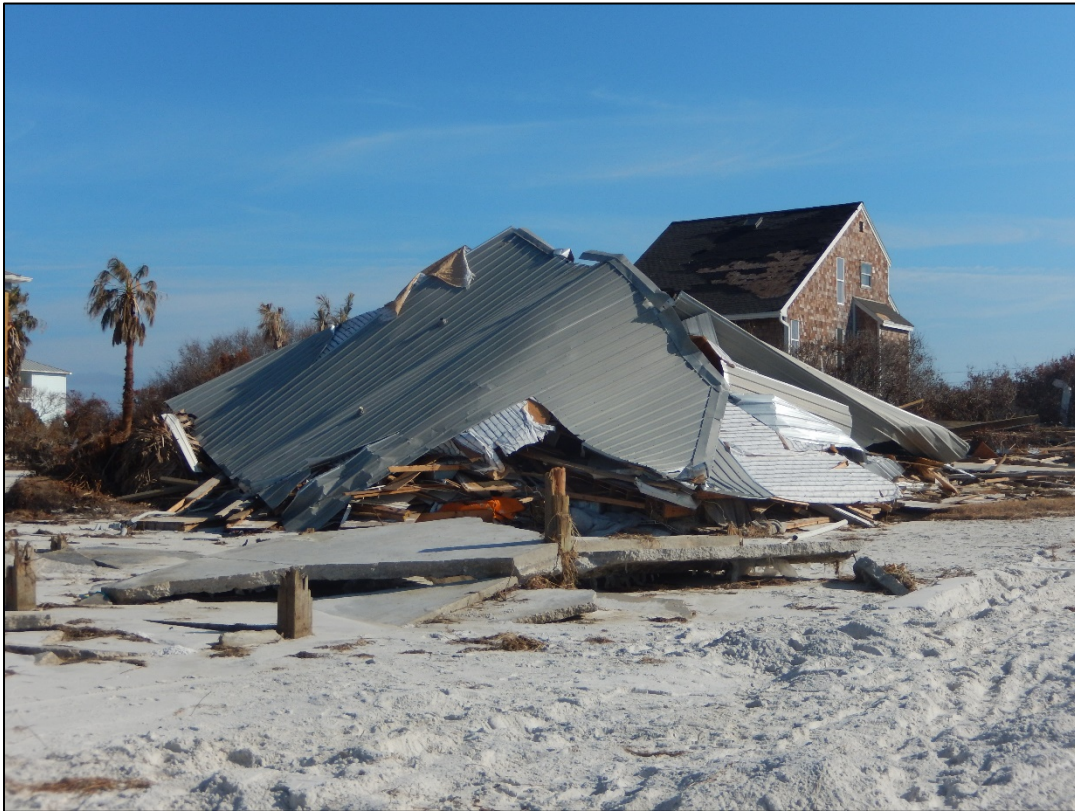
Figure 71. Dwelling destroyed near R99.5, St. Joseph Peninsula.
