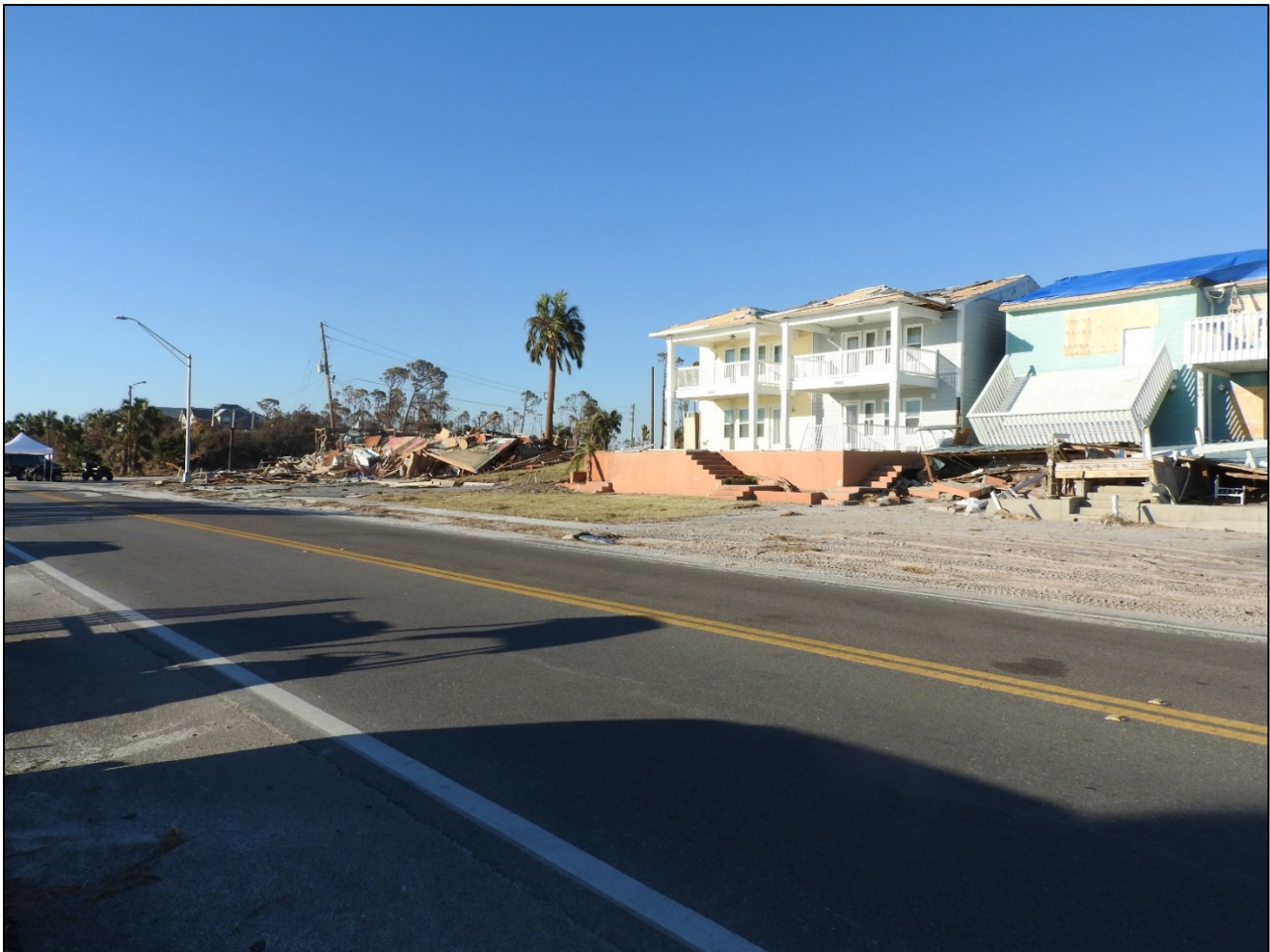
Figure 54. Site of high water mark of +21.2 feet NAVD along U.S. 98 and S.R. 386 near R1, Beacon Hill.
