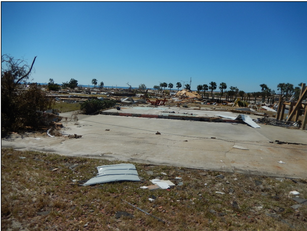
Figure 27. Rows of beach houses destroyed and removed by the storm surge, R127.5, Mexico Beach.
