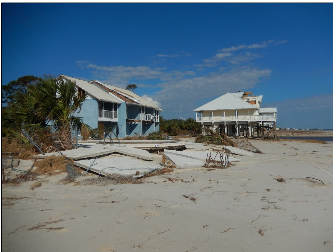
Figure 76. Storm surge damages at Money Bayou, R140.
