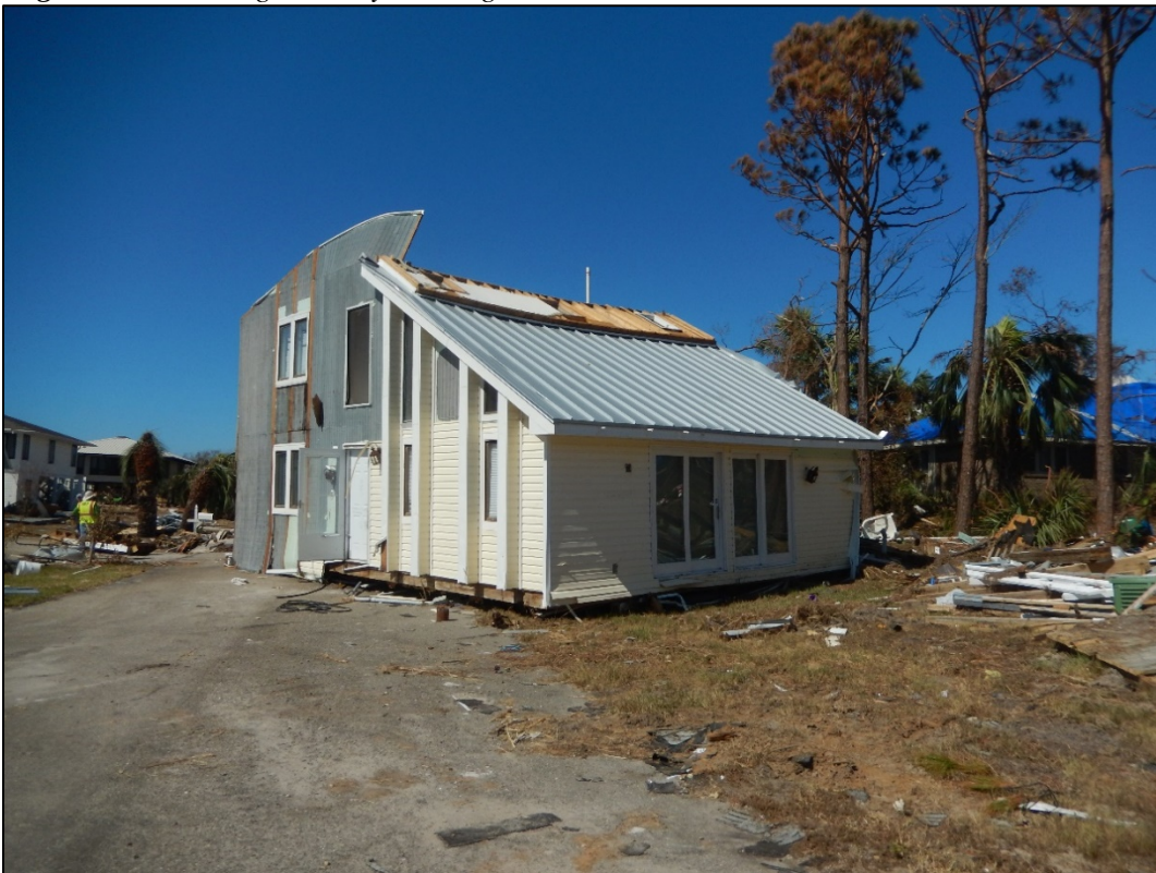
Figure 59. Dwelling transported by storm surge onto Trade Winds Dr. near R6, Beacon Hill.
