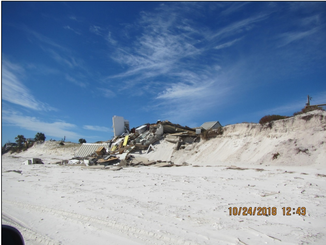
Figure 95. Dwelling destroyed near R176, Dog Island.
