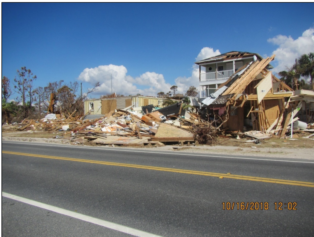
Figure 57. Dwellings along U.S. 98 destroyed near R3, Beacon Hill.
