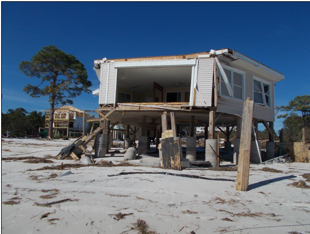
Figure 100. Dwelling destroyed near R210, Southwest Cape.
