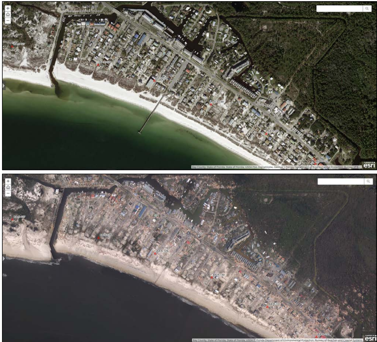
Figure 8. Aerial photo comparison of the severe damage in Mexico Beach (R127-R132). Source: Vexcel Imaging/NICB Geospatial Intelligence Center.
