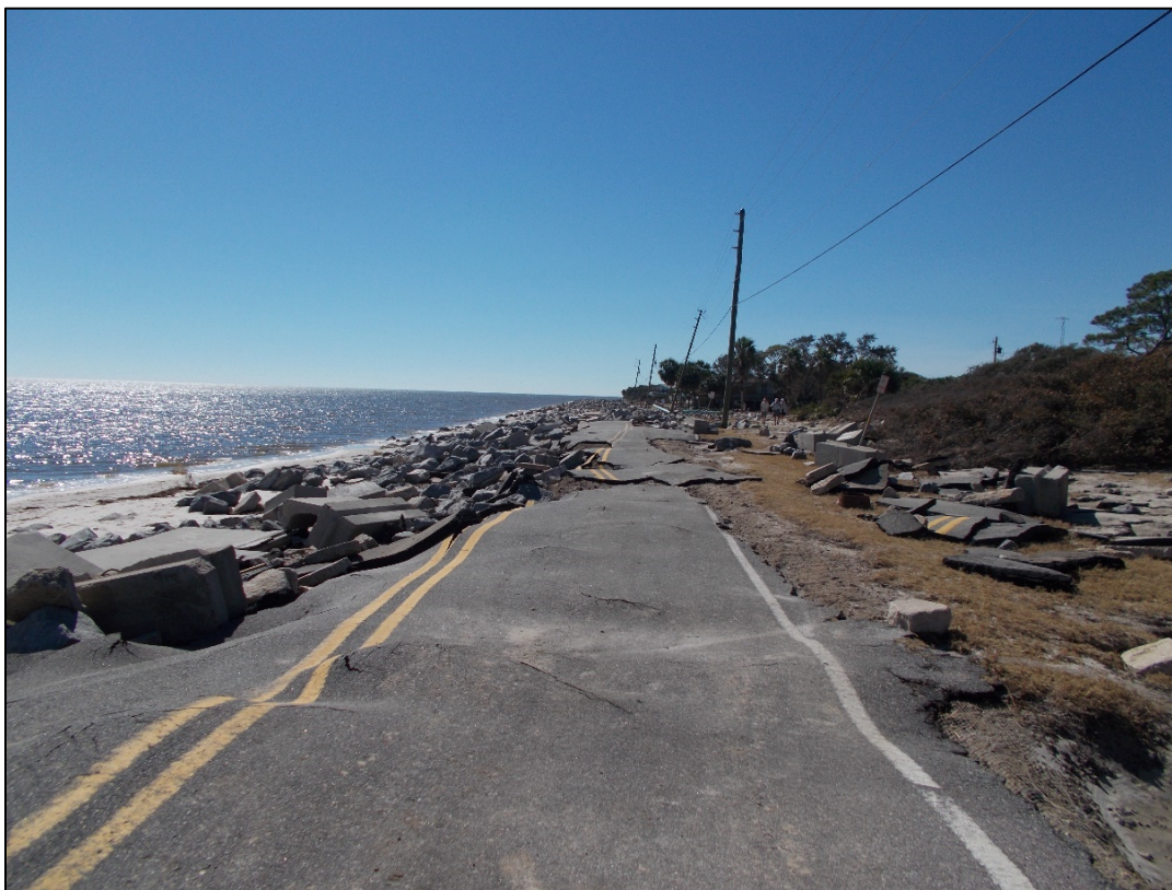
Figure 99. 3,000 feet of road and revetment destroyed between R211-R214, Southwest Cape.
