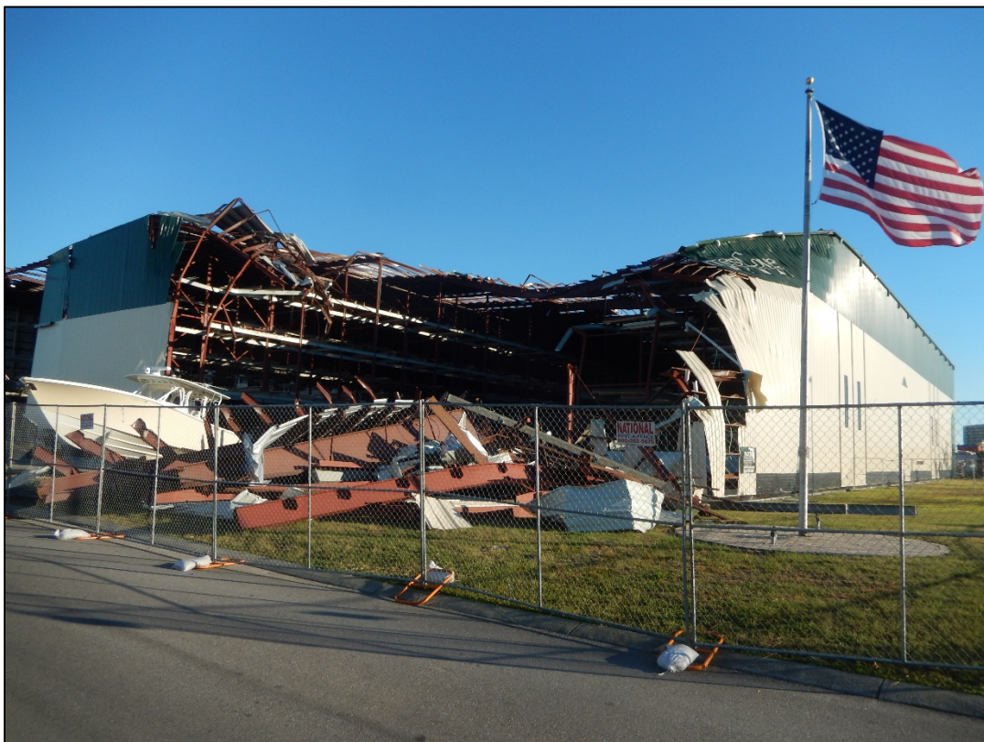
Figure 16. Dry storage marina with wind damage on Thomas Drive, Panama City Beach.
