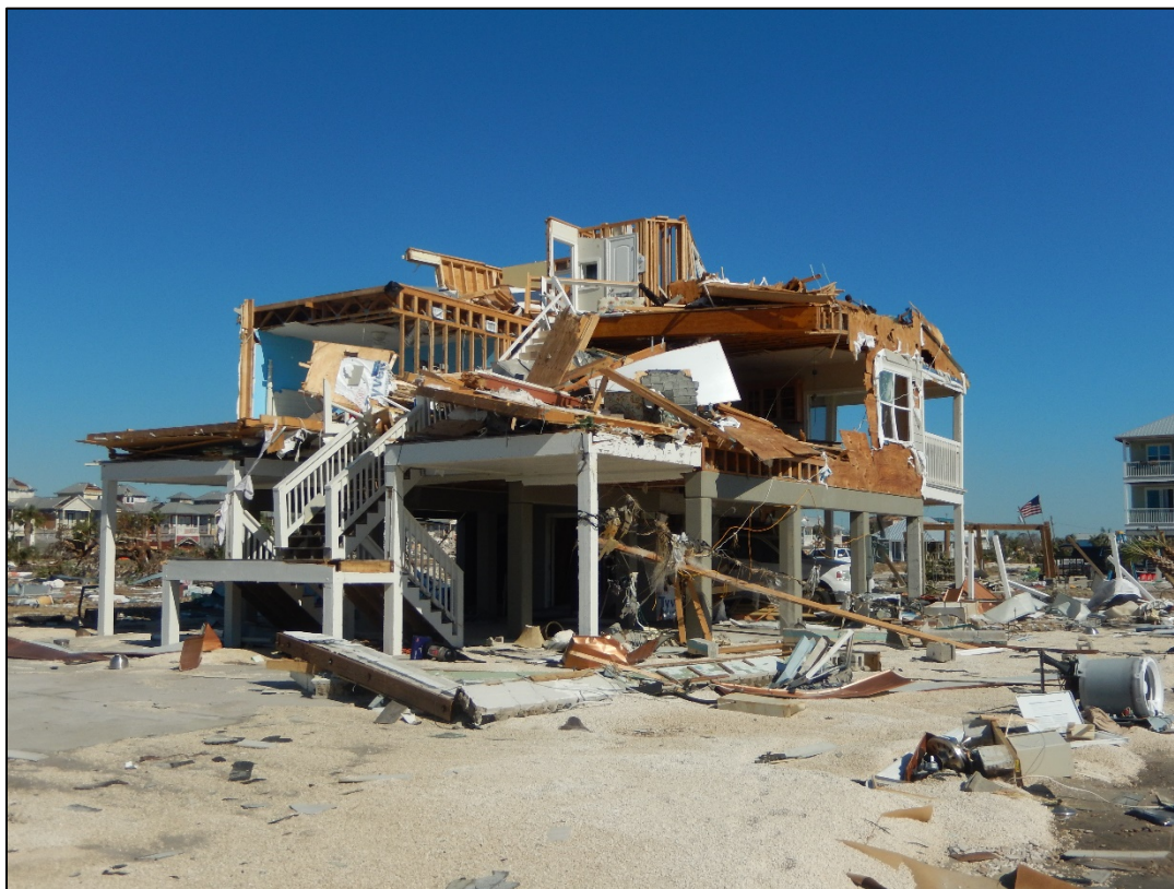
Figure 32. Pile-supported dwelling destroyed near R129, Mexico Beach.
