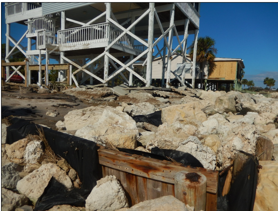
Figure 108. Rock revetment damaged and dwelling with parking slab and bracing damage at Shell Point, V361.
