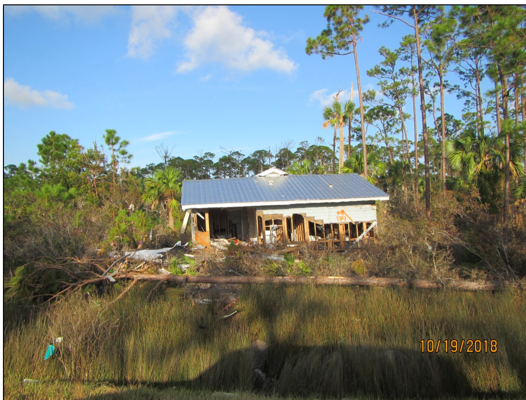
Figure 67. Destroyed dwelling transported across S.R.30A by the storm surge, St. Joseph Bay.
