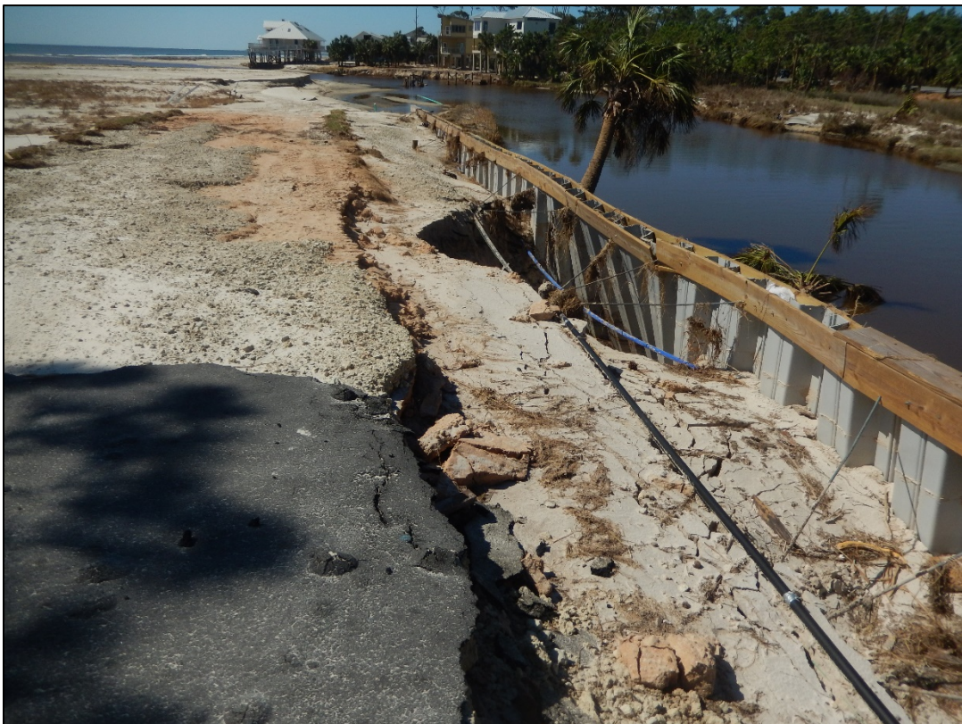
Figure 78. Bulkhead on Money Bayou damaged, R141.
