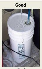
← Separator Water should be accumulated in a closed container, located within <u>secondary</u> containment.
