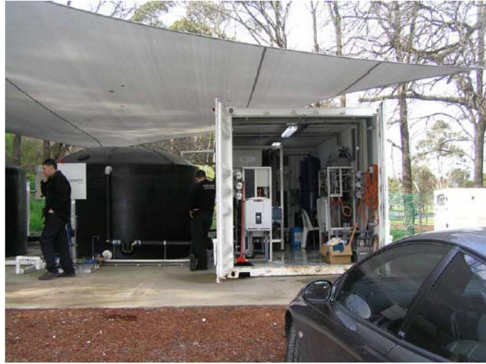
Figure 5-13. Flemington Racecourse Satellite Water Reclamation Facility (Waste Technologies of Australia 2006).
