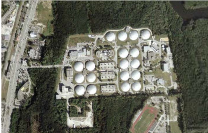
Figure 2-7. Aerial photograph of the Miami-Dade/North WWTP (Google Earth 2005)
