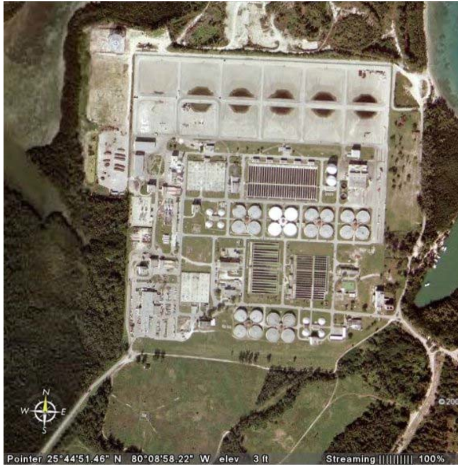
Figure 2-8. Aerial photograph of the Miami-Dade/Central WWTP (Google Earth 2005)
