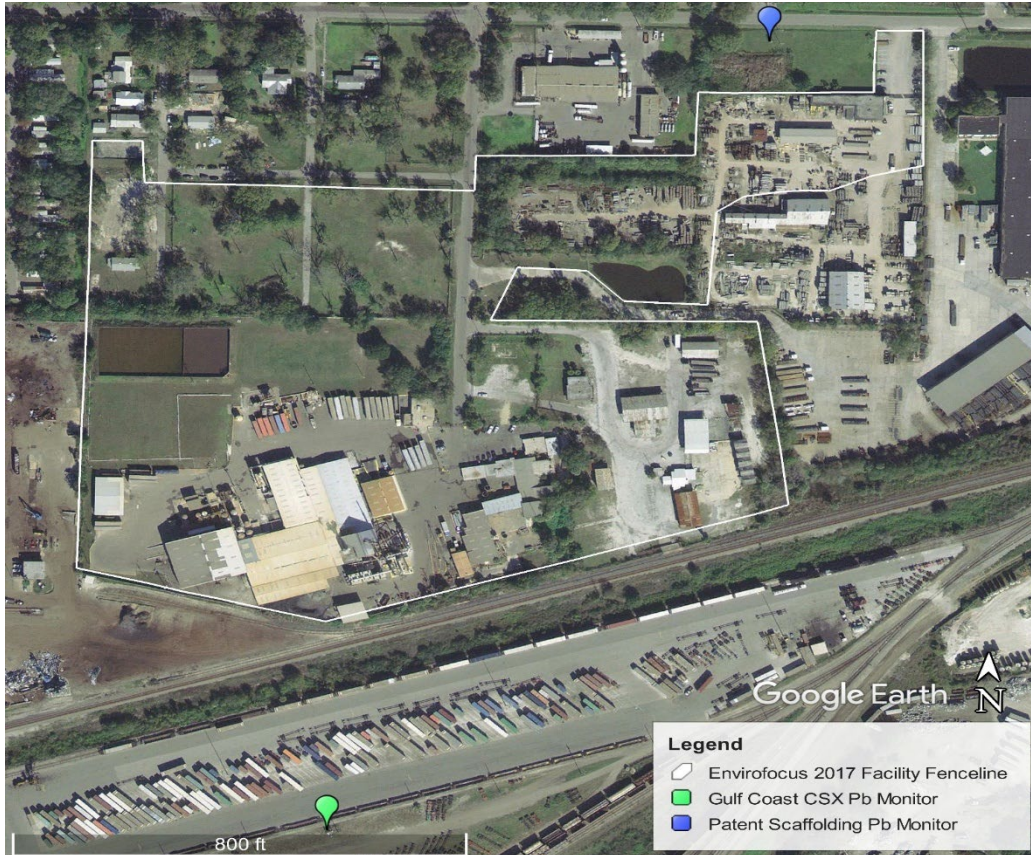
Figure 2. Satellite image of the Envirofocus facility before the reconstruction/modernization.
