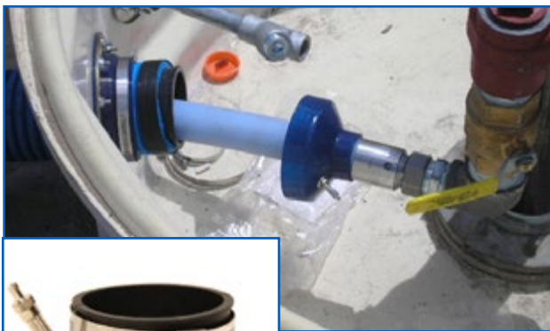
Test Boot Installed, Pulled Back After Testing
