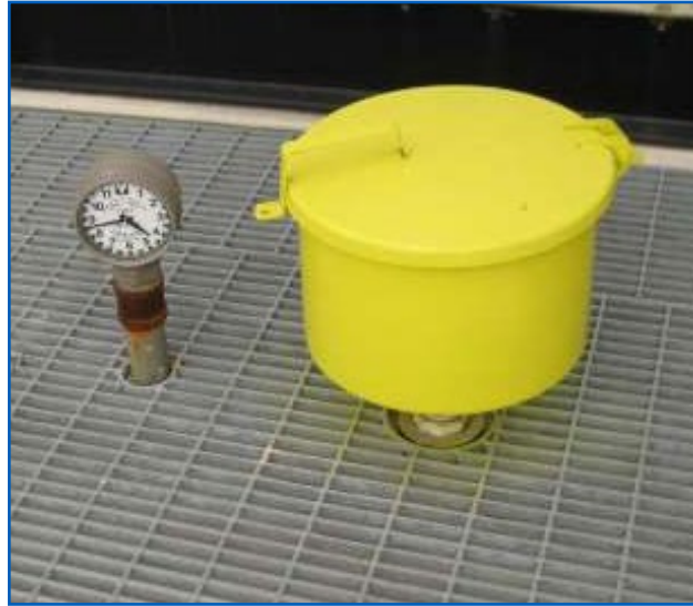
Clock Gauge Liquid Level Overfill Method
