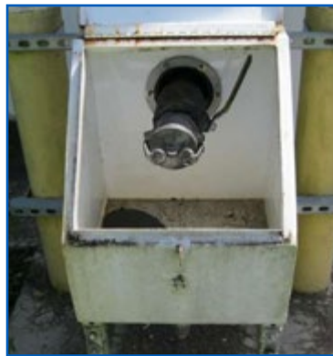
AST Remote Fill/Spill Containment
