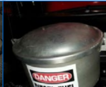
AST Remote Fill/Spill Containment
