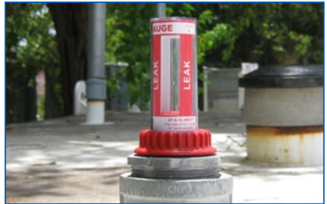
Mechanical RD Gauge
