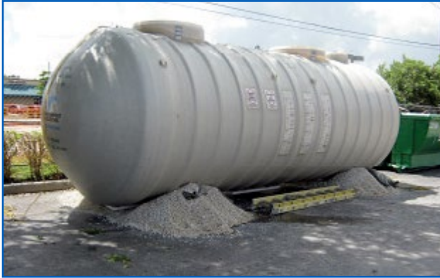
DW-Fiberglass UST Prior to Install
