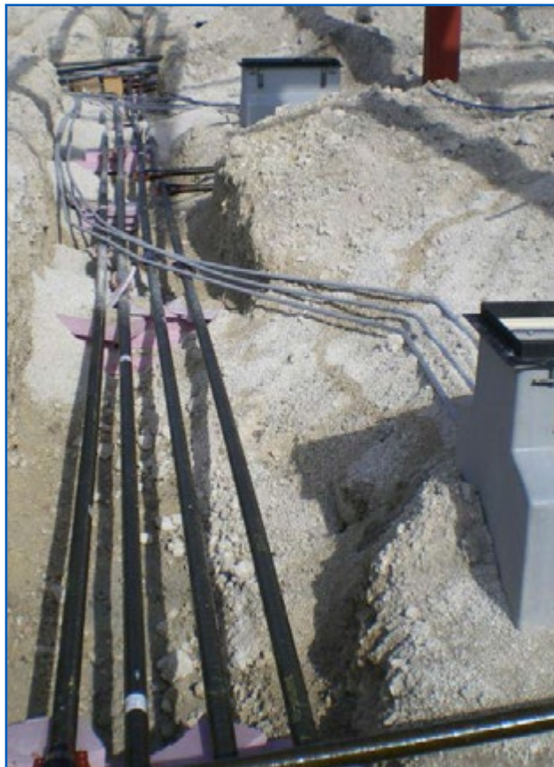
UST System Piping/Dispenser Liner Installation
