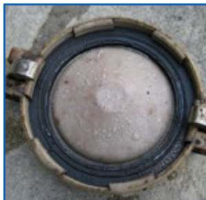
Fill Cap with Gasket
