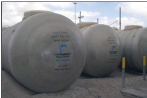
DW-Fiberglass USTs On-site, Pending Installation
