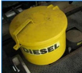
Miscellaneous Types of AST Spill Containment
