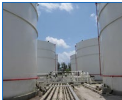
Piping for Field Erected AST
