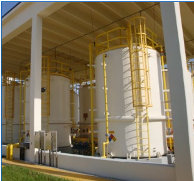
Check Roof for Integrity for Leaks, Especially after a Storm Event
