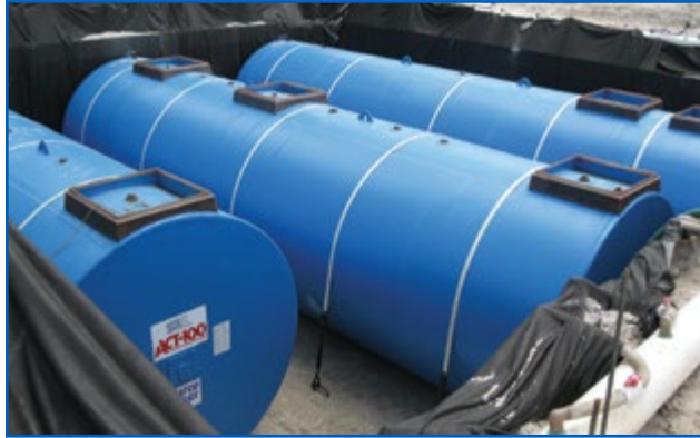
DW-Fiberglass Coated Steel Composite USTs During Installation
