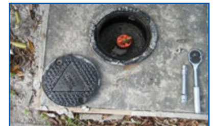
Cap in Place
