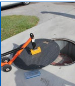
Pump/Piping Sump Manway Cover
