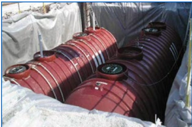
DW-Fiberglass USTs During Installation
