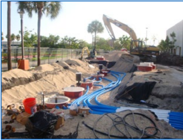
Double-walled Flexible Piping Layout
