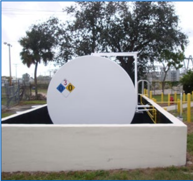
Check Tank Coating and Secondary Containment Integrity
