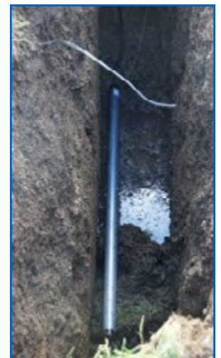
Sacrificial Anode Install
