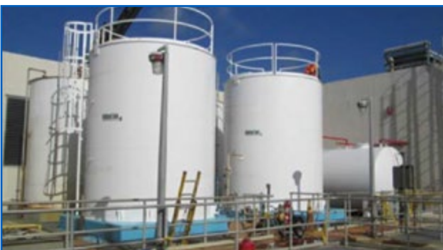
Double-walled Vertical Steel ASTs
