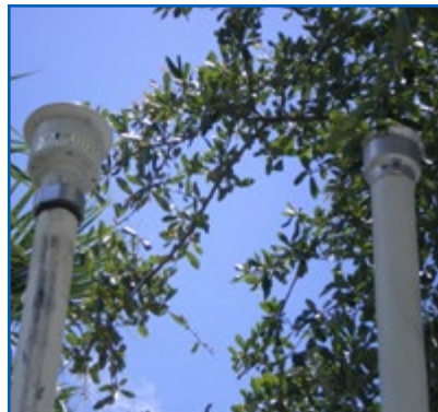
Vent Lines with Valves Installed
