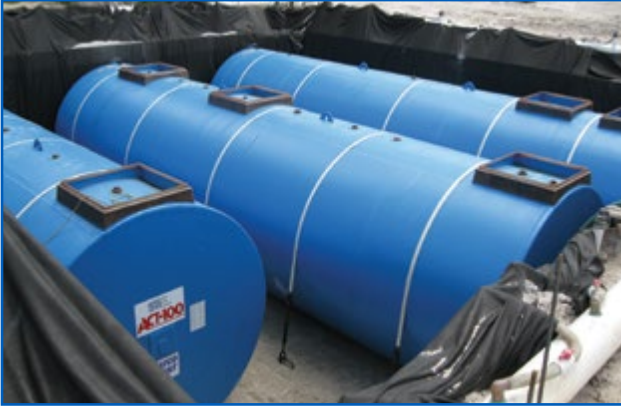
Double-walled Fiberglass-coated Steel USTs during installation
