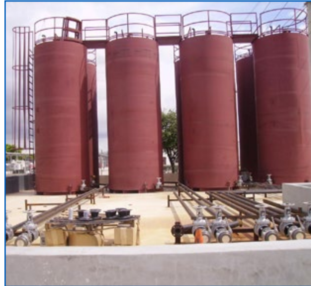
Check for Proper Secondary Containment Dimensions
