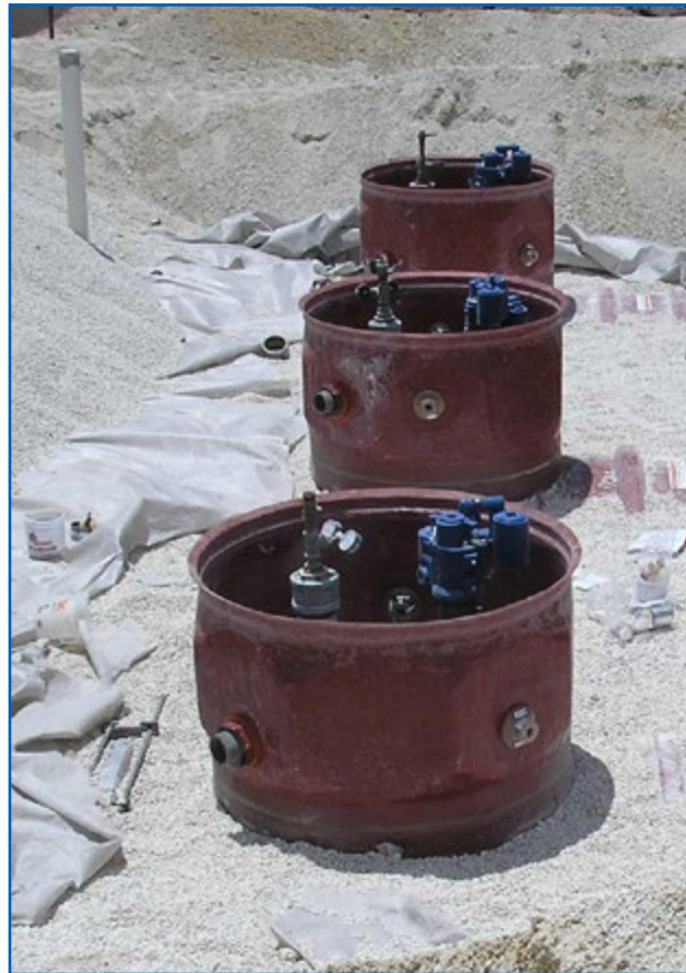
Pump Sump Installation
