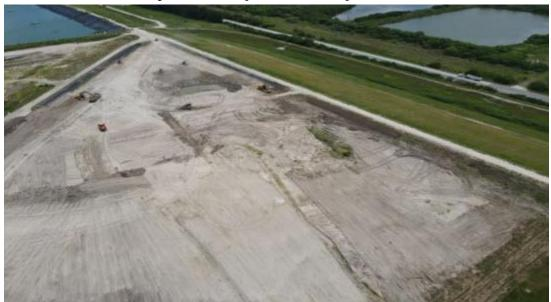
The court-appointed receiver and its contractor, Forgen, LLC, have begun closure work at the at the OGS-South compartment. Contractors are grading and shaping the area so that it will no longer accumulate rainwater and eliminate the need for future rainwater releases to Port Manatee.
