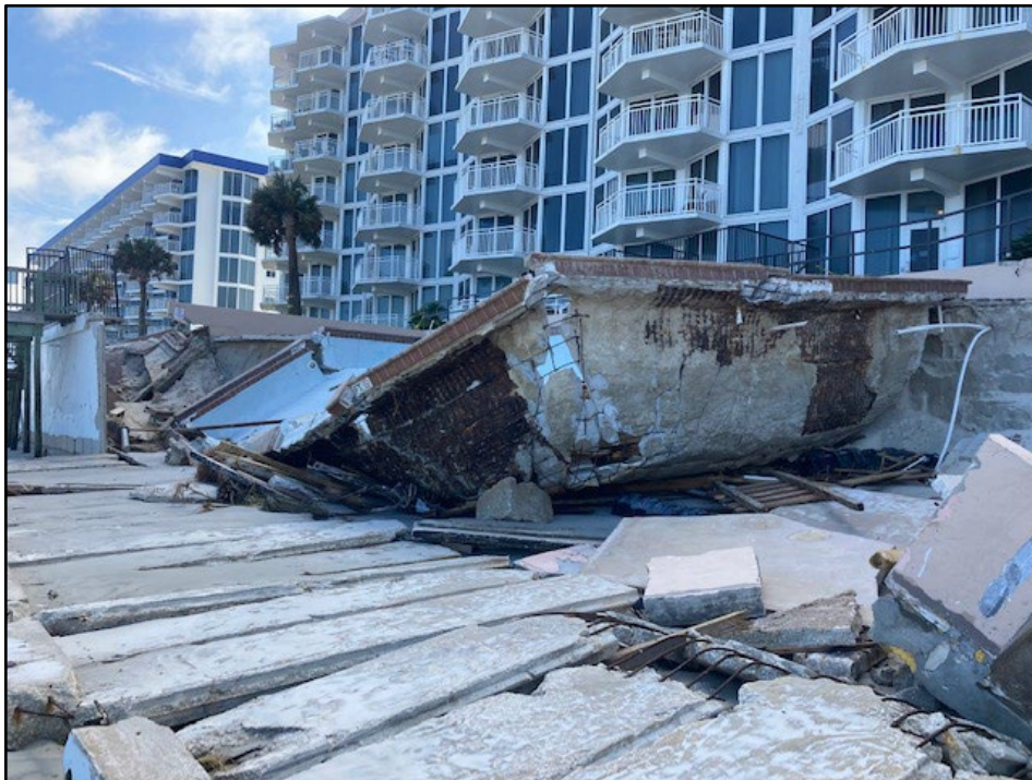
Figure 81. Seawall destroyed with inadequate pile penetration resulting in a destroyed
