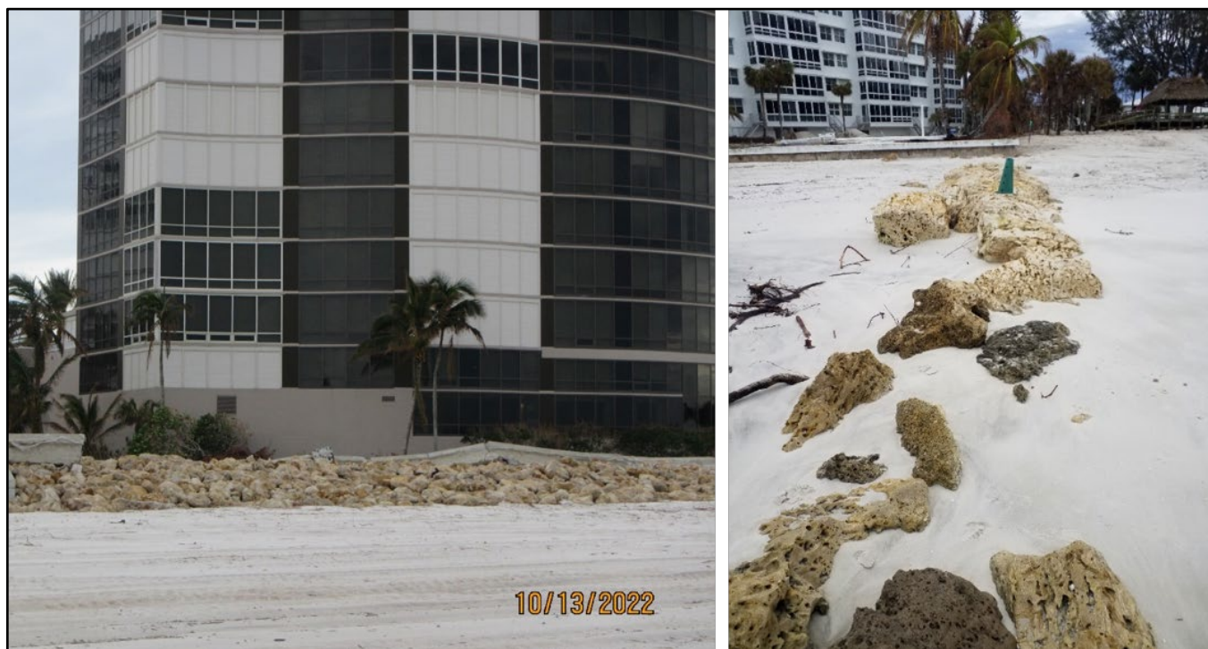
Figure 48. Concrete seawall collapsed in Naples at R-47 (left) and buried groin exposed at R-58 (right).
