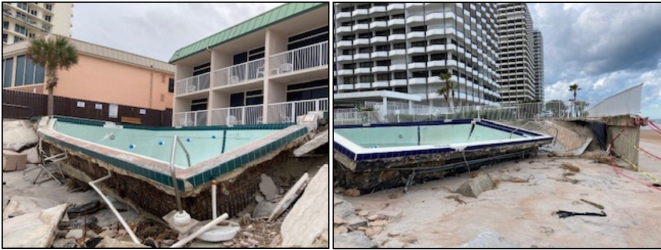
Figure 77. Swimming pools destroyed with seawall failure (R101).
