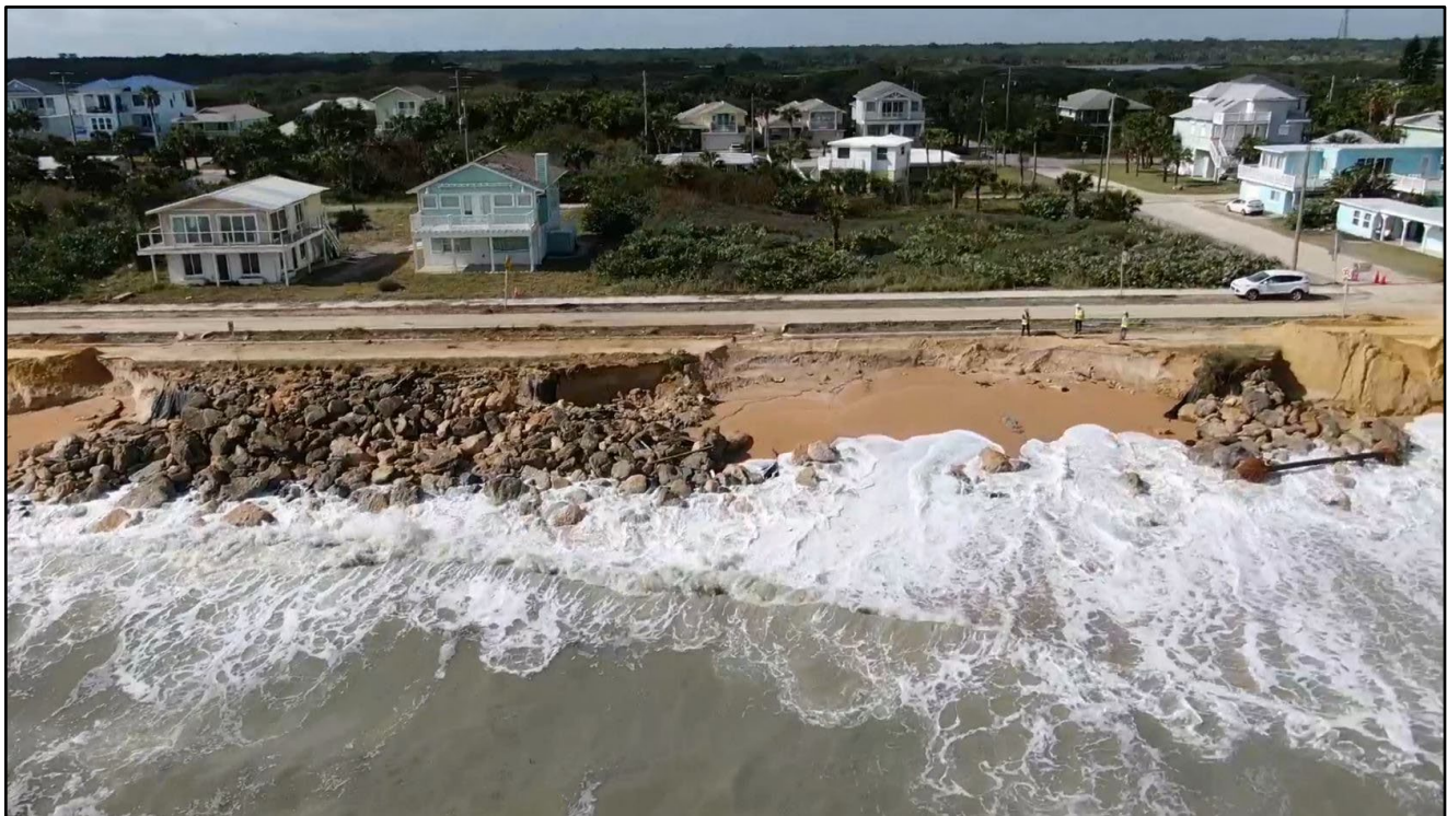
Figure 72. A1A revetment and road damage after Hurricane Nicole in Flagler Beach at 17 th Street South (R-88). Drone footage courtesy of Olsen Associates and Flagler County.
