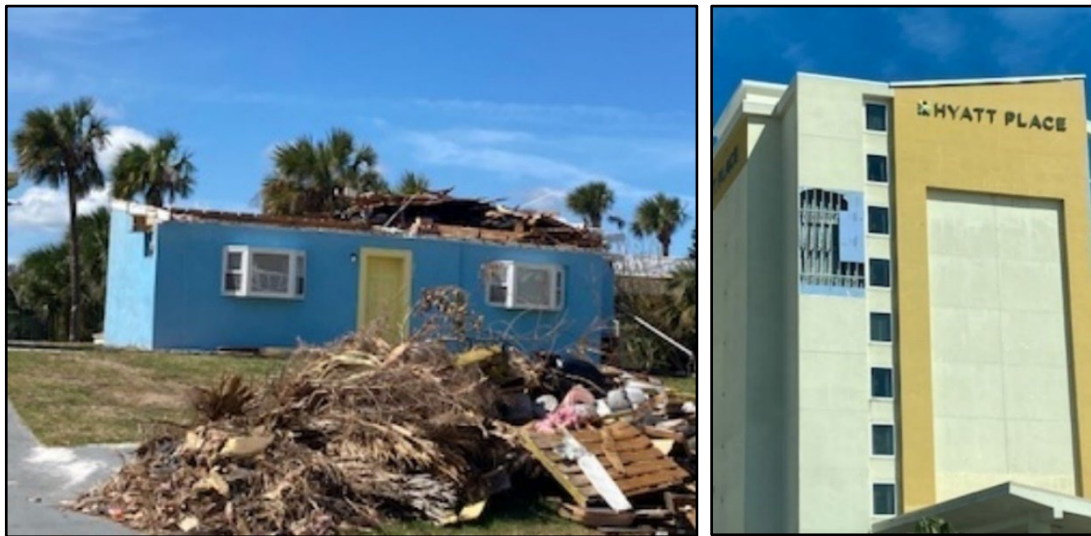
Figure 76. Roof blown off dwelling (left, R94); siding damage on hotel (right, R111).
