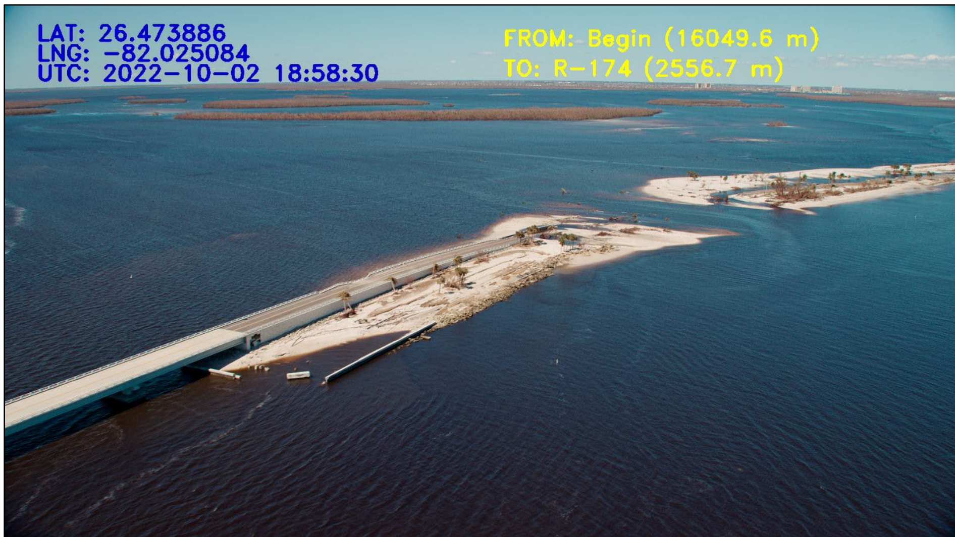
Figure 30. Sanibel Island bridge and causeway destroyed. (Image source: Active Camera Systems and Camera Copters).
