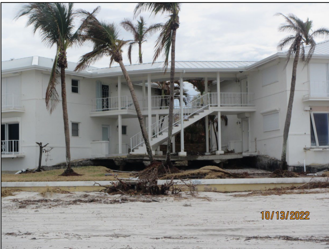
Figure 44. Understructure damage in Naples (R-60).
