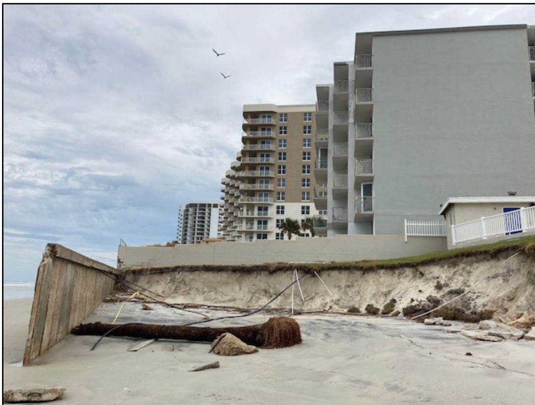
Figure 90. Substantial loss of property with seawall failure.
