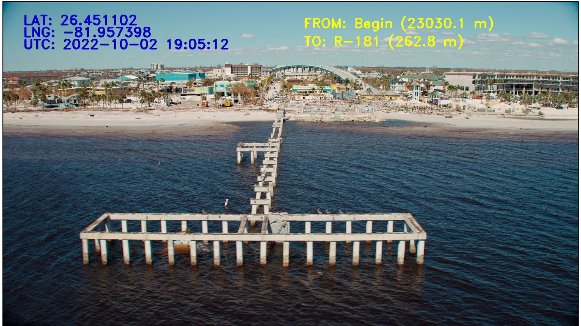
Figure 32. Ft. Myers Beach structures and pier with major damages, R-181 (Image source: Active Camera Systems and Camera Copters).
