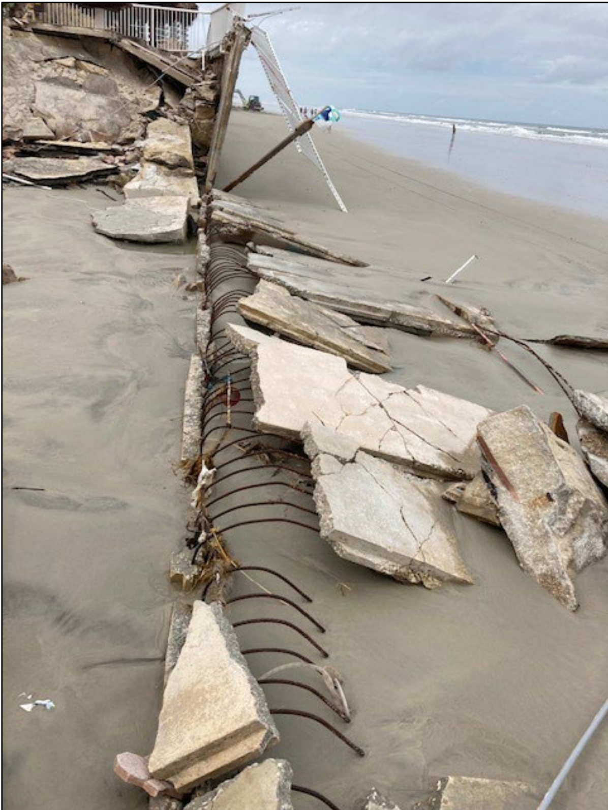
Figure 79. Seawall failure due to inadequate panel thickness of only 4 inches.
