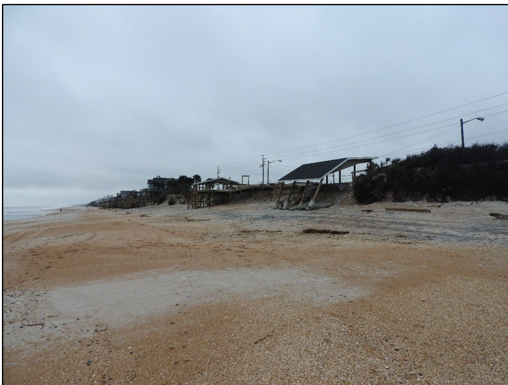
Figure 52. Major damage to a pavilion due to erosion in a county park in South Ponte Vedra (R-95).
