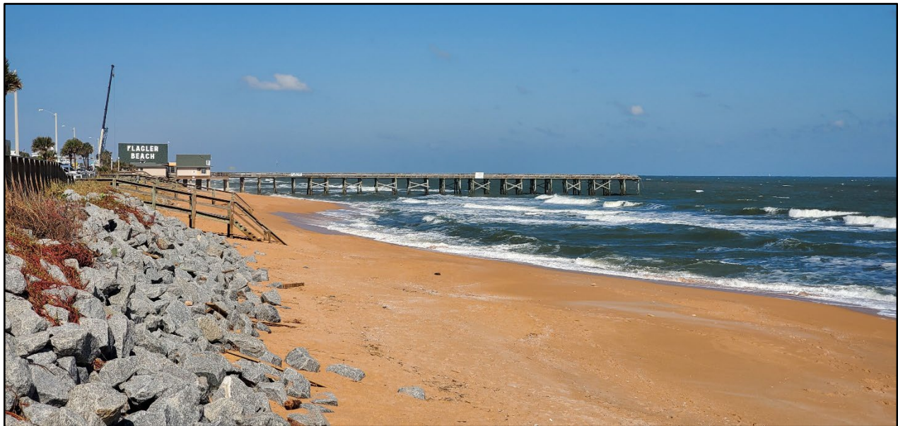
Figure 71. Flagler Beach Fishing Pier with 165 ft. of the seaward end destroyed (R-79).
