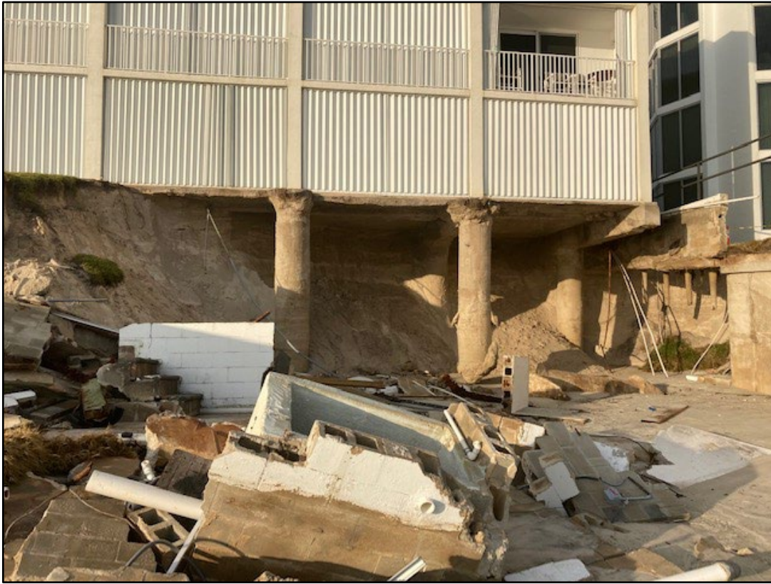
Figure 97. Threatened multifamily dwelling with foundation piles suspended (R117).
