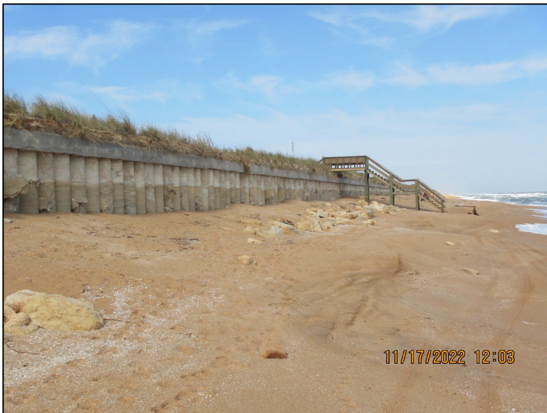
Figure 68. Major beach and dune erosion exposed the new secant wall constructed by the Florida Department of Transportation (R-66).
