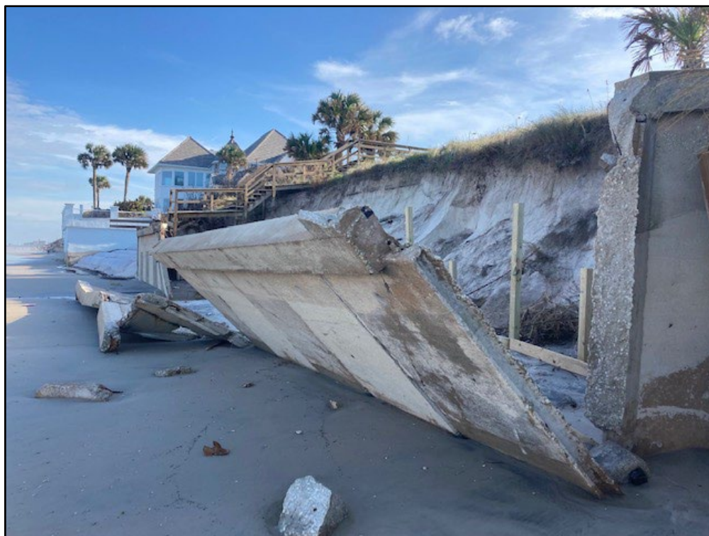
Figure 85. Seawall failure due to beach profile lowering and lack of tie-backs in Wilbur by the Sea (R124).
