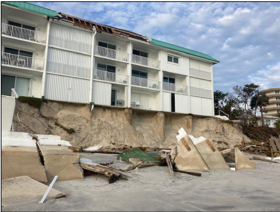
Figure 98. Condominium in imminent danger with roofing and siding damages.
