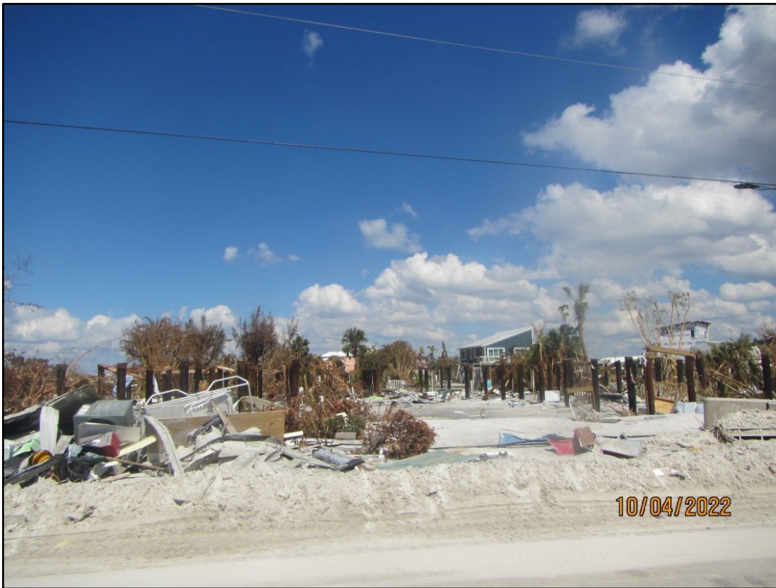
Figure 37. Homes destroyed and removed off pilings, Ft. Myers Beach near Matanzas St. (R-179).
