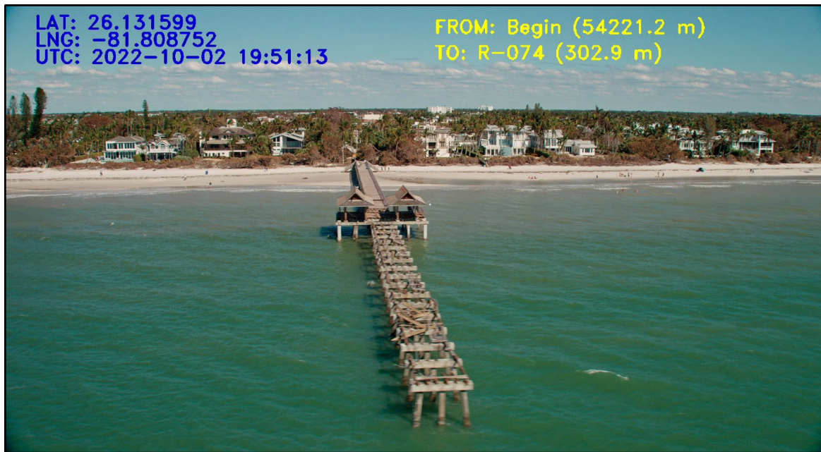
Figure 45. Damage to the Naples Pier (R-74).
