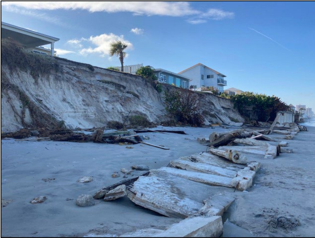
Figure 87. Catastrophic seawall collapse with loss of upland property in Wilbur by the Sea (R125).
