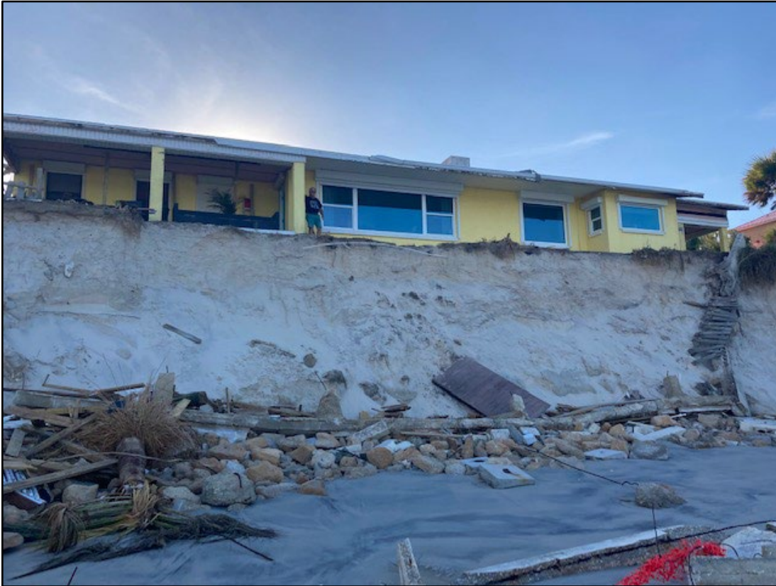
Figure 88. Wilbur-by-the-Sea dwelling threatened following seawall failure (R125).
