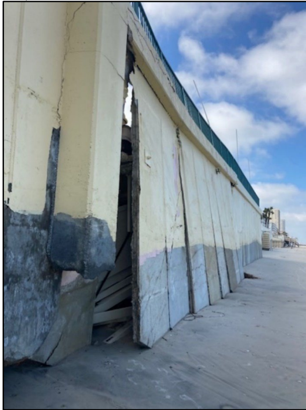
Figure 82. Inadequate sheet pile penetration.
