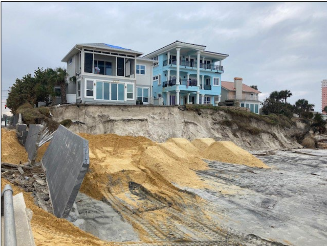
Figure 112. More threatened houses following severe erosion in Daytona Beach Shores (R-103).
