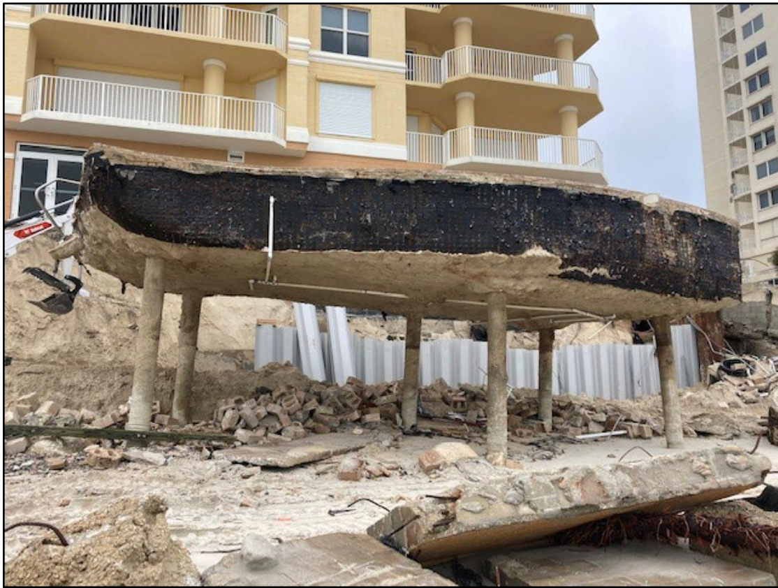
Figure 109. Undermined pile-supported pool in Volusia County.
