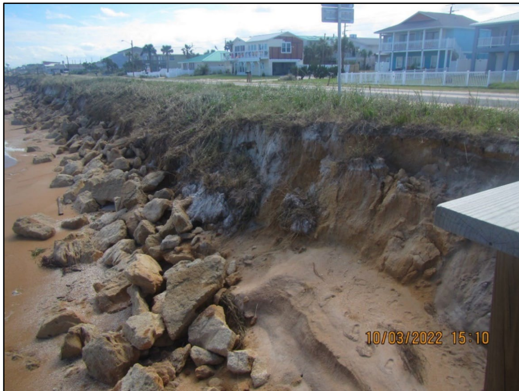
Figure 70. Major revetment damage due to Hurricane Ian south of the pier (R-80).
