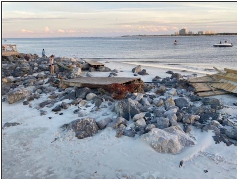
Figure 93. Damaged north jetty to Ponce de Leon Inlet (R-148).
