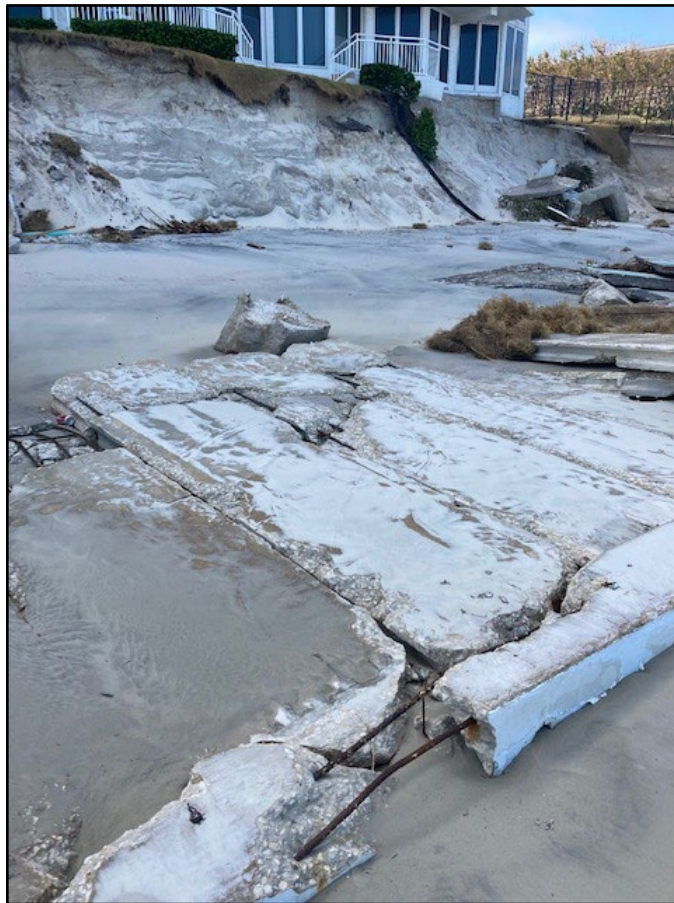
Figure 80. Old seawall with corroded reinforcing steel in Daytona Beach Shores (R116).
