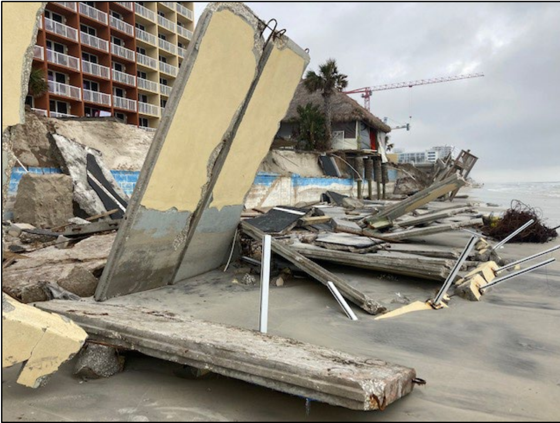
Figure 111. More seawall damage by Hurricane Nicole.
