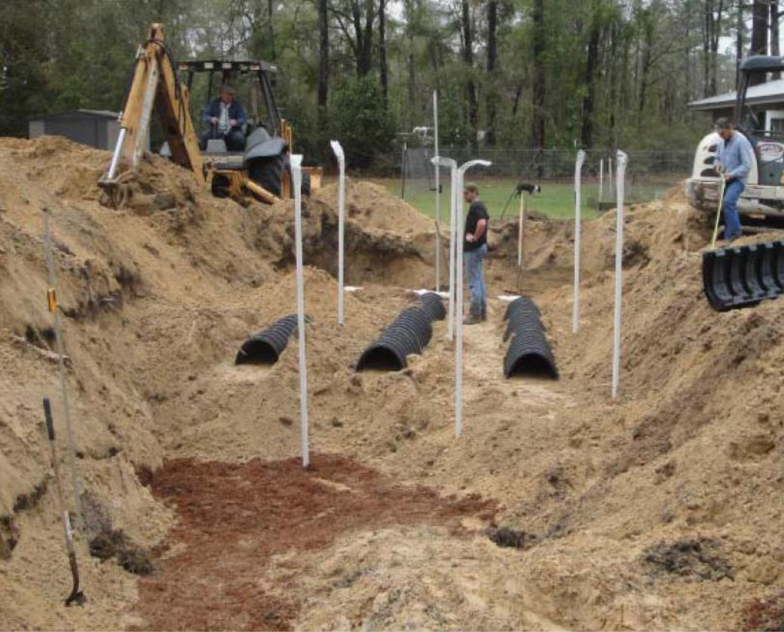
Figure 10. Installation of three rows of chambers at a slight angle to the length axis of the mulch bed. ~4:36 pm
