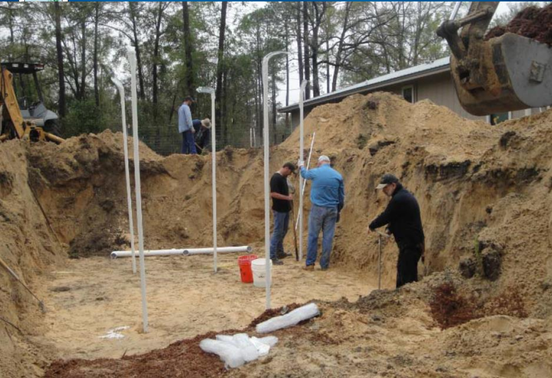
Figure 6. Installation of deep lysimeters (buckets contain silica mix). ~1:55 pm
