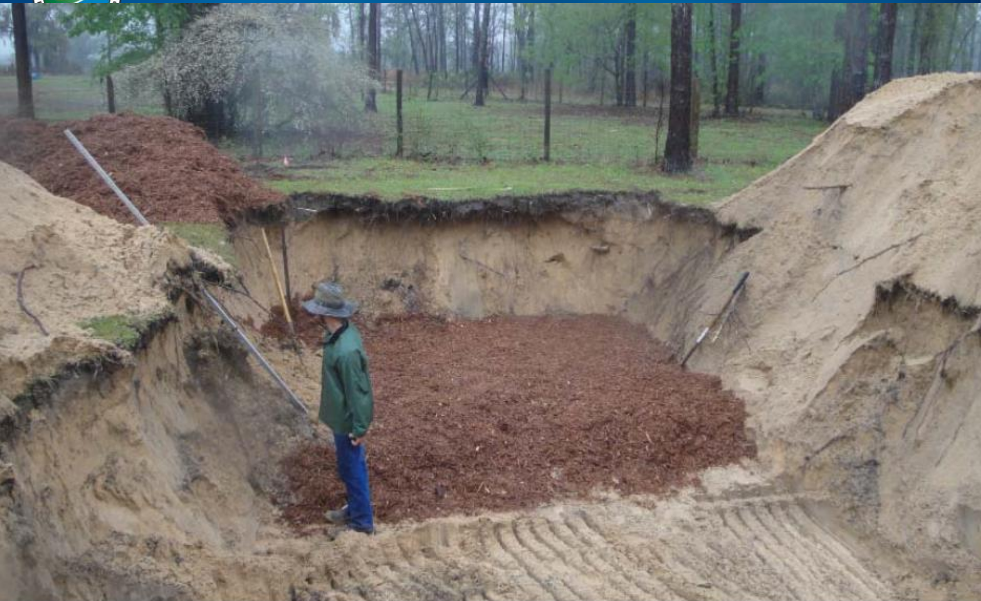
Figure 1. View East: First phase of lignocellulosic layer installation. ~11:20 am
