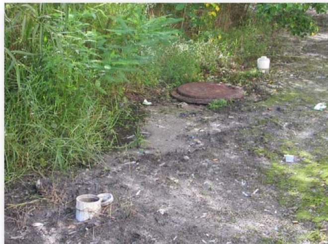
Clean out caps missing from sanitary sewer laterals
