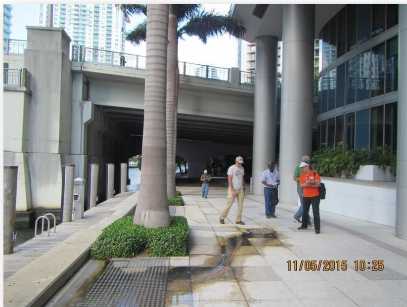
Sidewalk stained by sewage discharge from stormwater system
