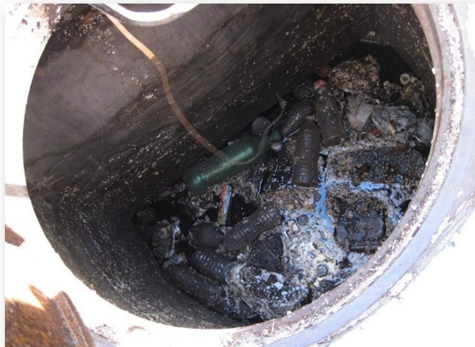
Stormwater system in need of clean out and maintenance
