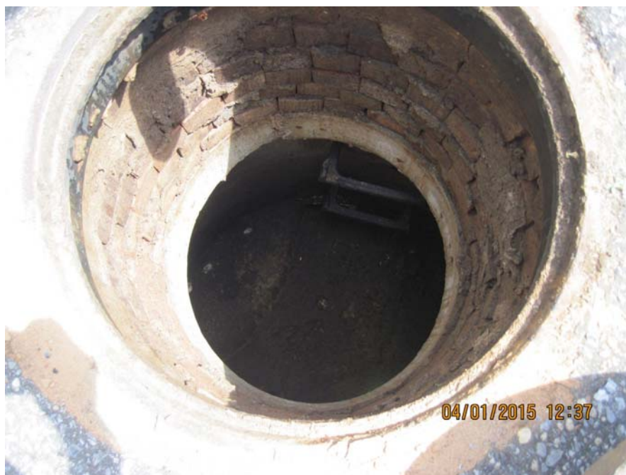
Degrading sanitary sewer manhole
