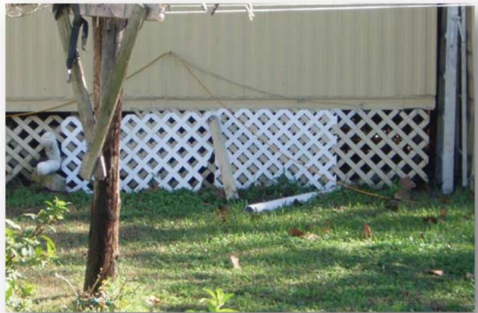
Illicit discharge pipes
