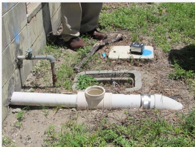
Clean out caps missing from sanitary sewer laterals
