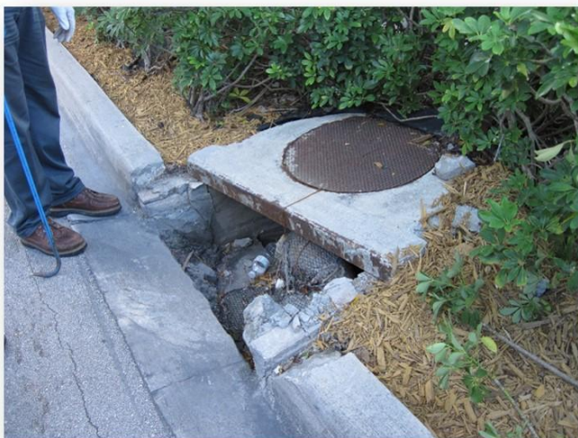
Stormwater system in need of clean out and maintenance
