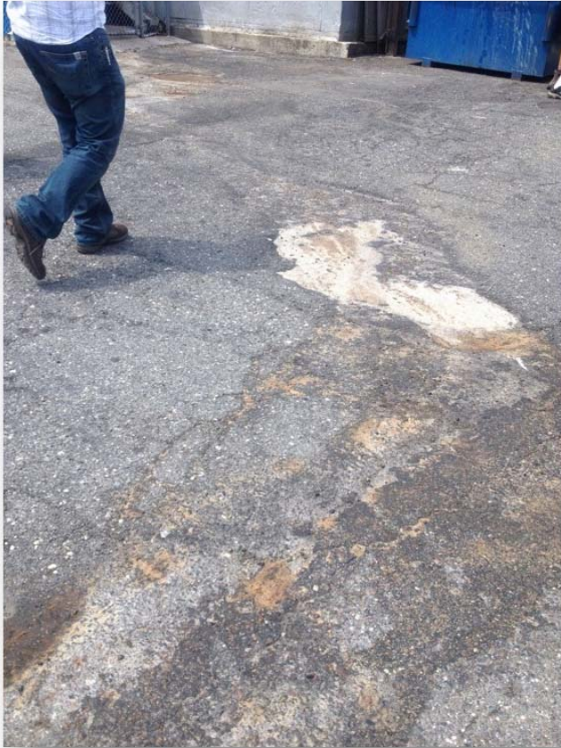
Greasy sludge on asphalt and grease trap cover
