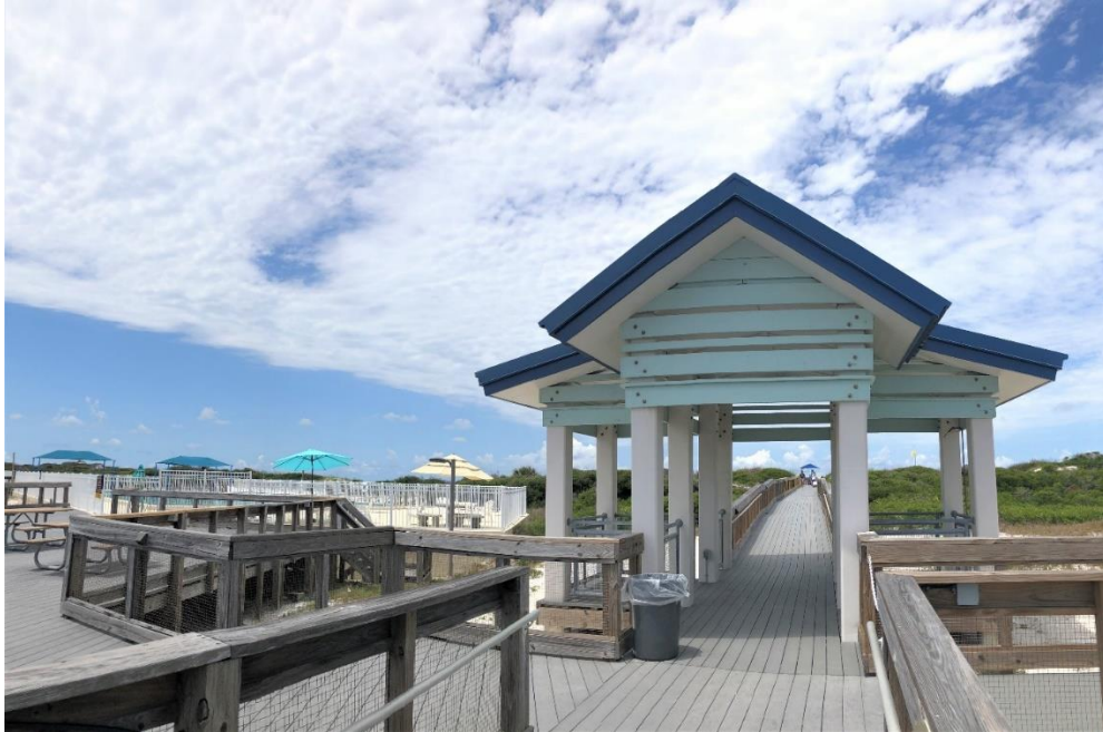
View of pool area connected to the main boardwalk, a potential location for a restroom and concessionaire operating area.
