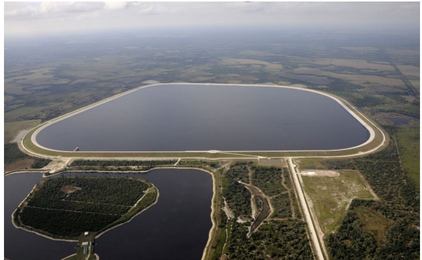
Surface Water Storage
