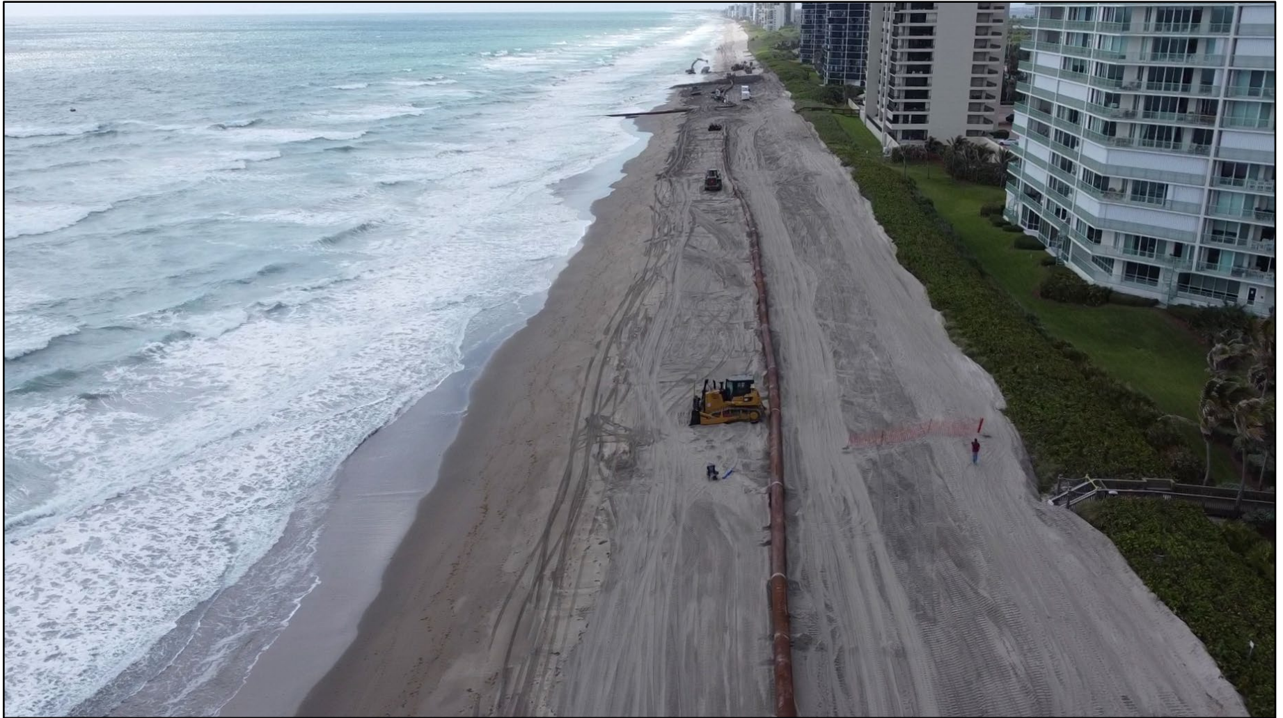
The federal (USACE) St. Lucie County Coastal Storm Risk Management Project being constructed near R-99, in April 2022. Photo courtesy of Joshua Revord P.E., with St. Lucie County. See additional construction photos of beach nourishment projects.
