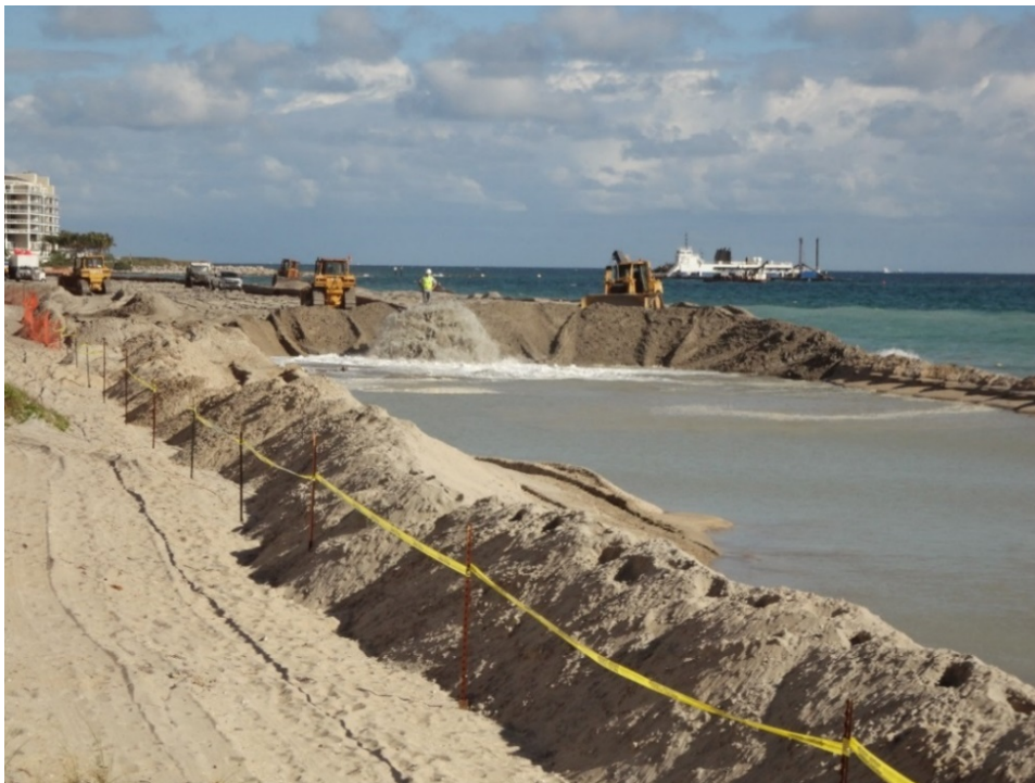
Figure 8. South Boca Raton beach nourishment project (2013) using sand from offshore sources. Photo courtesy of Peter Seidle, P.E..
