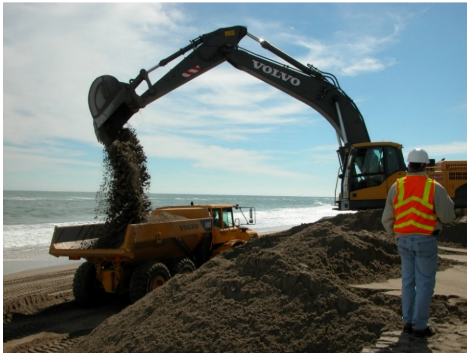
Figure 7. Wabasso Beach (Indian River County) nourishment project (Sector 3) using sand from upland sources. DEP project file photo.
