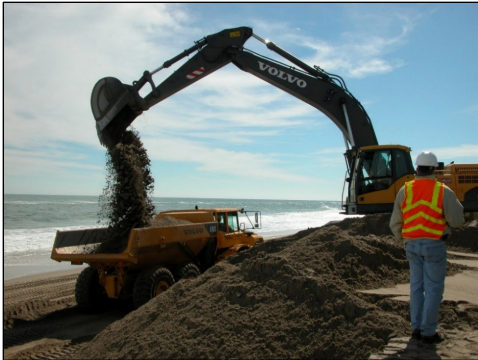
Figure 7. Wabasso Beach (Indian River County) nourishment project (Sector 3) using sand from upland sources. DEP project file photo (2010).
