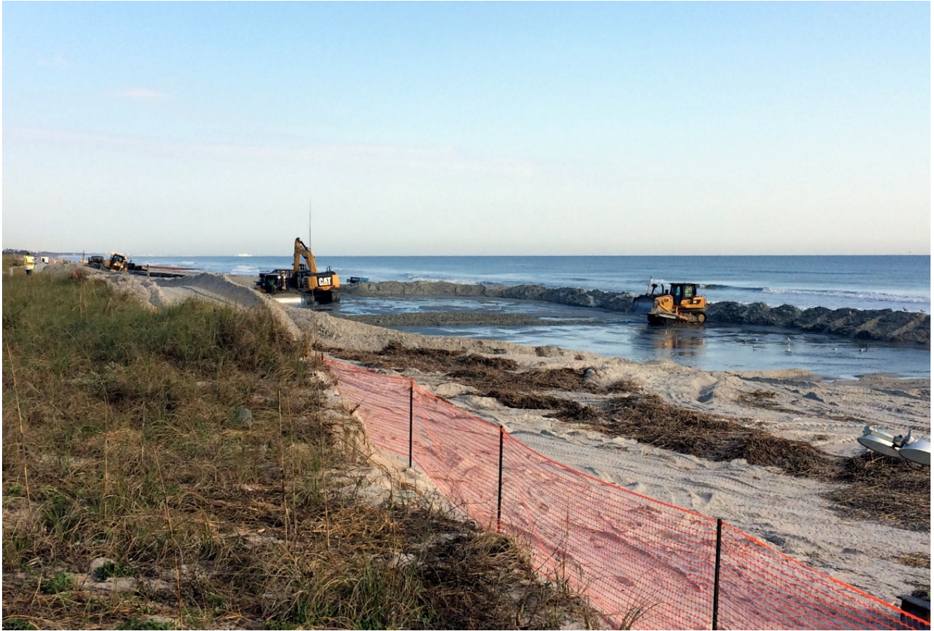
Duval County Shore Protection Project under construction in November 2016. Photo courtesy of Kevin Bodge, P.E.
