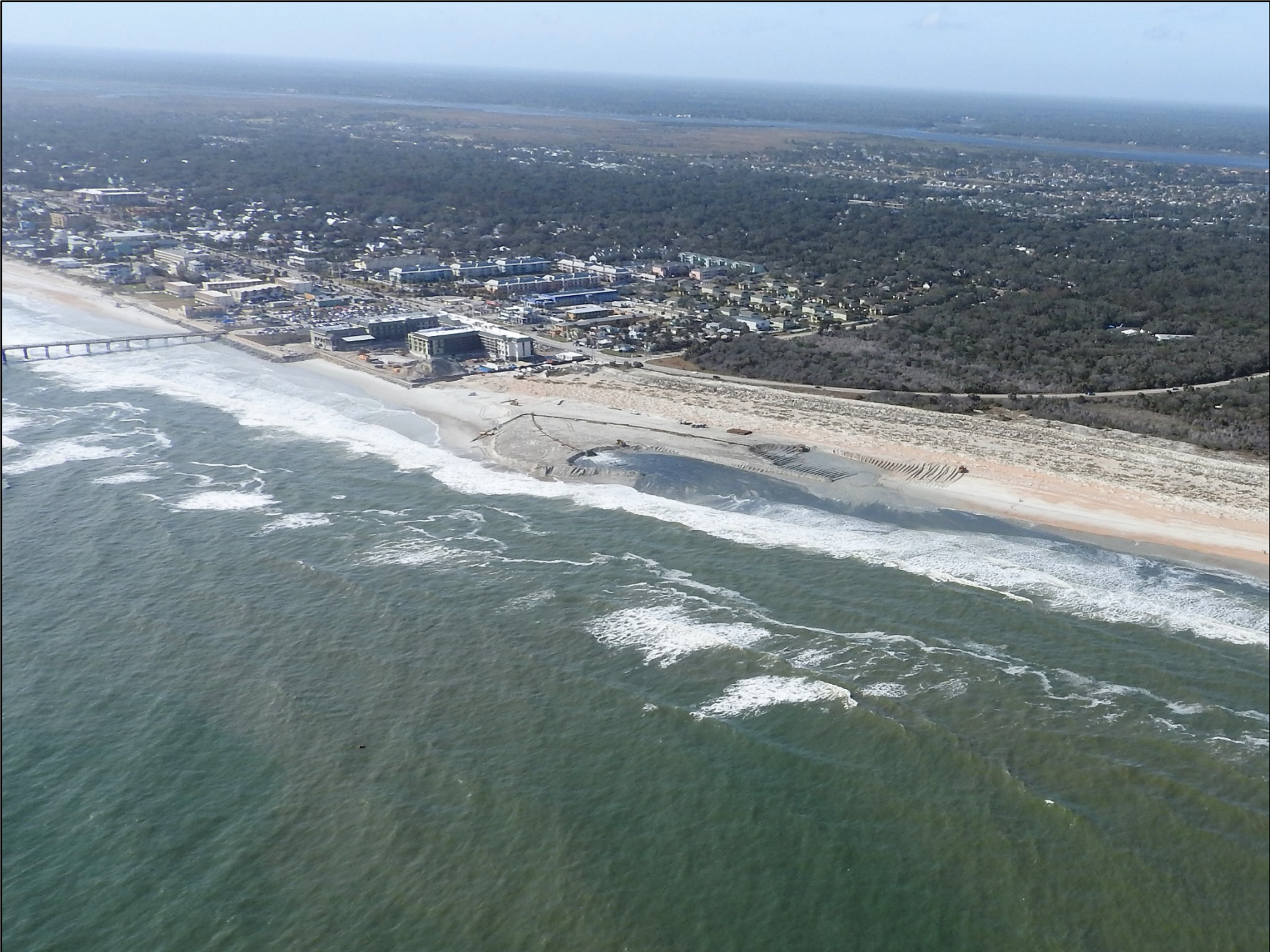
St. Augustine Shore Protection Project at early stages of construction near R141 in February 2018, photo by W.G. Weeks.
