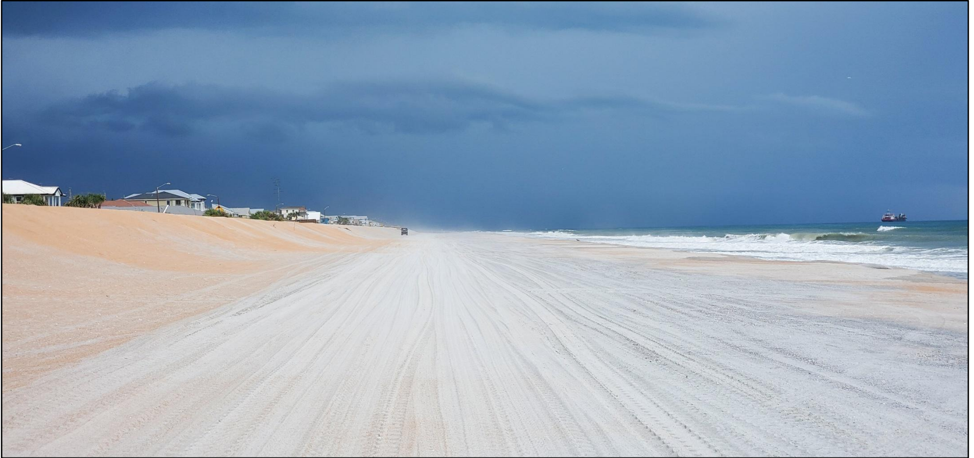
Project Photo 2. The federal Flagler County Hurricane and Storm Damage Reduction Project (Reach I) during construction by the USACE, near R91 or S. 25 th St. in August 2024. Photo was taken before the salt tolerant dune plants were planted by contractor. Photo taken by DEP staff, Guy Weeks. See additional construction photos of beach nourishment projects.
