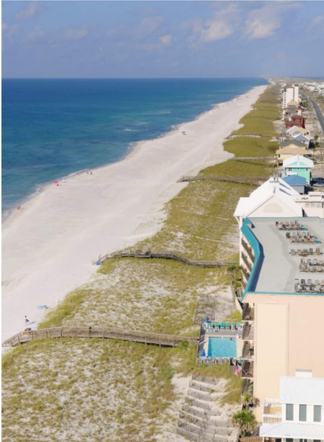
Completed Navarre Beach Nourishment Project in September 2016. Photo courtesy of Michael Walther, P.E.
