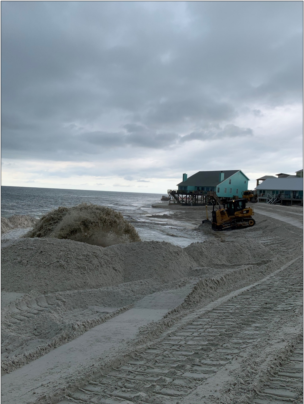
St. Joseph Peninsula Beach Nourishment Project under construction in October 2019. FDEP photo taken by Greg Garis.
