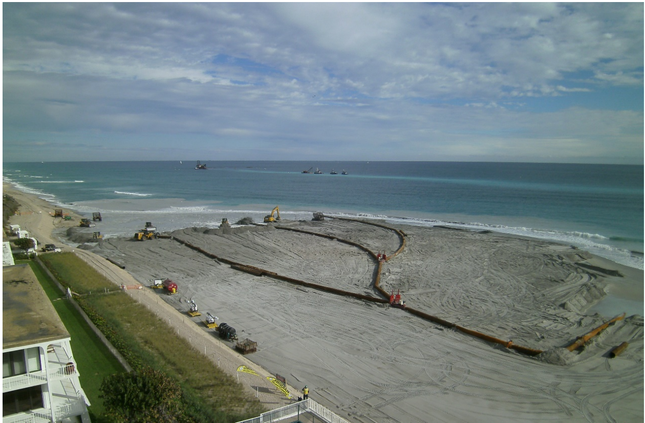
Phipps Ocean Park Beach Nourishment Project being constructed in January 2016. Photo courtesy of the Town of Palm Beach.
