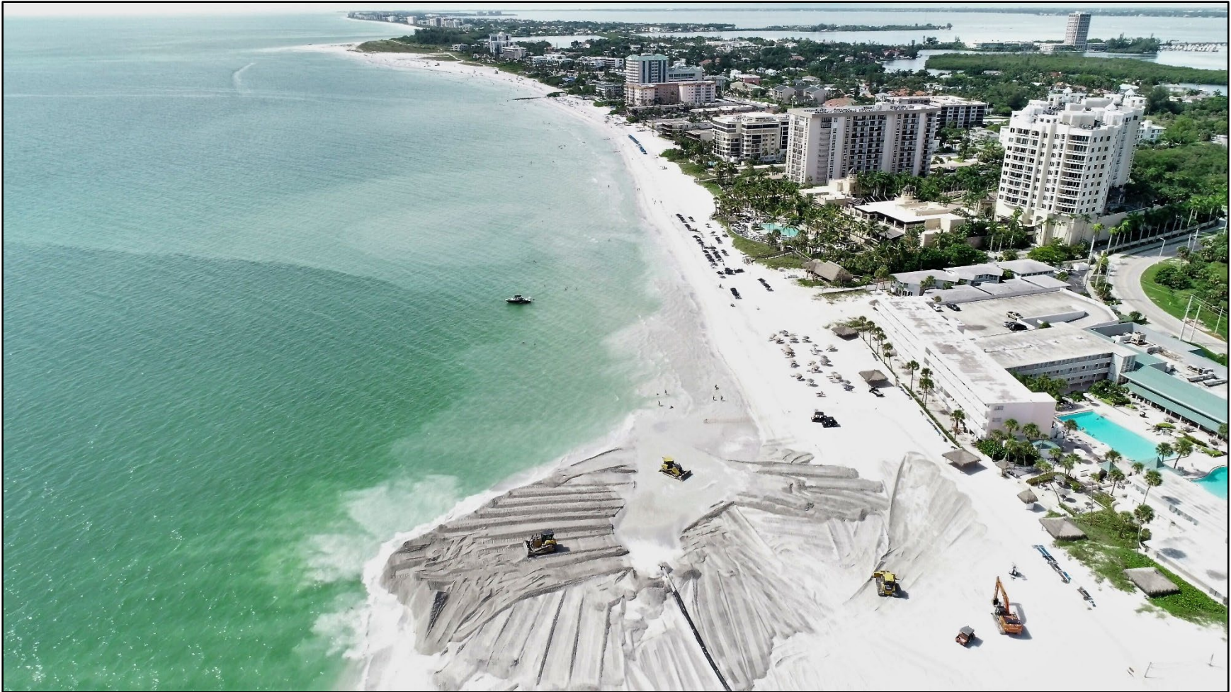
Lido Key Shore Protection Project being constructed in 2020 near R41. Photo courtesy of Camden Mill, P.E., with the City of Sarasota. See additional construction photos of beach nourishment projects.
